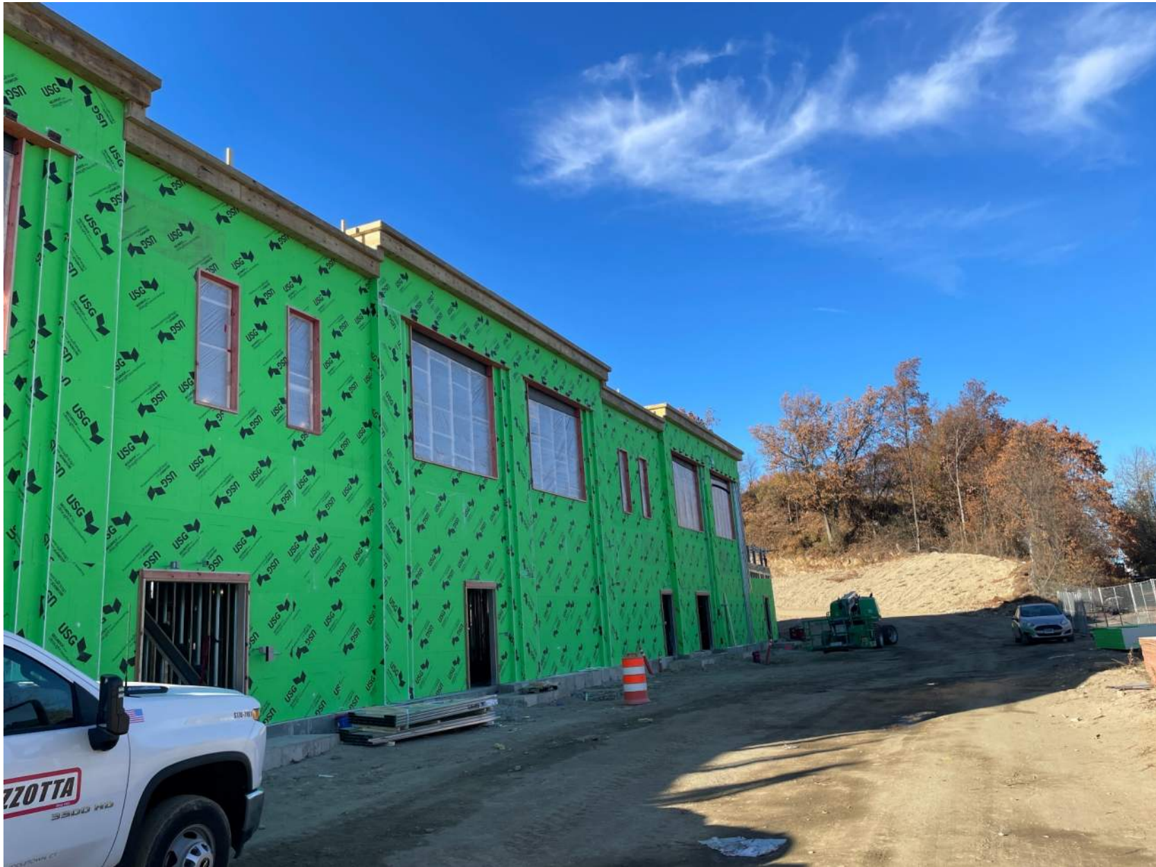
East Elevation – CFMF & Exterior Sheathing Complete 11/15/24
