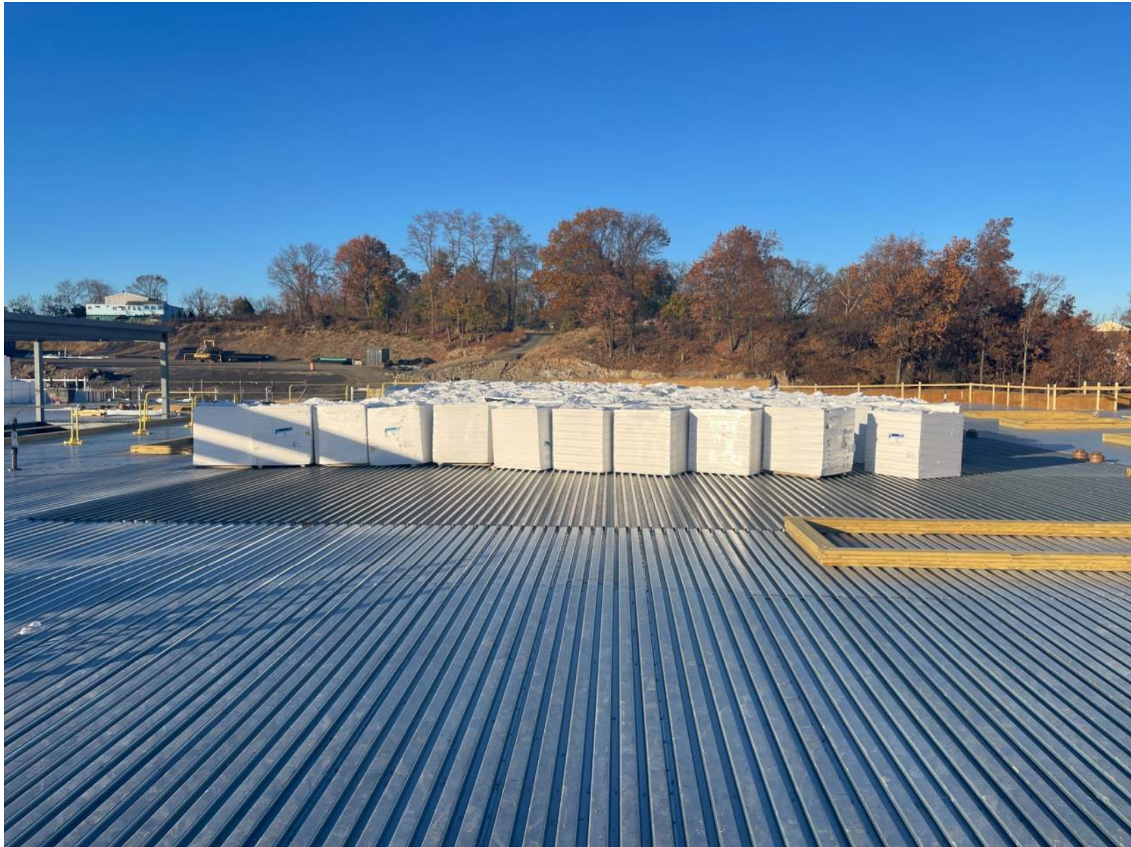
Rough decking, Equipment/Skylight Curbs, Roof Insulation 11/13/24
