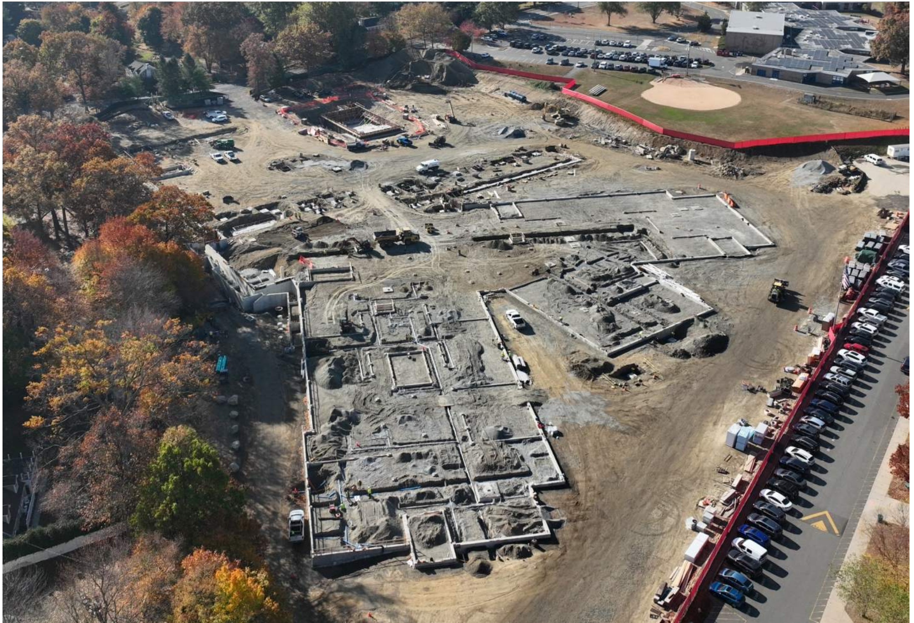
Drone Image – Foundations, Underslab Utilities, Pool Concrete 10/31/24
