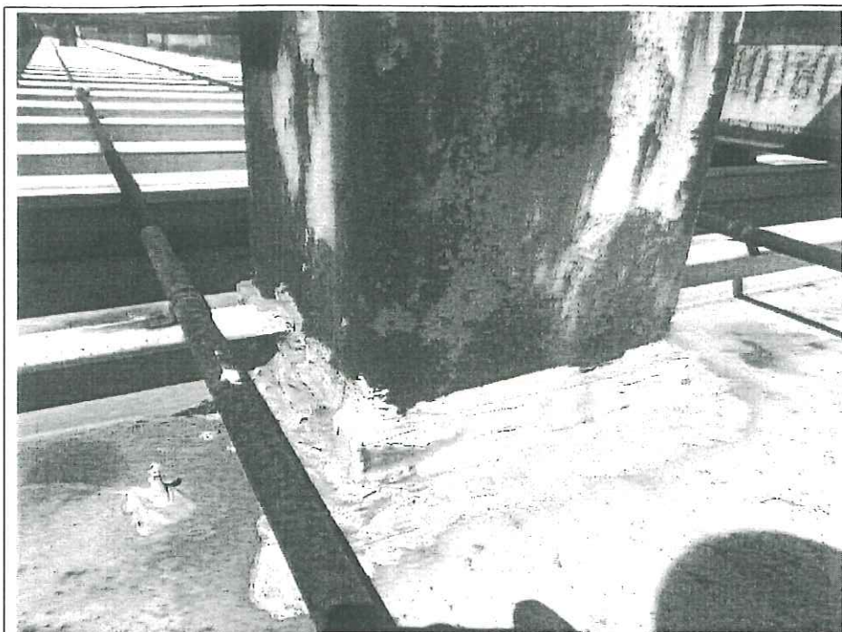
Photo 11: Canopy panels cut and sealed around support columns.
