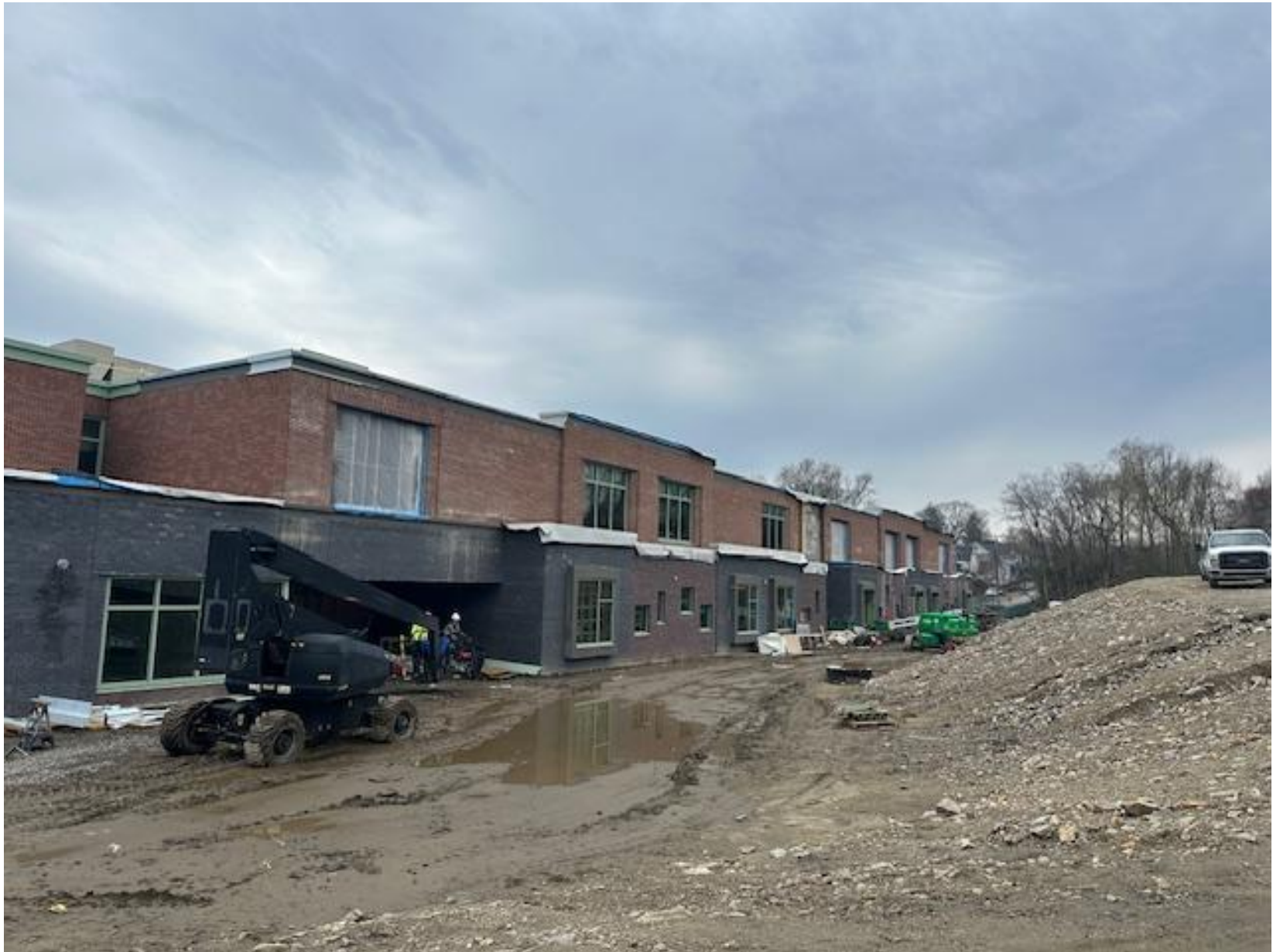
Rear of Building on North Side 4/15/25
