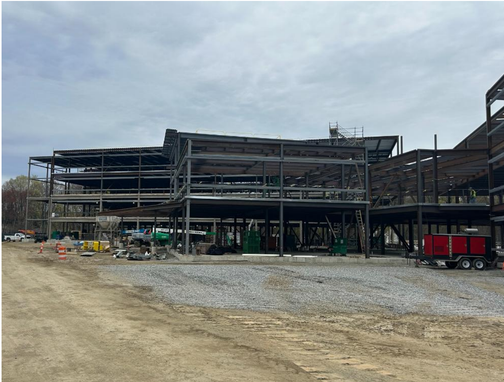
Steel Erection & Metal Deck – NHS and Main Entrance 4/21/25
