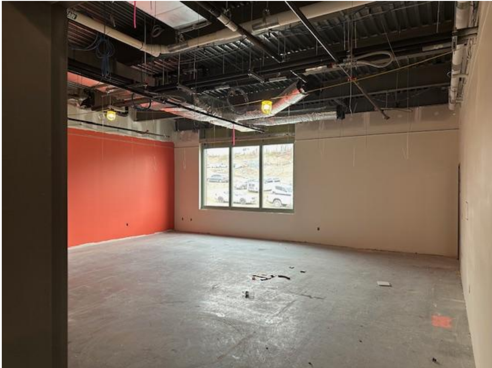
Classroom Paint & Ceiling Grid Wire Installed 4/15/25
