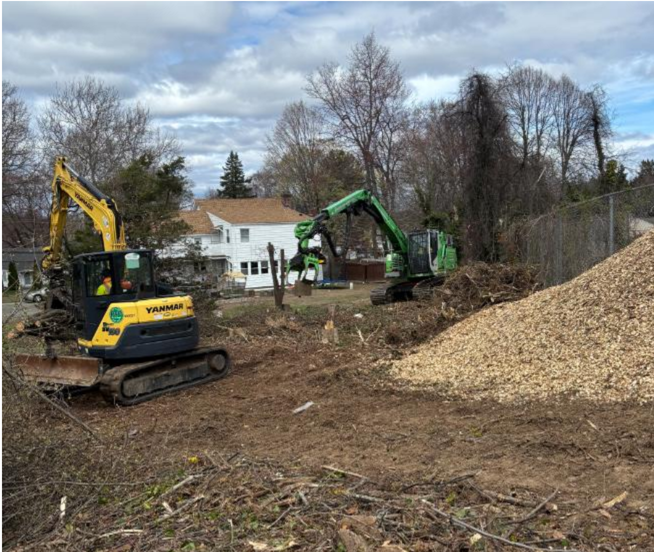
Additional Site Clearing for Multi-Use Field 4/16/25
