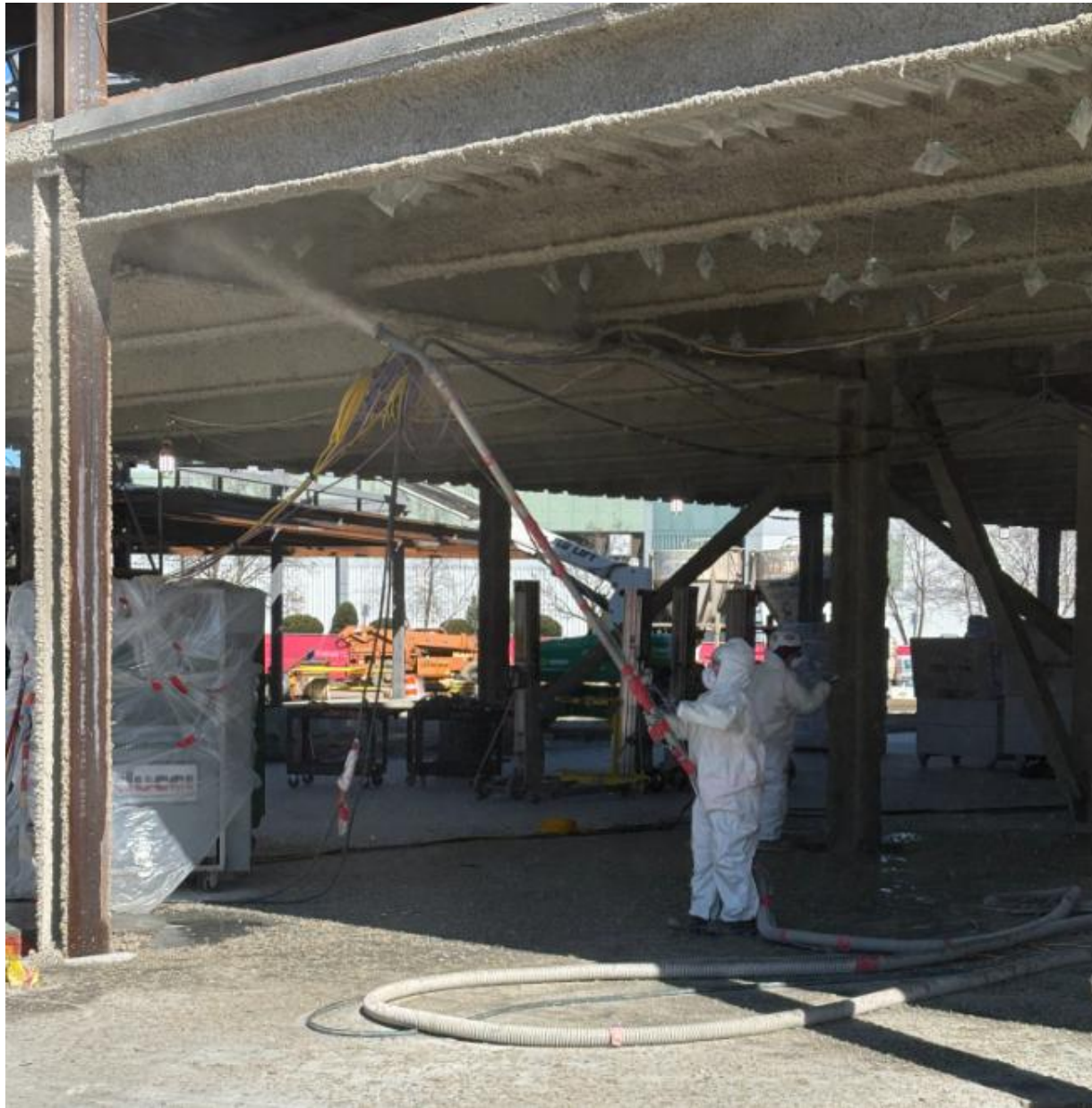
Spray on Fireproofing 4/21/25
