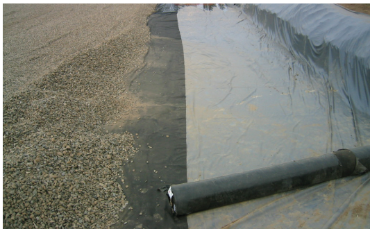
Non-woven fabric is placed over PVC liner before placing angular bedding stone.
