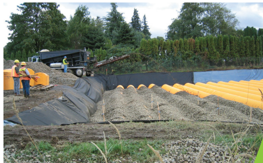
Angular stone backfill is placed around chambers.
