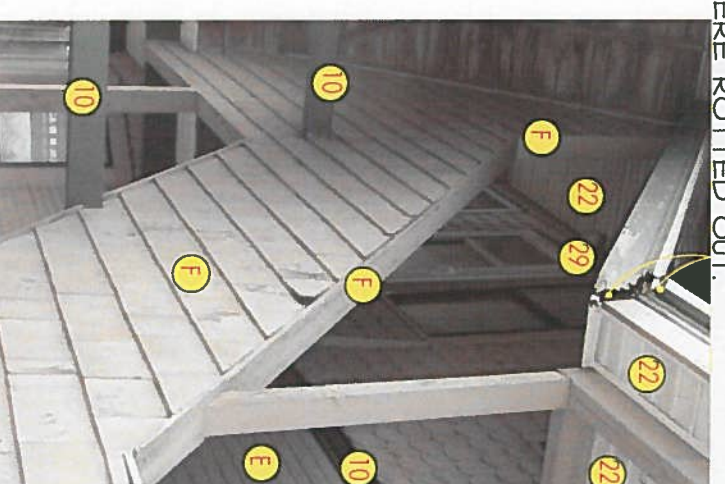
BACK FIRE STAIR TO 2ND. FL. LOOKING TOWARDS STREET
