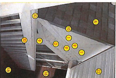
FRONT STAIR DOWN FROM ATTIC FL.
