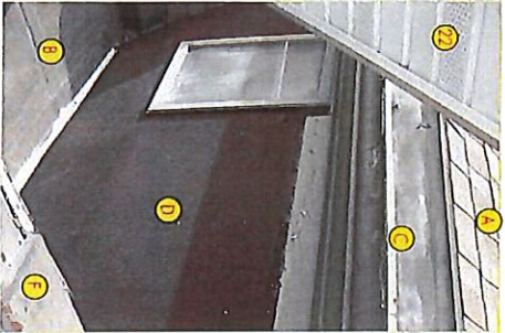
WALL, GUTTER, ROOF & STAIR CLG. @ BACK ATTIC FL.
