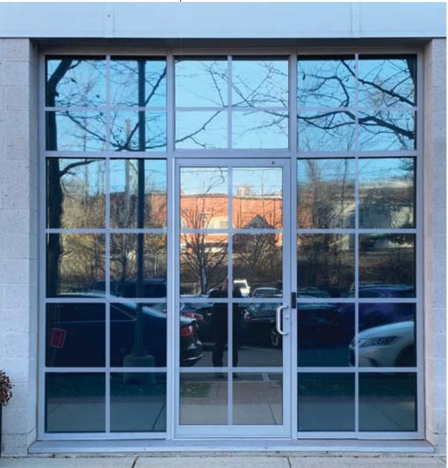
NEW APARTMENT TERRACE DOORS
