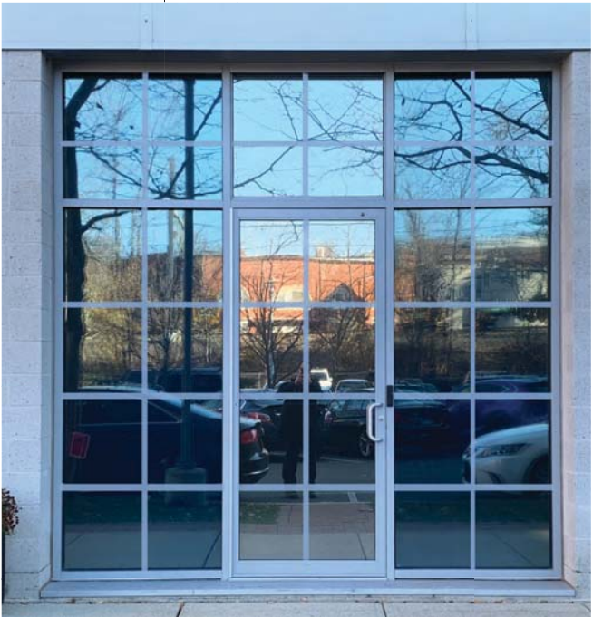
NEW APARTMENT TERRACE DOORS
