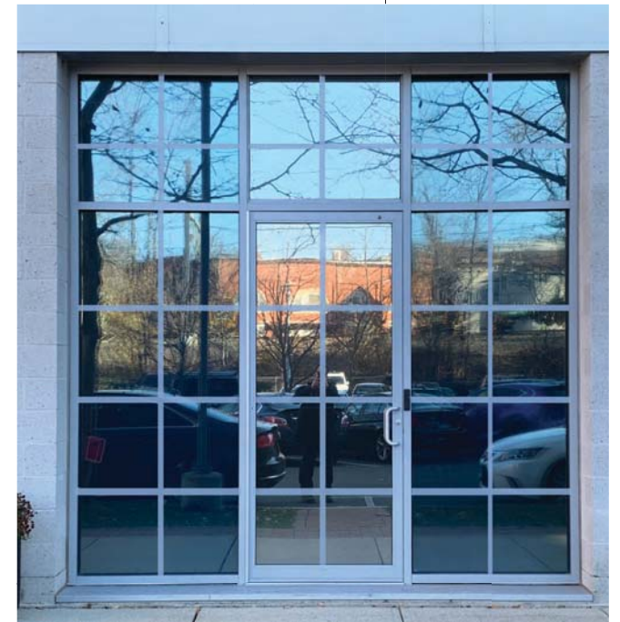
NEW APARTMENT TERRACE DOORS
