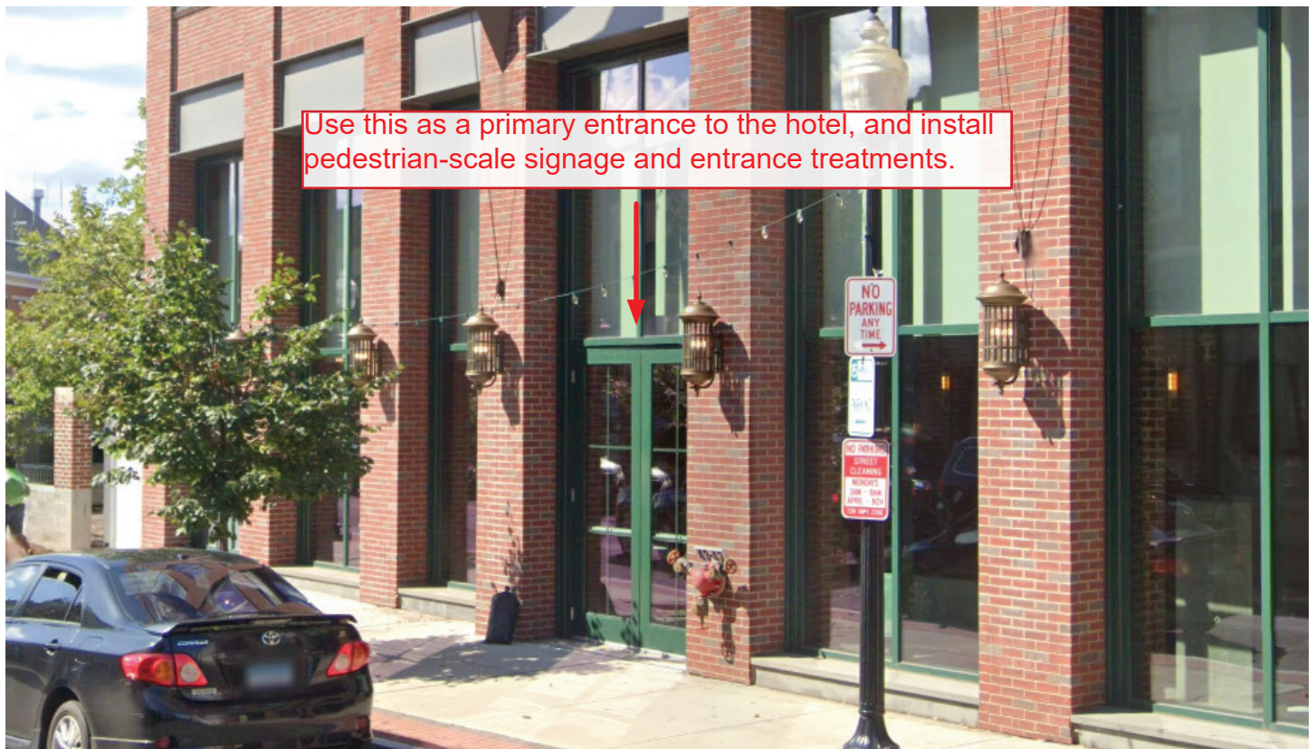
Photo 4: View of unused street entrance to Marriott hotel.
