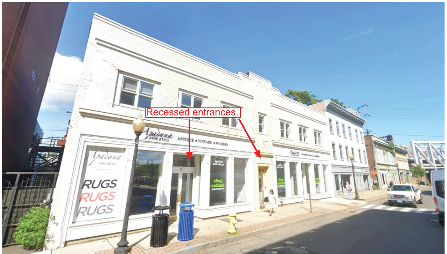
Photo 2: View of existing building at 31-35 South Main Street looking northwest.
