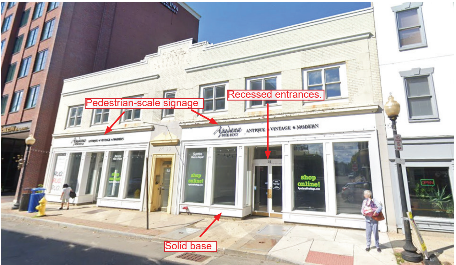
Photo 1: View of existing building at 31-35 South Main Street looking southwest.
