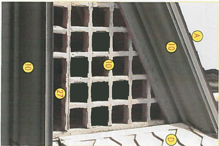
PORCH UPPER LATTICE
