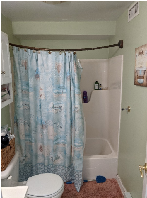
Image 4 – Second Floor Bathroom
