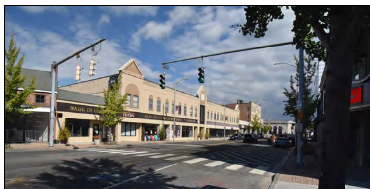
84 Wall Street with 68 Wall in the distance
