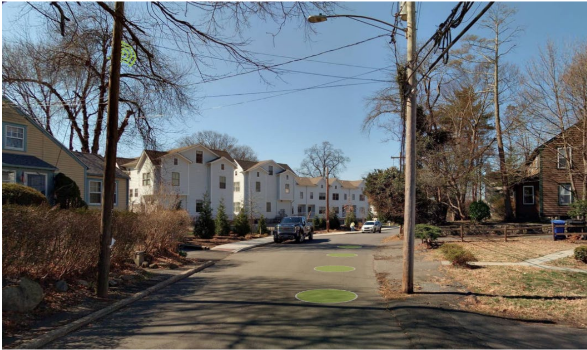
Howard Ave facing west around the roadway curve
