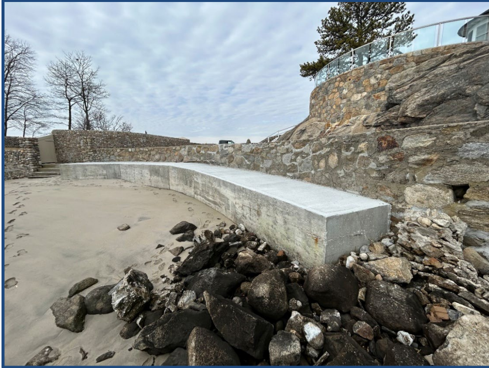
Figure 3: Repaired Lower Seawall, Facing Southwest (3/4/2025)
