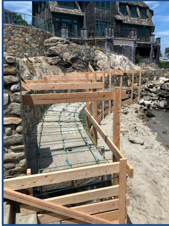
Figure 9: Installation Of Formwork in Preparation for Concrete Pour, Facing North (7/10/2025)
