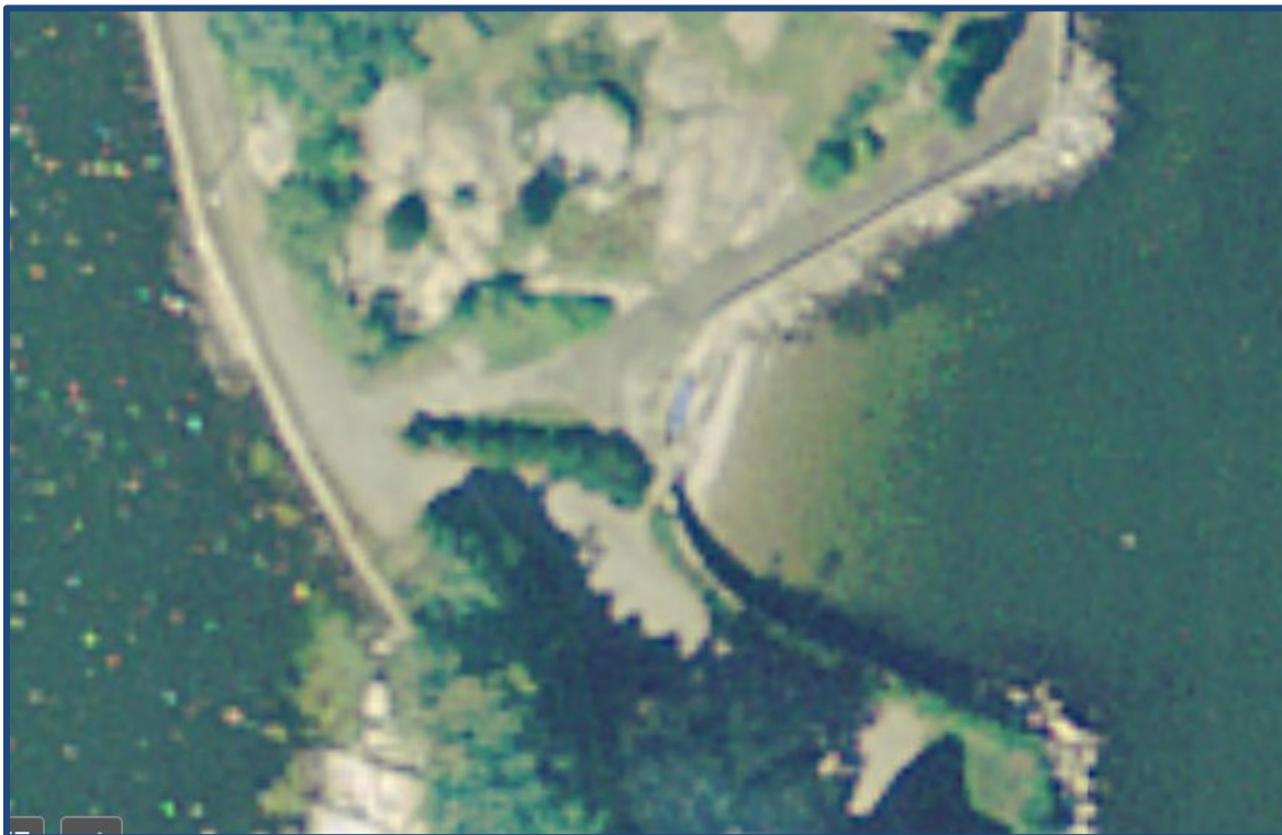
Figure 7: 2004 Aerial Showing Lower Seawall
