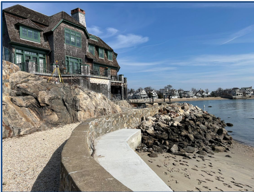
Figure 4: Residence, Upper and Lower Seawall, And Stone Revetment, Facing Northeast (3/4/2025)
