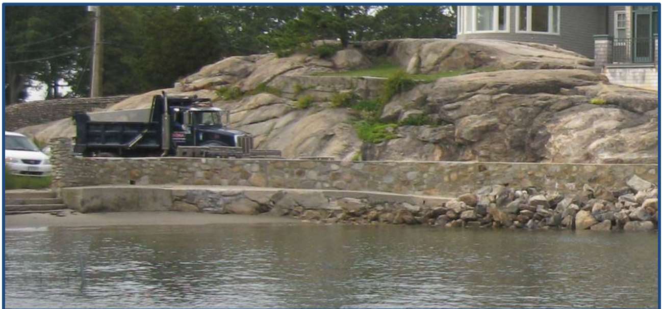
Figure 10: Photograph of Lower Seawall in Serviceable Condition (10/09/2008)
