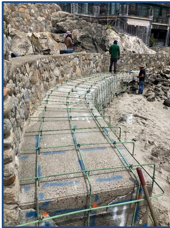
Figure 8: Steel Reinforcement Installed on Existing Wall, Facing North (7/9/2025)
