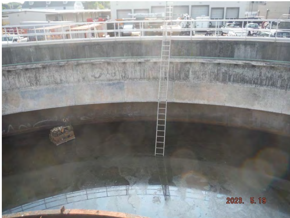
Tank #4 – General view of the inside face of segment 4-5, looking south. Note 40' ladder installed.
