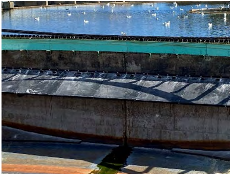
Figure 7. Stamford Baffle
