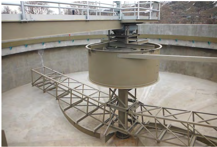
Figure 5. Spiral Scraper Type Mechanism from Envirodyne Systems Inc.
