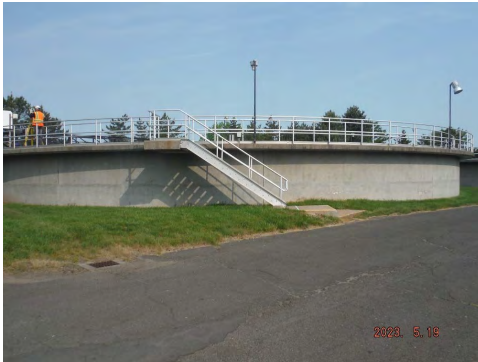
Tank #3 - General View, looking north.
