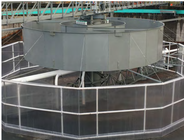
Figure 8. Cylindrical Baffles
