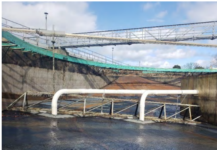
Figure 4. Conventional Scraper with Draft Tubes
