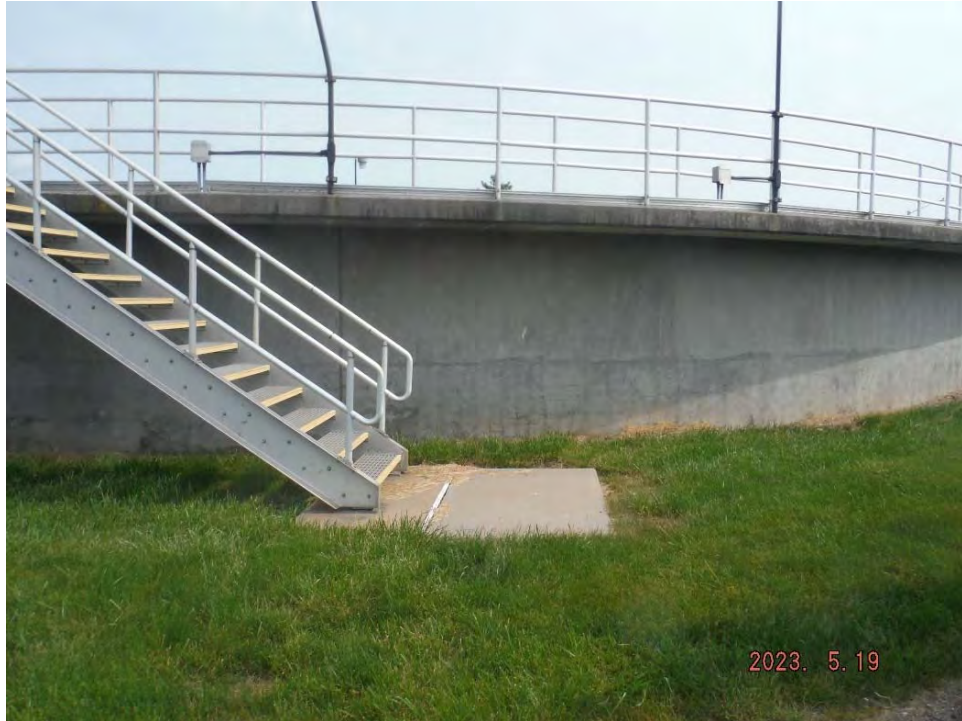
Tank #1 - General View, looking north.
