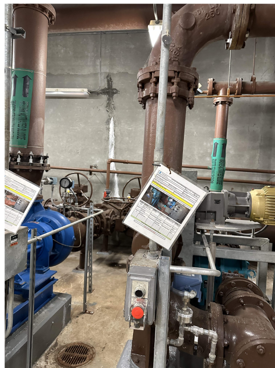
#6 -Efflorescence on Wall
