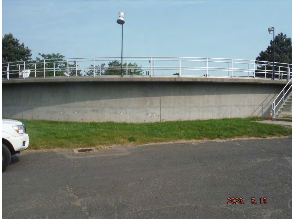
Tank #2 - General View, looking north.
