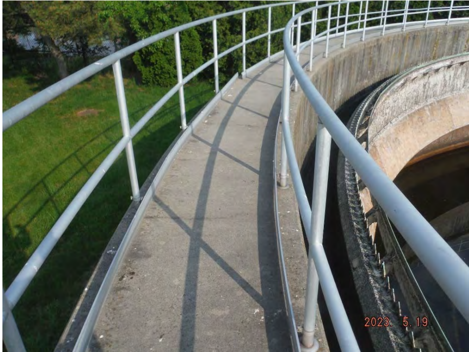
Tank #4 – General view of the top of catwalk at Segment 4-5, looking north.
