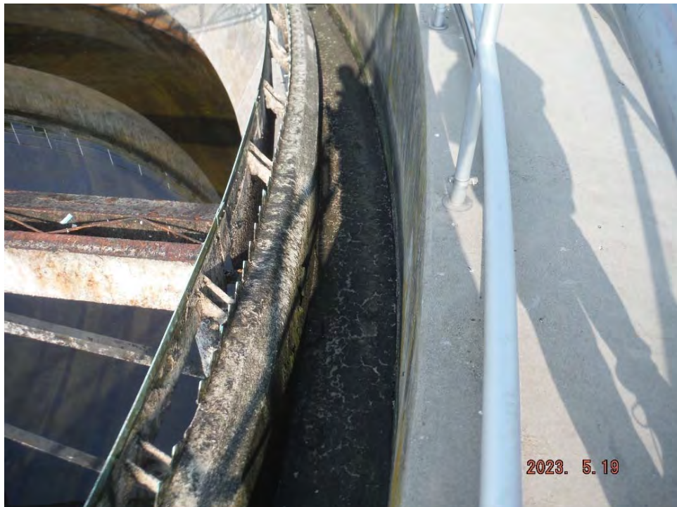
Tank #4 – General view of the inside face of segment 4-3, looking north.
