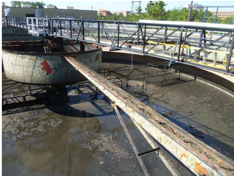
Figure 2. Existing FST Mechanism
