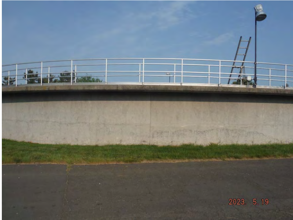
Tank #4 - General View, looking north.
