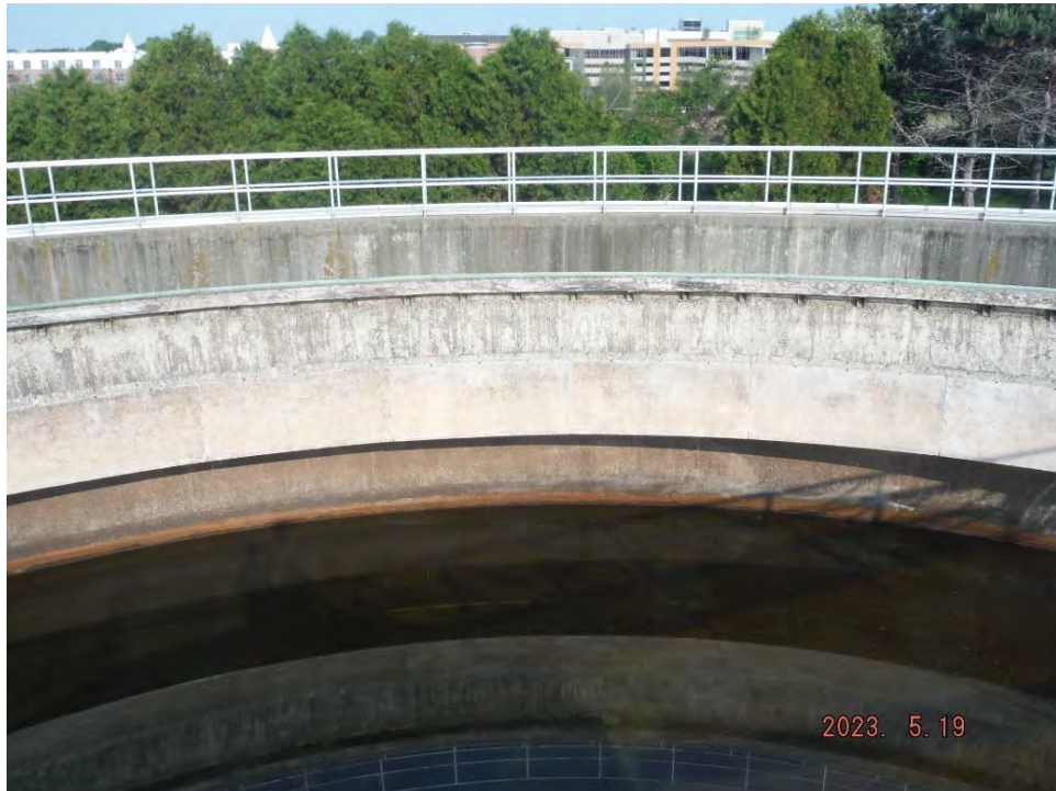
Tank #4 – General view of the inside face of Segment 1-12, looking north.
