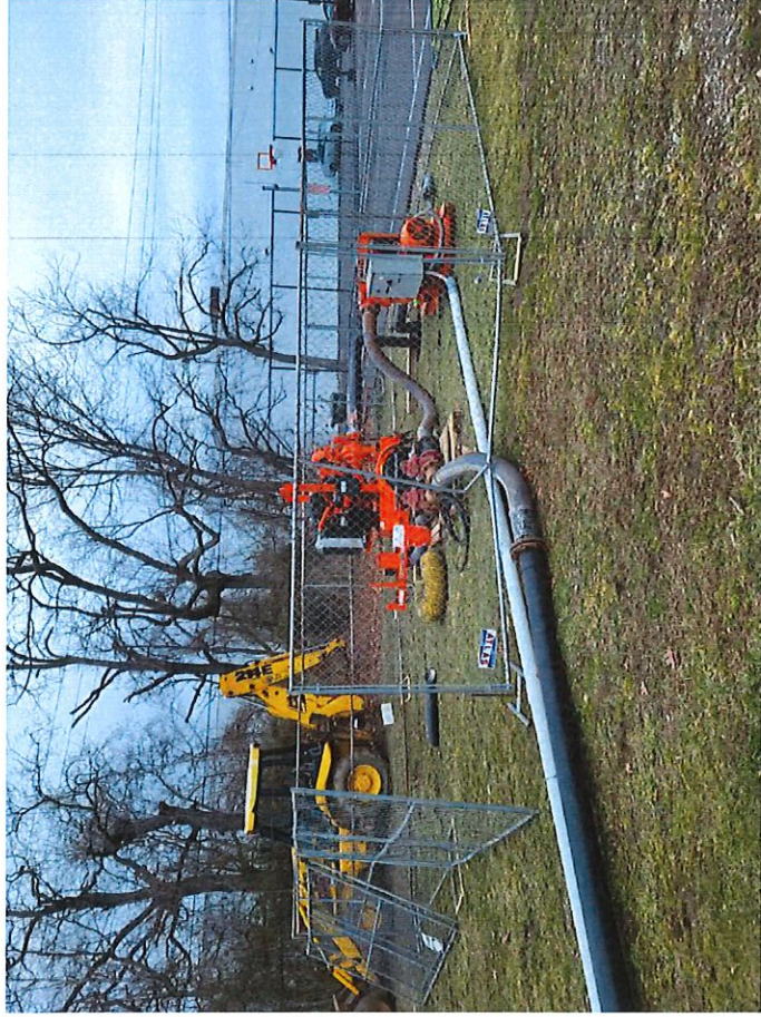
Pump Station Bypass Set up
