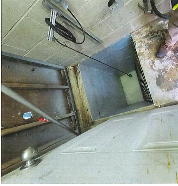
Wet well entrance after coating and installation of new floats
