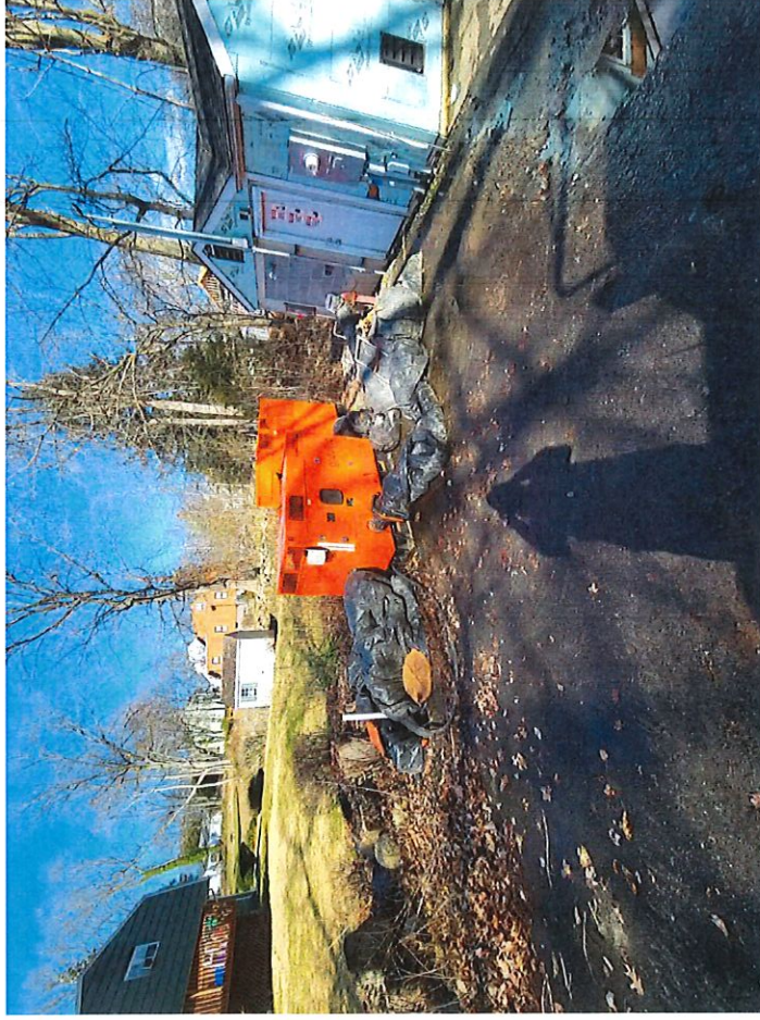
Pump Station Bypass Set up
