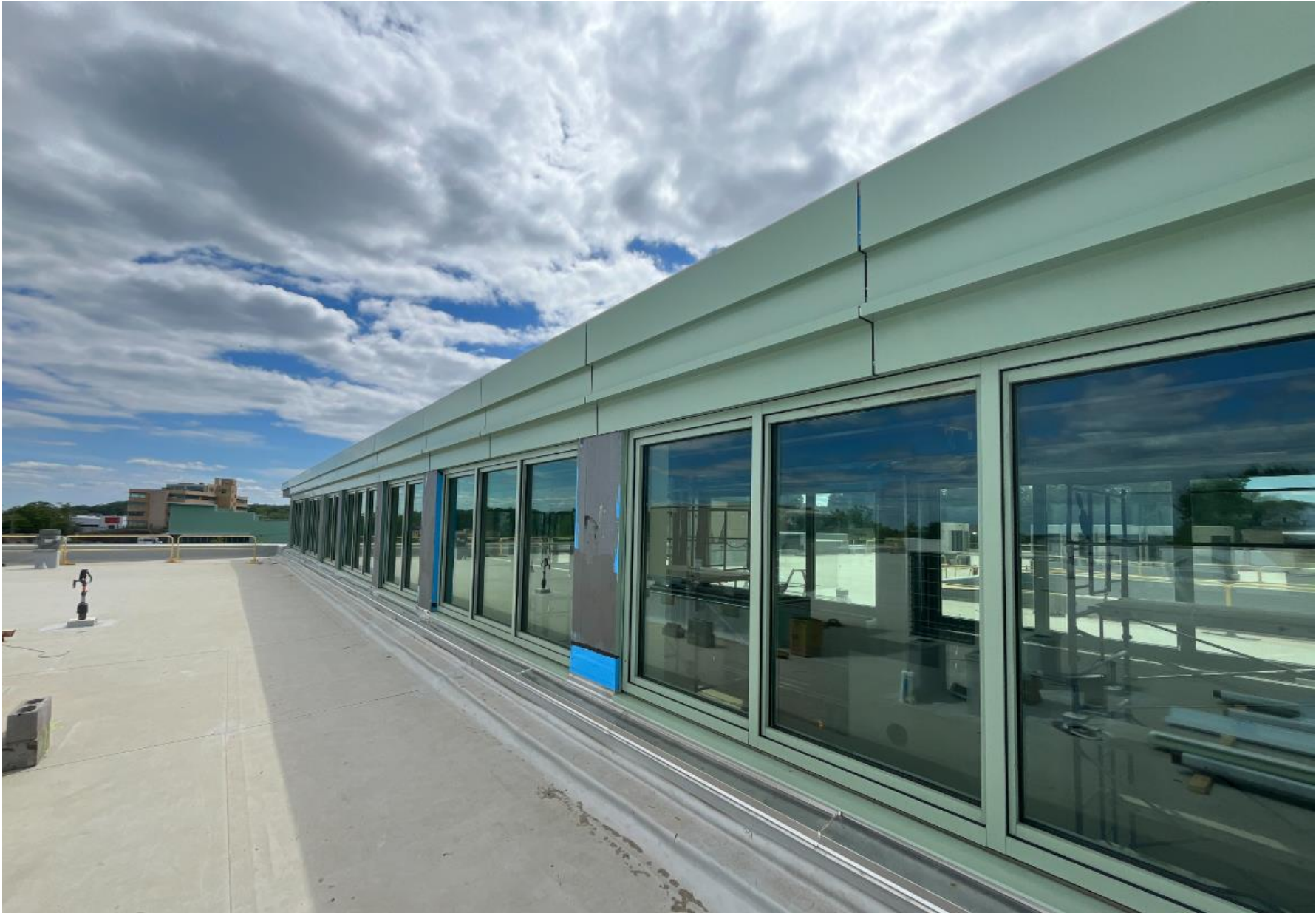
Roof & Glazing at Main Stair 5/20/25
