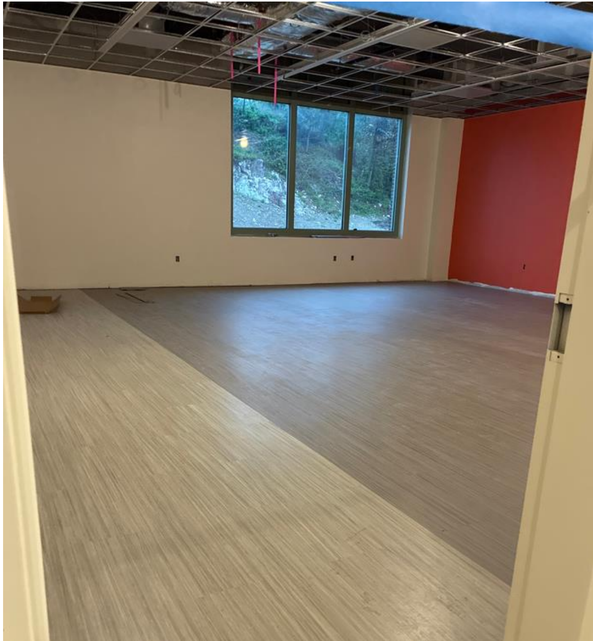
Classroom Ceilings & Flooring 5/15/25
