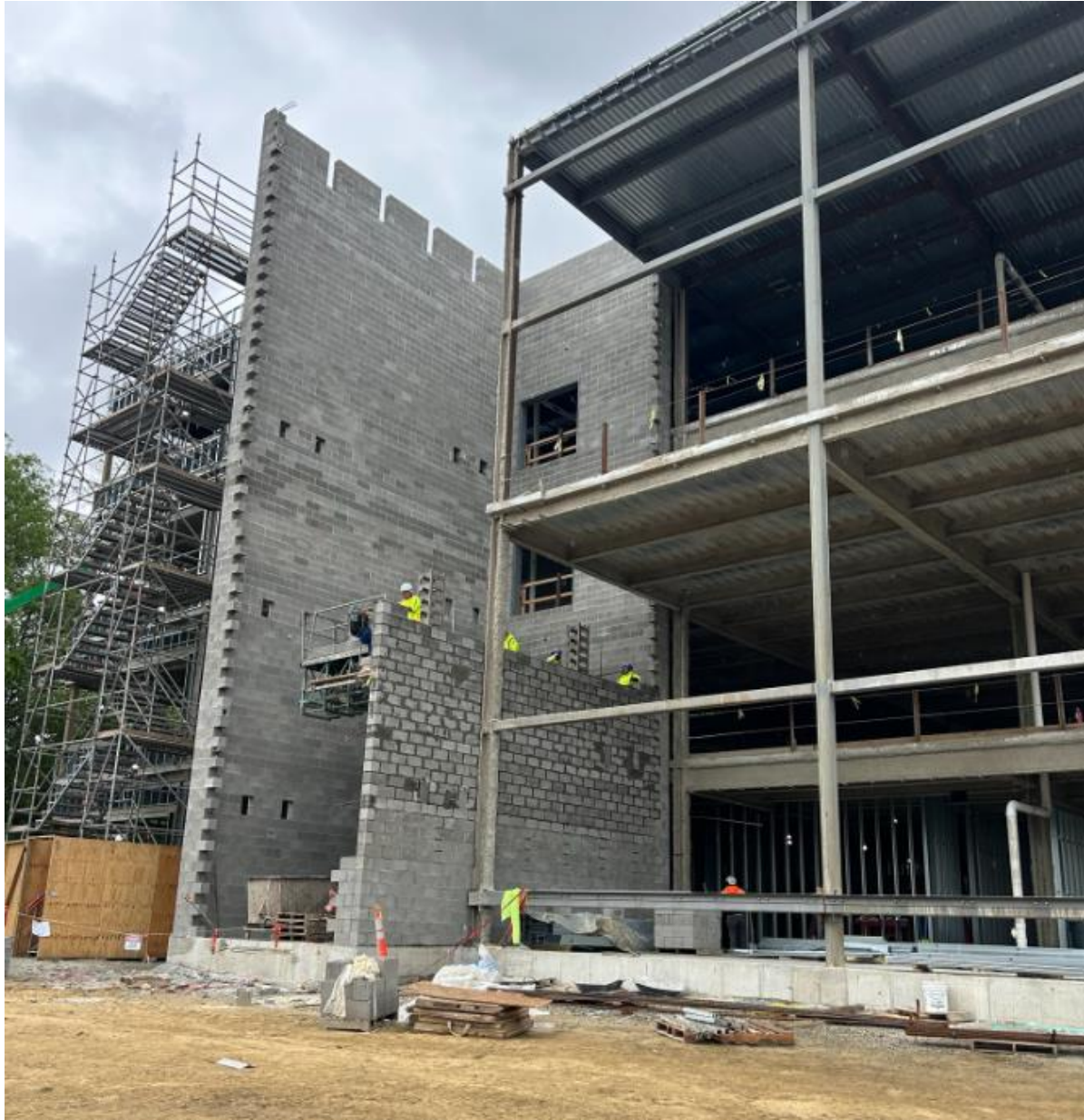
Masonry Stair Walls 5 /21/25
