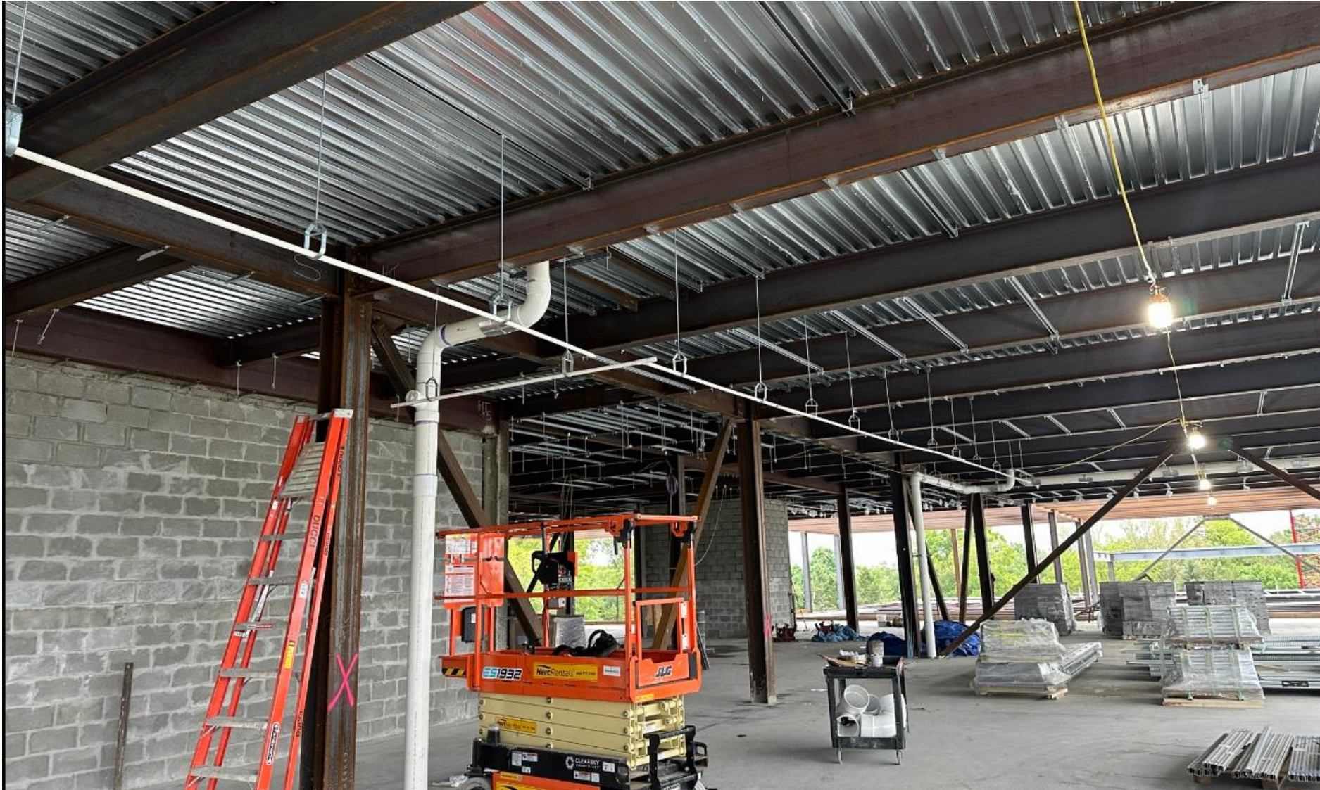
Interior MEP Overhead Rough-in 5/21/25
