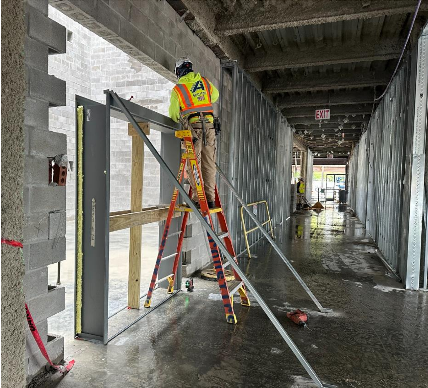
Interior Metal Framing and Door Frames 5/22/25
