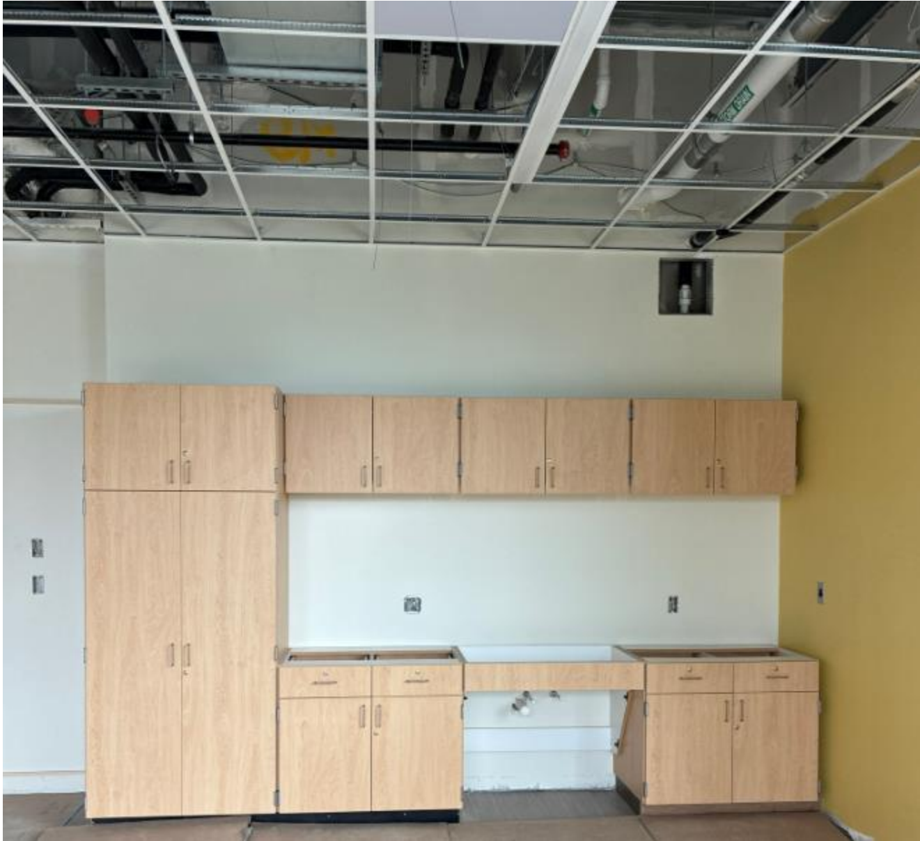
Classroom Ceilings & Millwork 5/17/25
