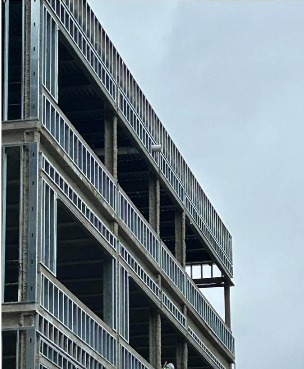
Exterior Metal Framing 5/21/25
