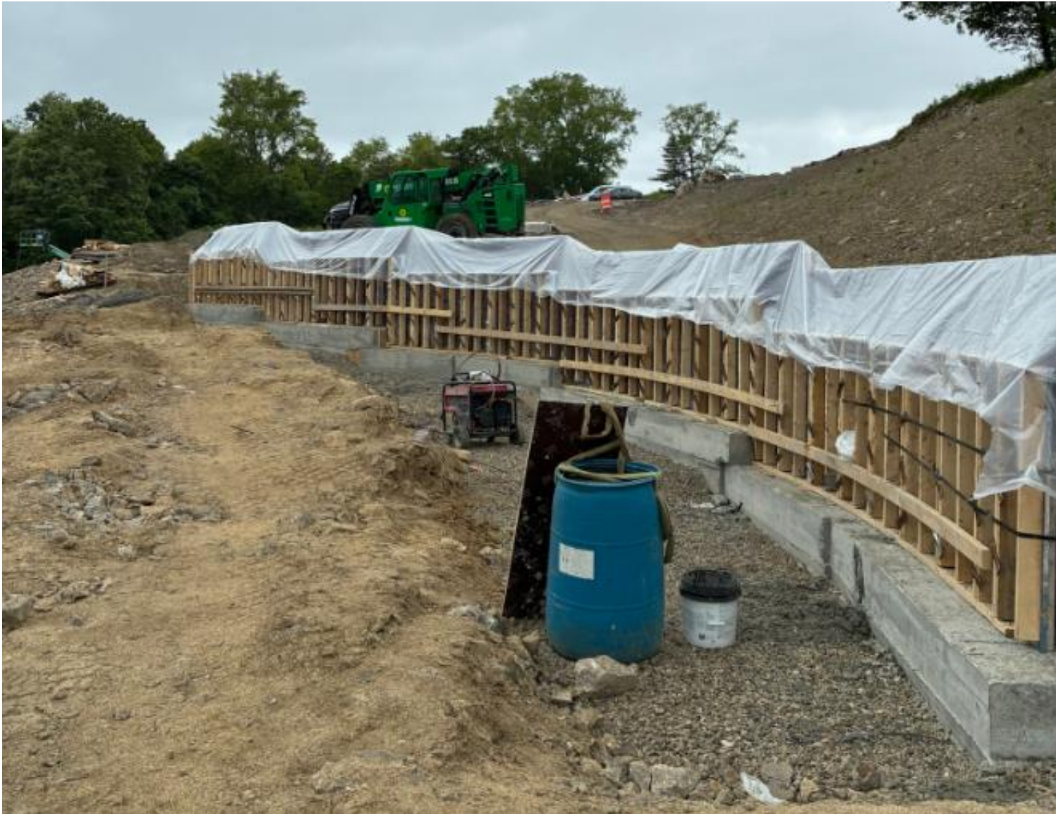
Site Development – Retaining Wall at Rear of School 5/21/25
