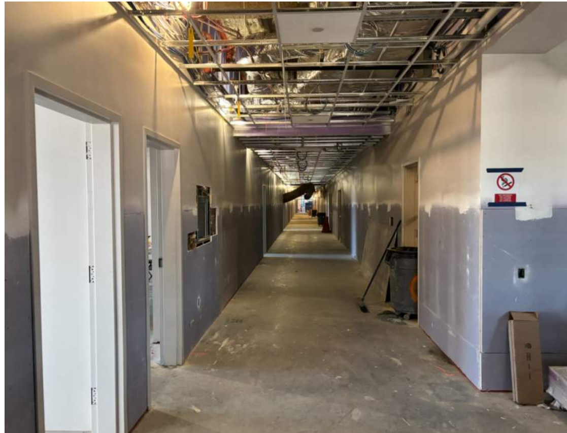
Corridor with Door Frames, Wall Finishes and Ceiling Grid – 3/24/26
