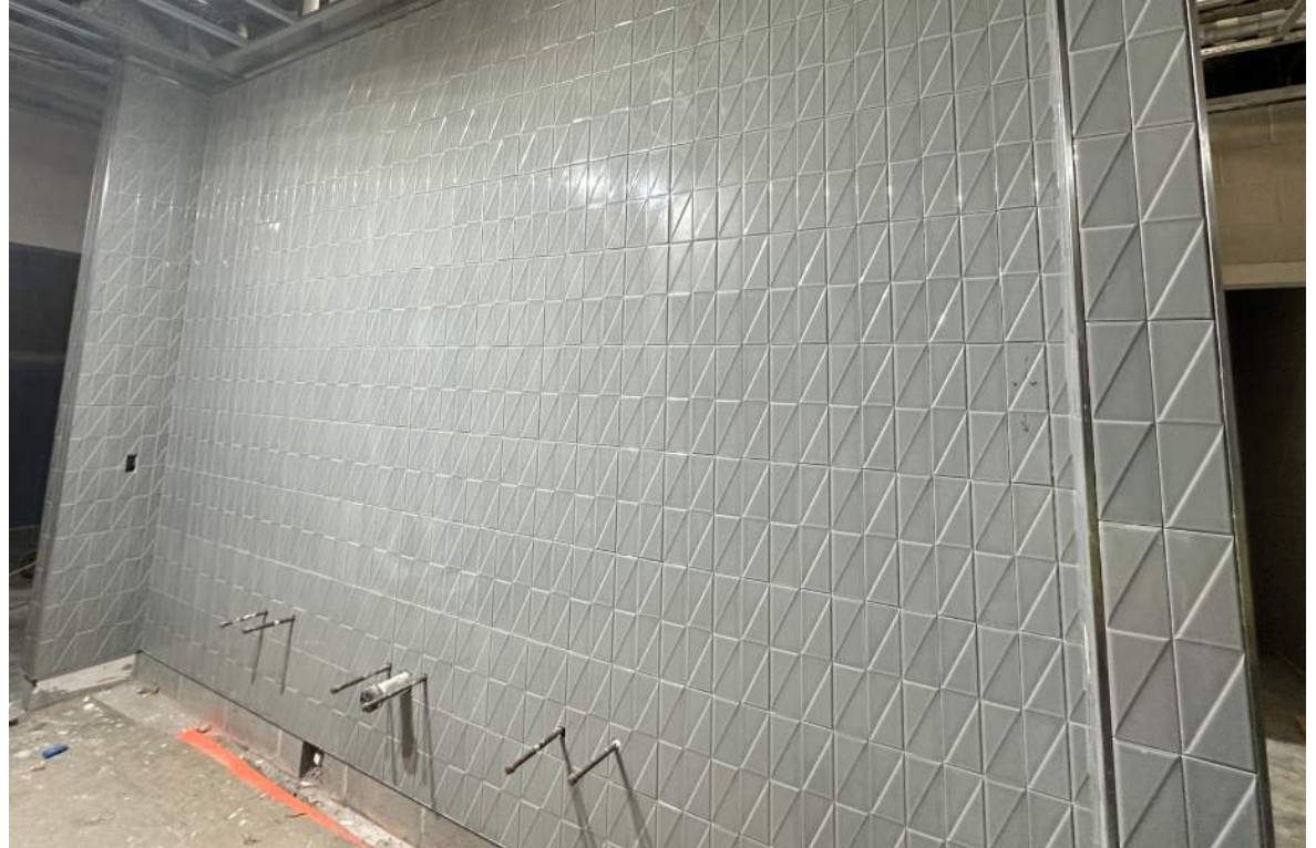
Interior Framing with Glazing & Interior Wall Tile – 3/25/26
