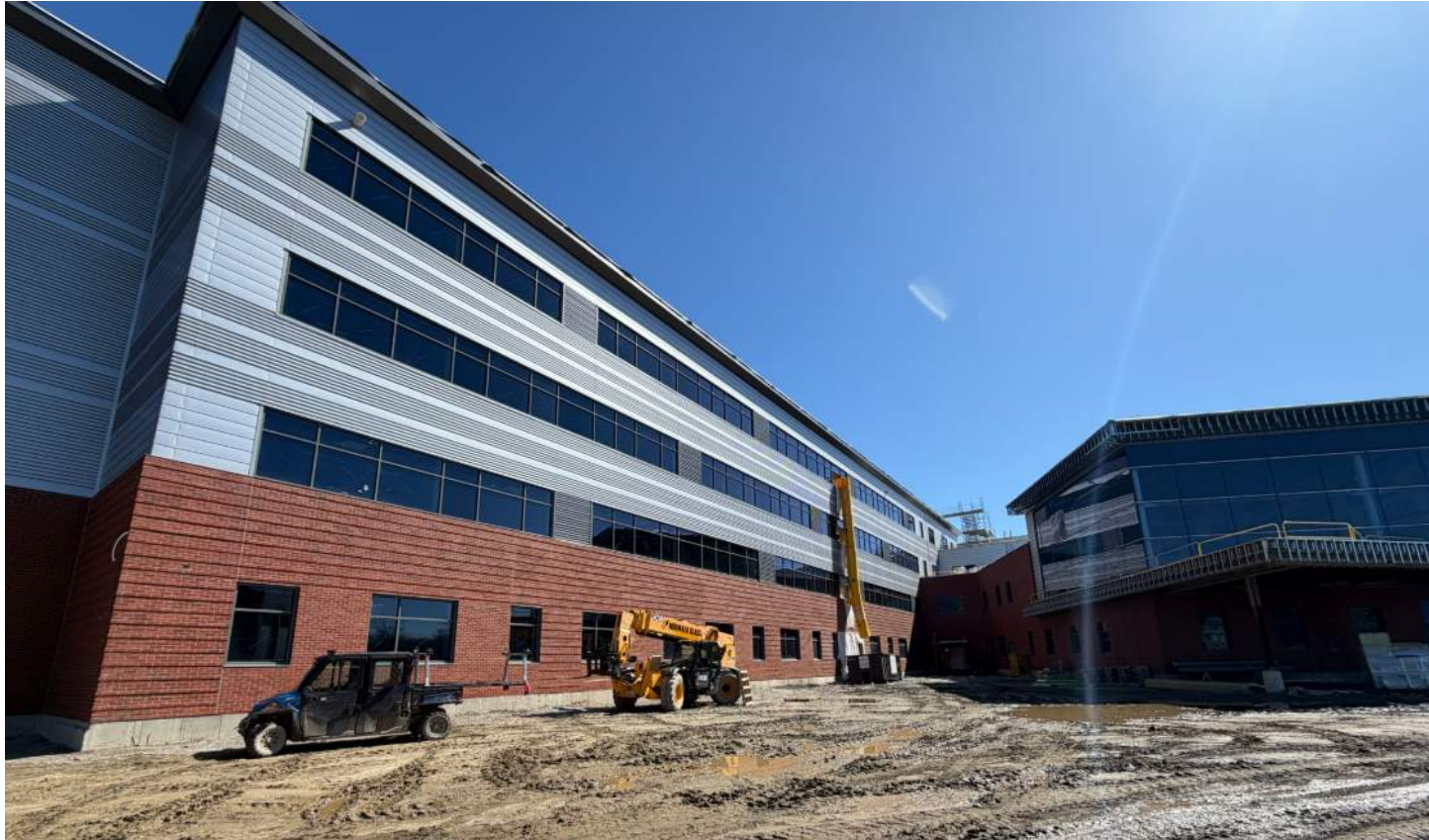
Building Envelope at NHS Wing & Main Entrance – 3/24/26
