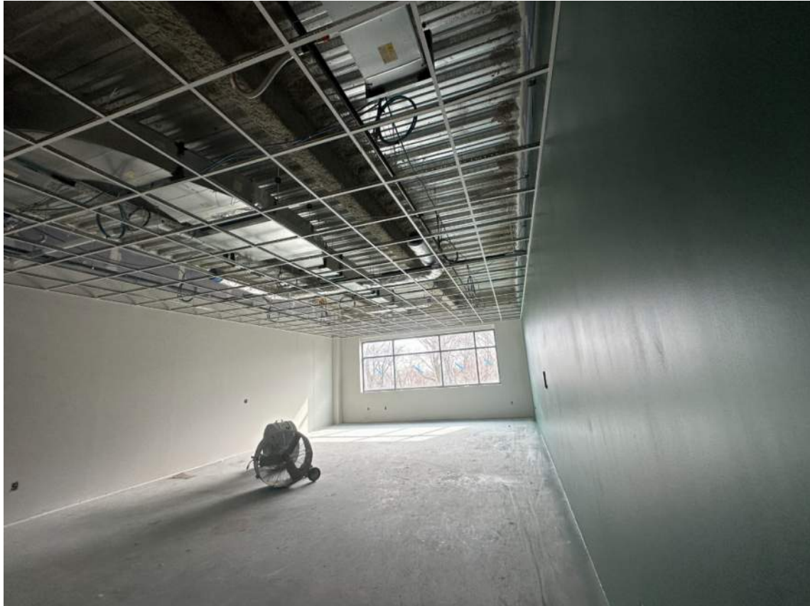
Classroom with Wall Finishes and Ceiling Grid – 3/25/26
