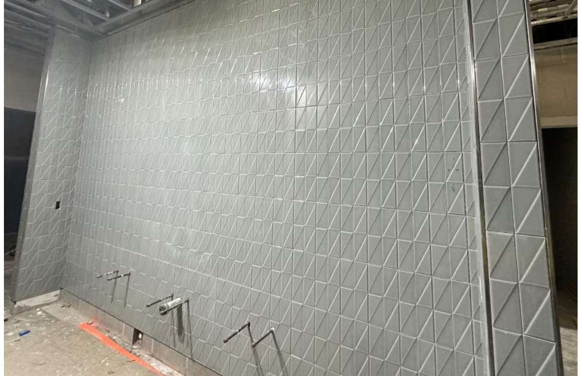
Interior Framing with Glazing & Interior Wall Tile – 3/25/26
