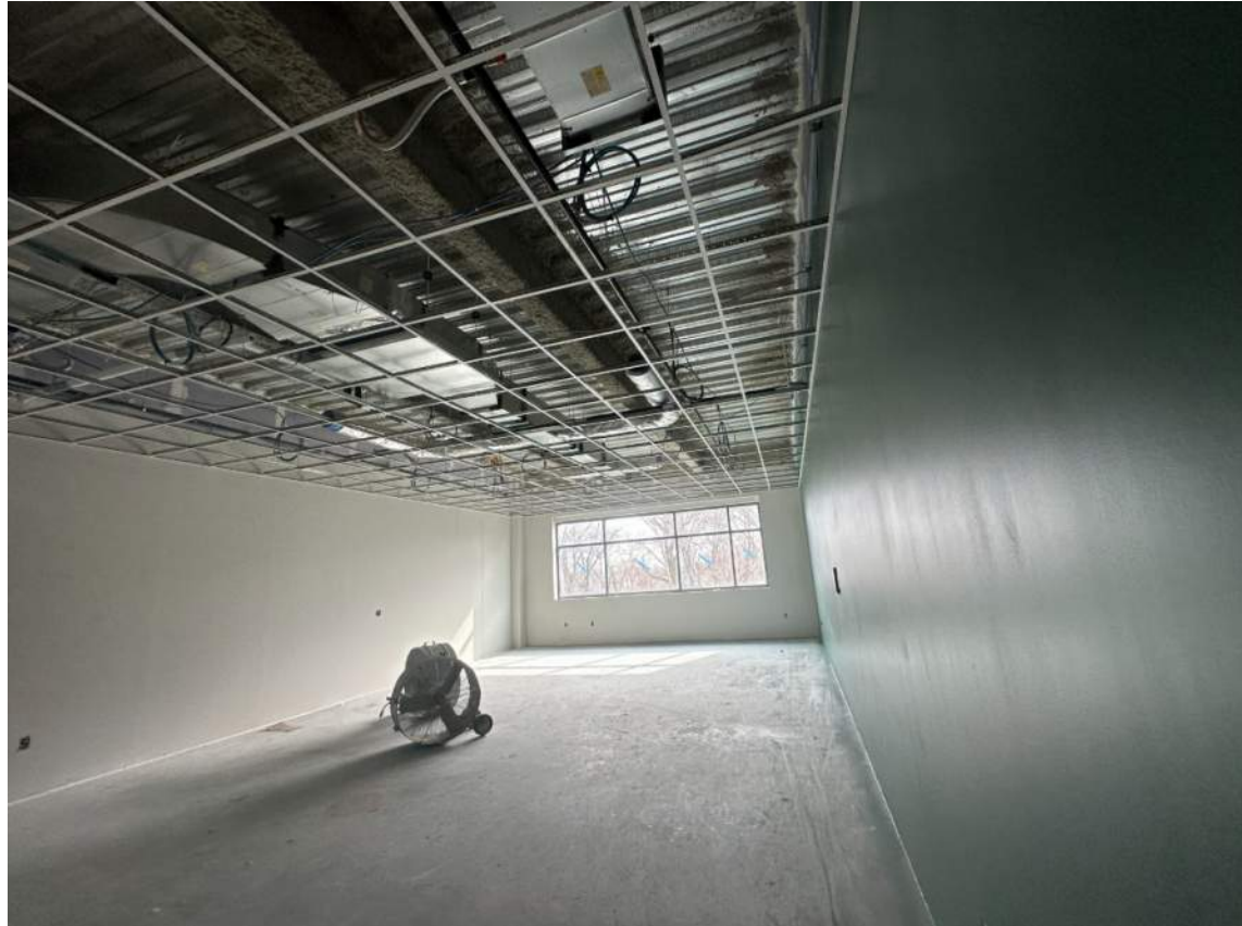
Classroom with Wall Finishes and Ceiling Grid – 3/25/26
