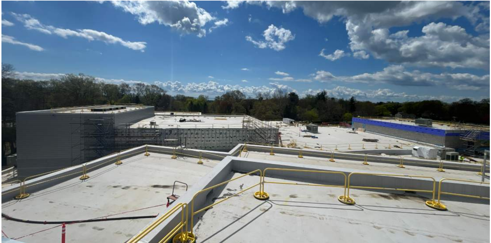
Roofing at P-TECH Auditorium, Gym, Aux Gym – 4/17/26
