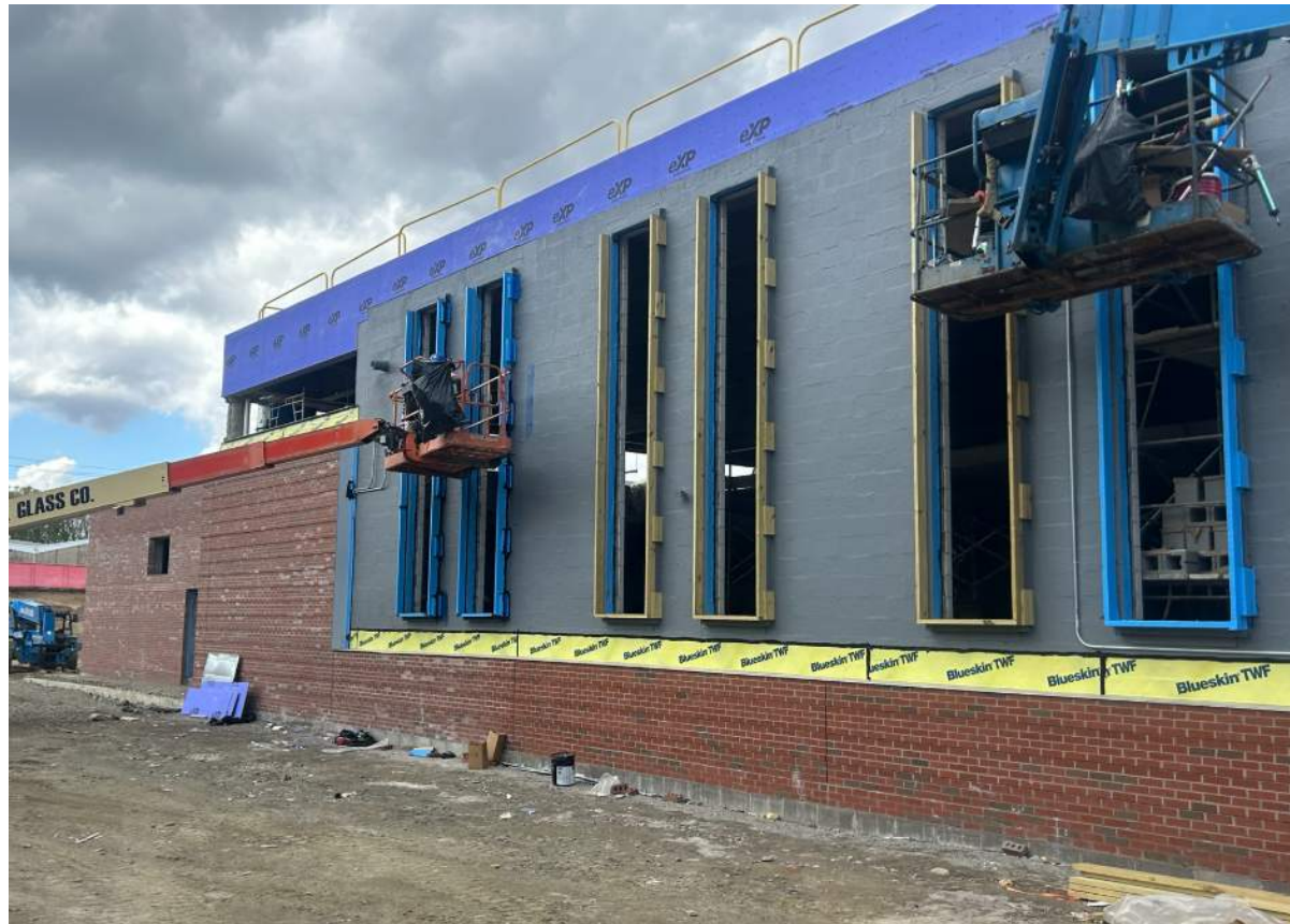
Pool Building Envelope – 4/20/26
