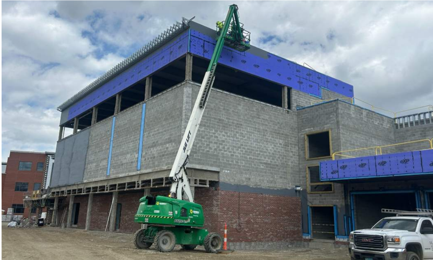
P-TECH Wing, Aux Gym, Pool Entrance Vestibule – 4/20/26
