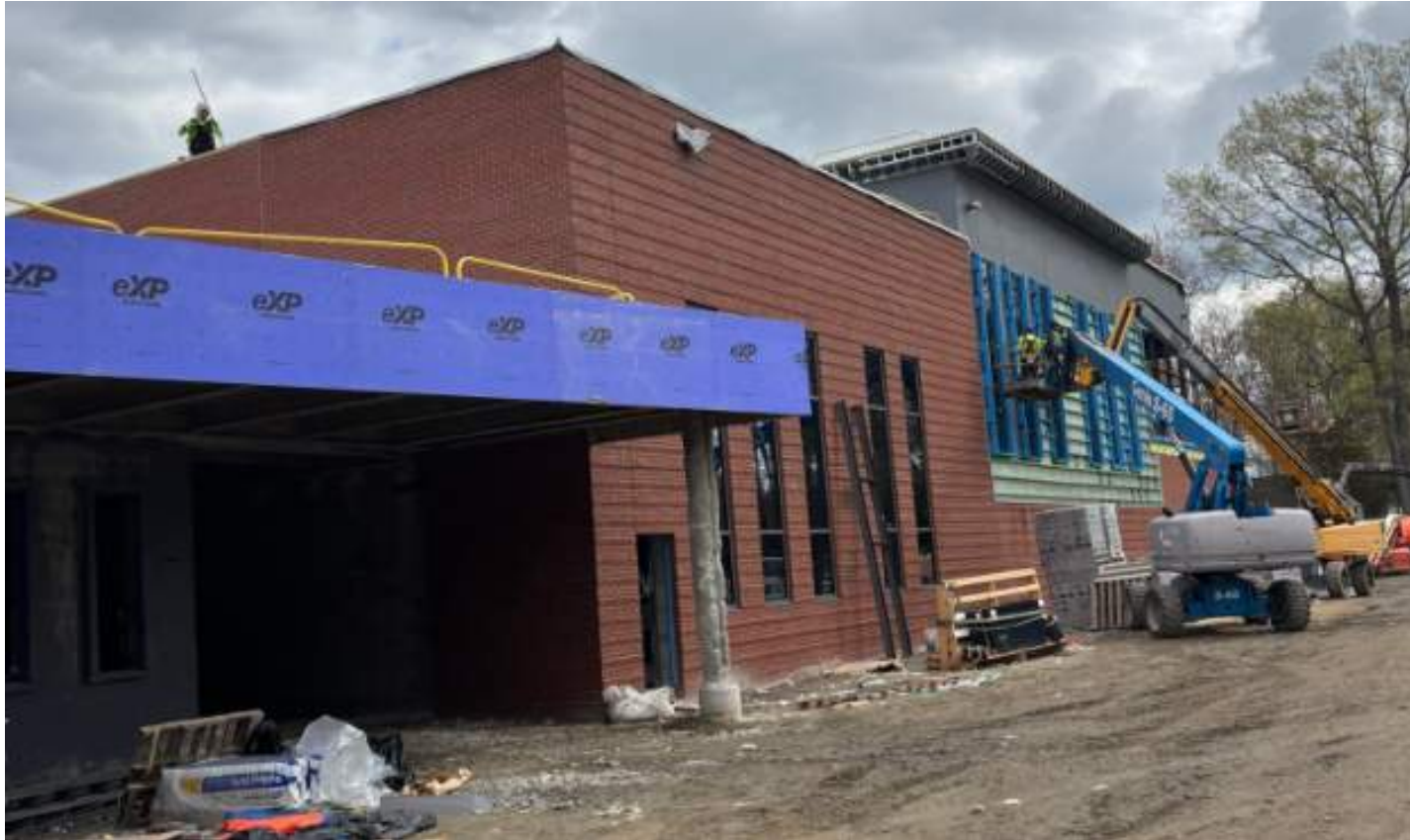
Performing Arts Entrance & Band Room – 4/20/26
