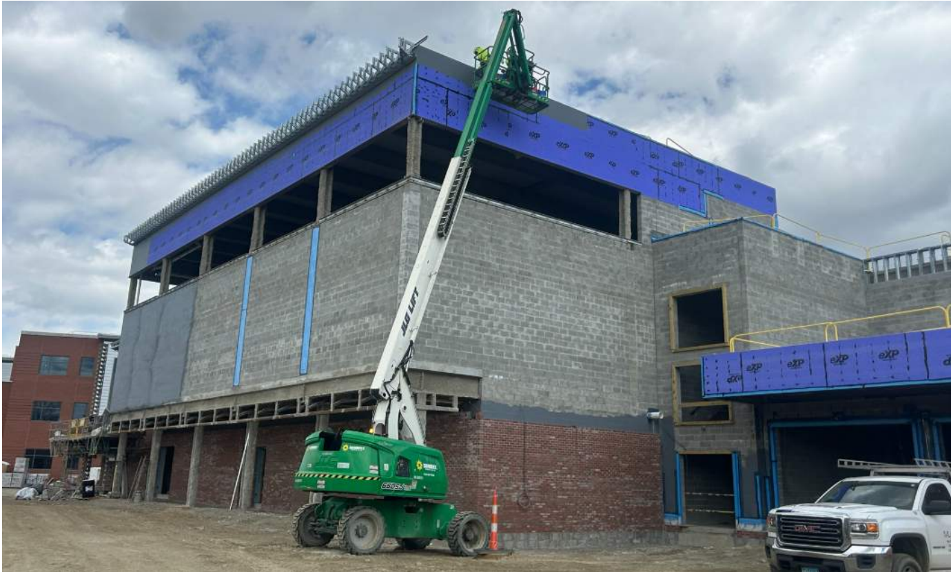
P-TECH Wing, Aux Gym, Pool Entrance Vestibule – 4/20/26
