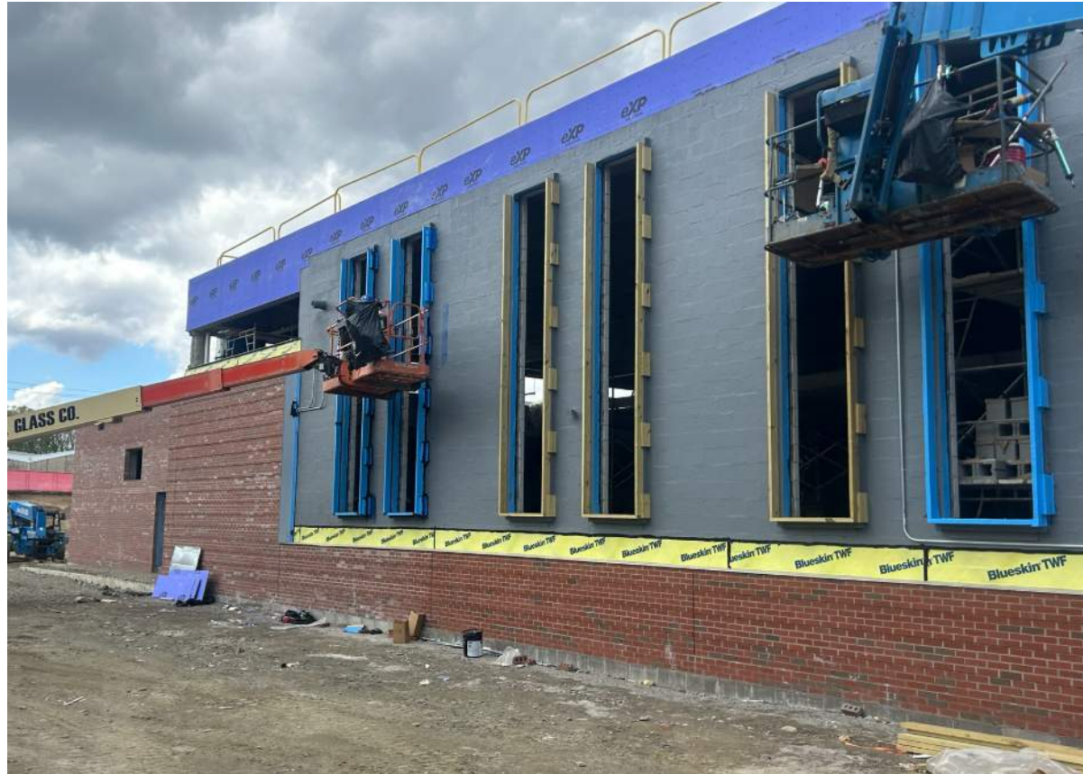
Pool Building Envelope – 4/20/26
