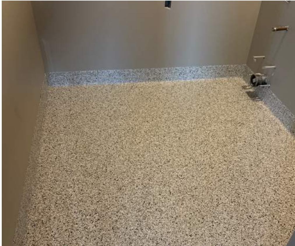
Bathroom Resinous Flooring – 5/19/25
