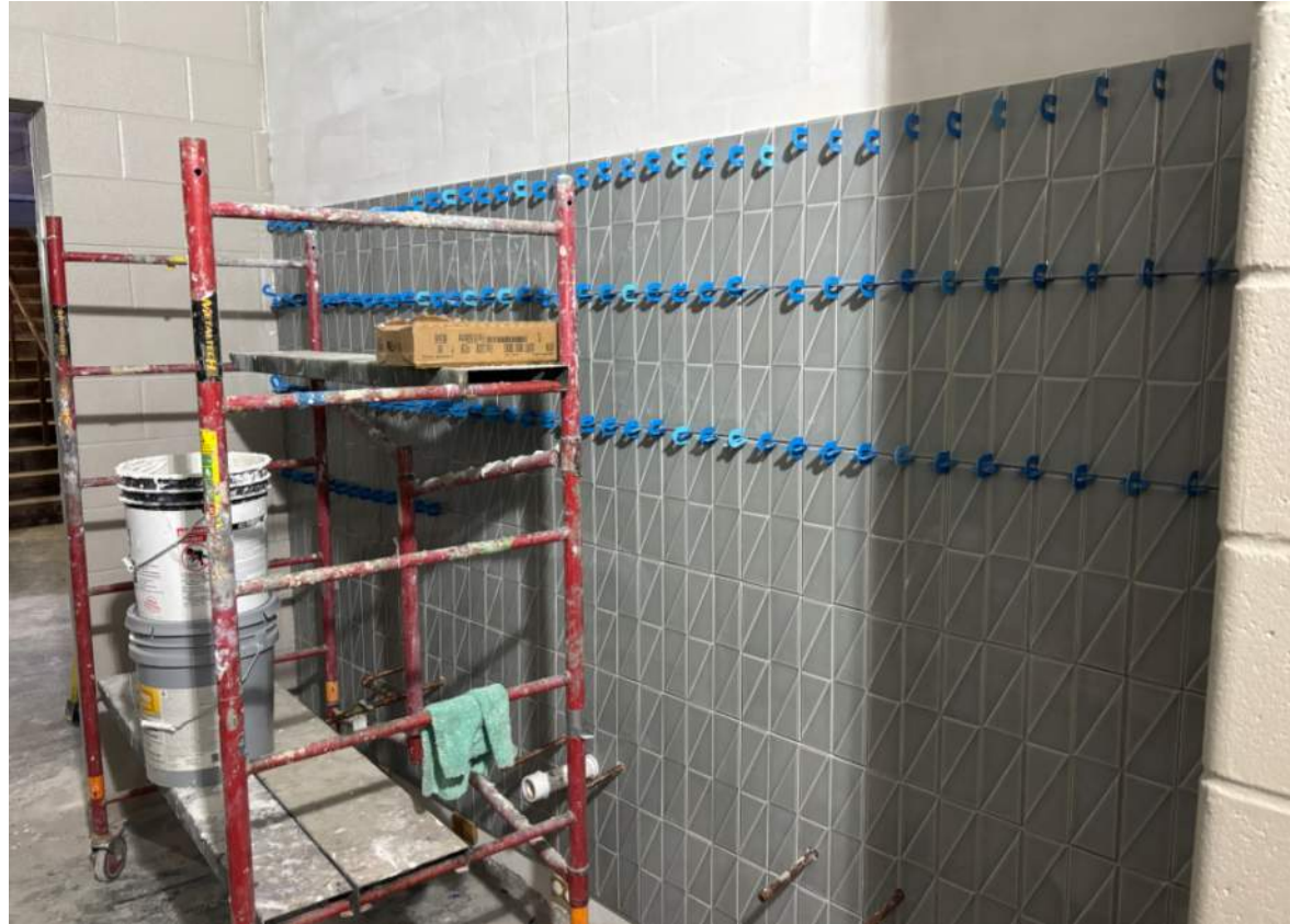
Bathroom Wet Wall Tiling – 5/19/25
