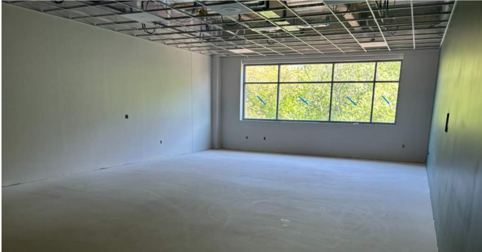
Classroom Finishes with Ceiling Grid and Floor Prep – 5/18/2026
