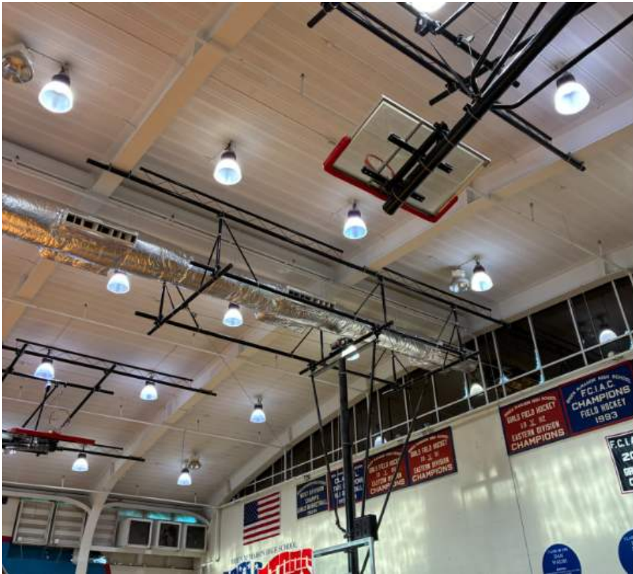
Gym Duct Insulation – 5/6/26
