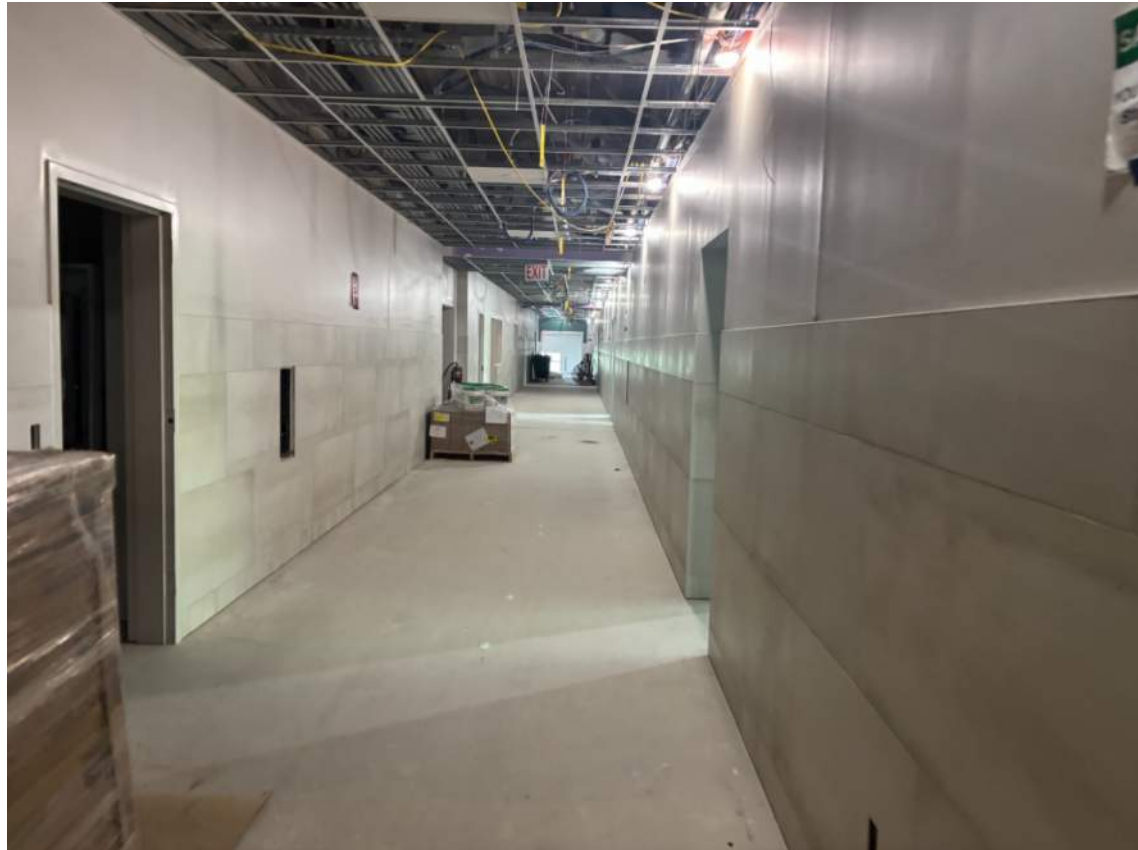
Interior Corridor with Ceiling Grid & Wall Tile – 5/18/26
