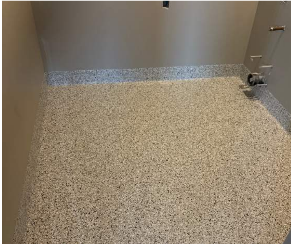
Bathroom Resinous Flooring – 5/19/25
