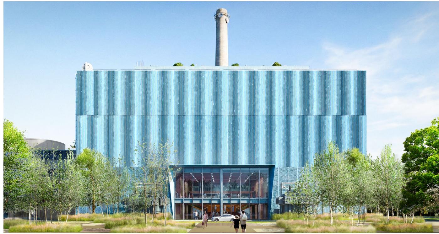
A WELCOMING ARRIVAL TO THE BUILDING The plant's two historic transformers frame the main entryway and guest drop-off at the Turbine Hall.
