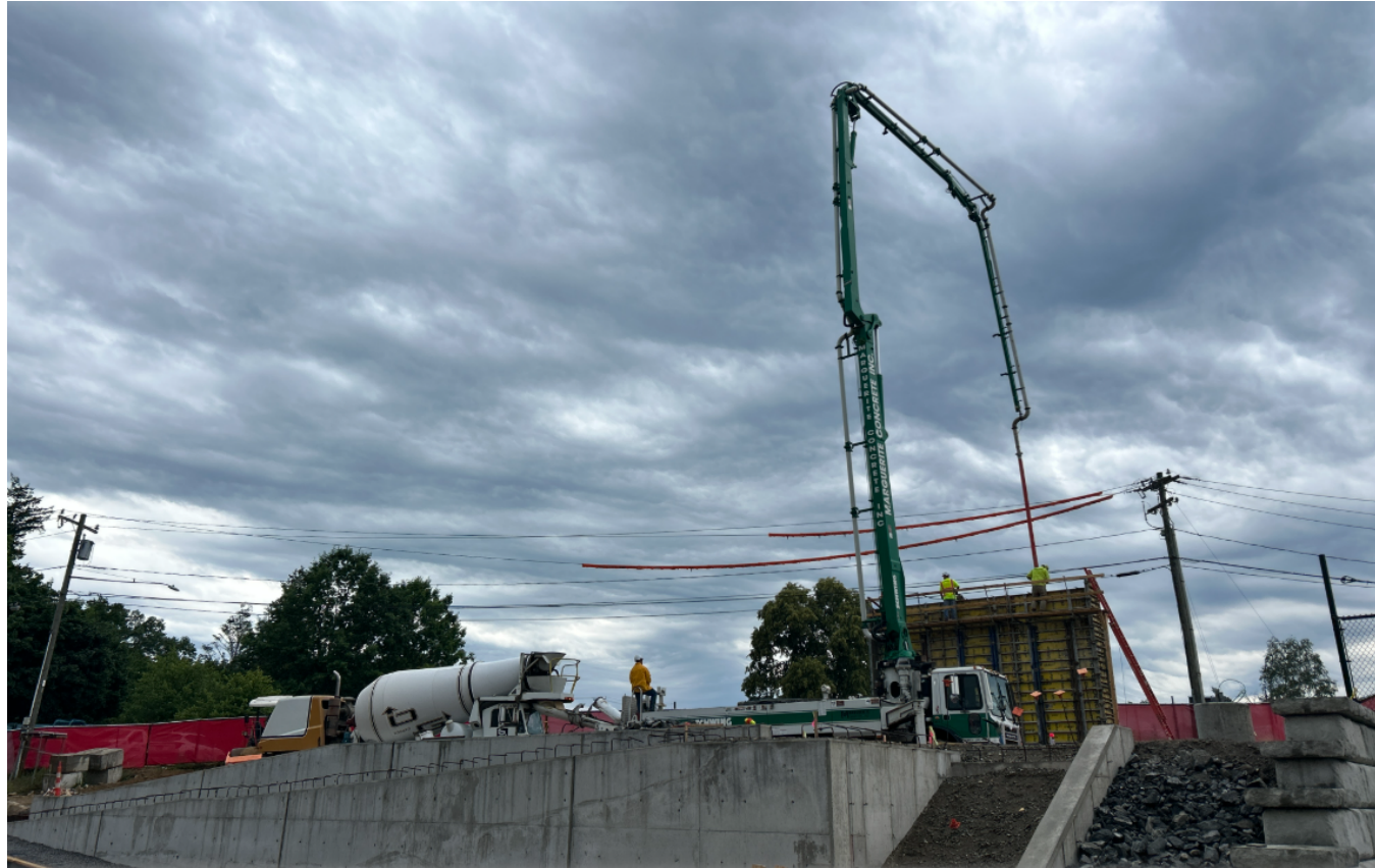
Site Concrete Ramp/Stair & Ball Wall – 6/22/26
