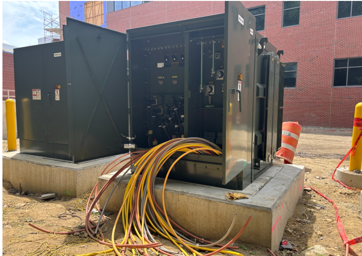
New Electrical Service – Transformers and Primary Cabling – 6/19/26
