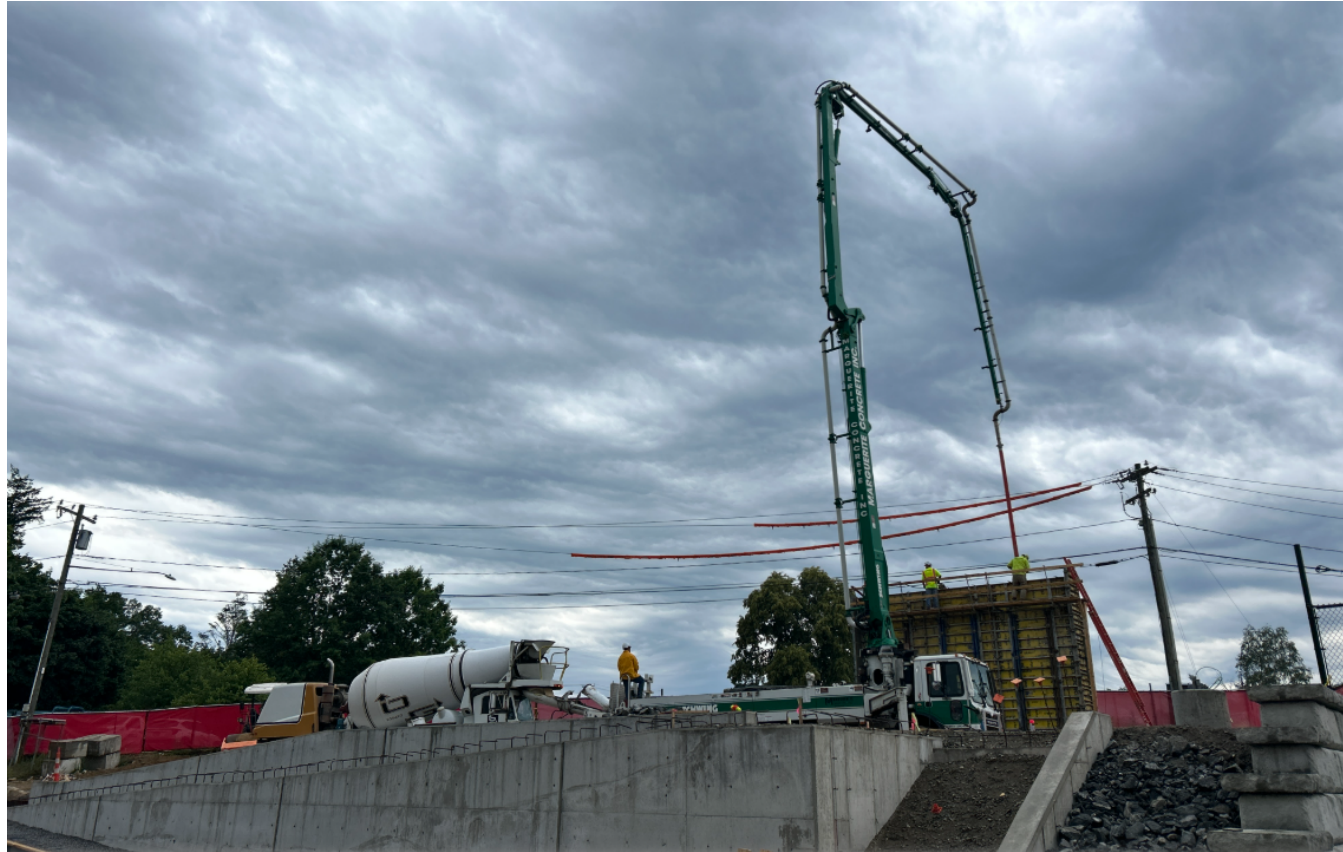
Site Concrete Ramp/Stair & Ball Wall – 6/22/26
