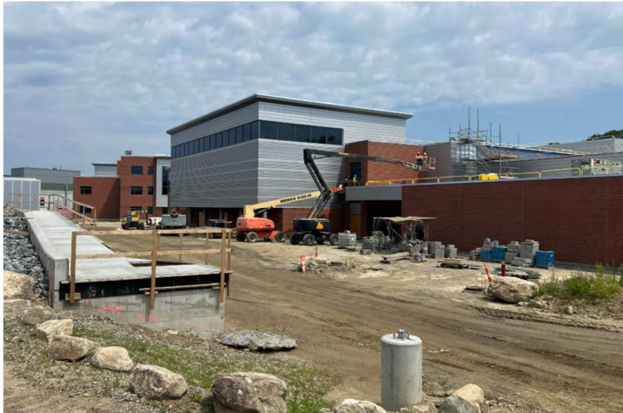
Building Envelope at P-TECH, Aux Gym, Pool – 7/27/26
