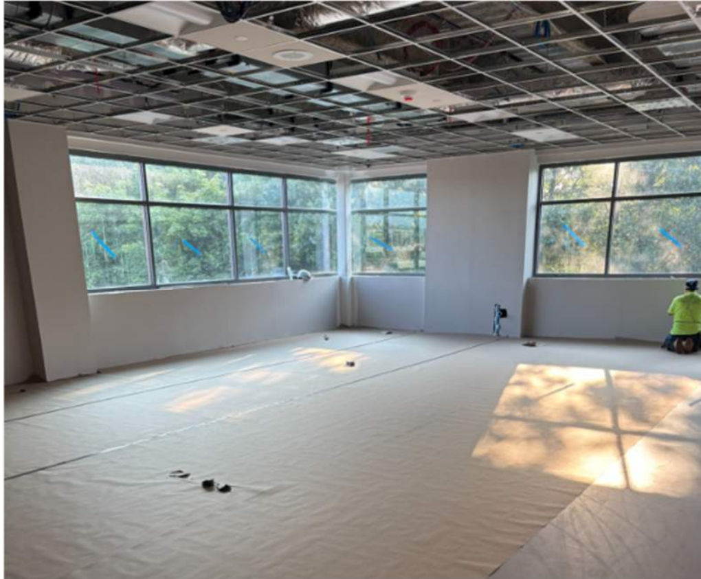
Classroom Finishes with Floor Protection – 7/27/26
