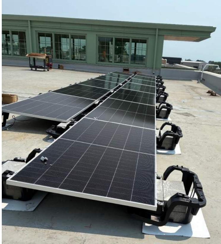
Rooftop PV System Install – 7/28/26
