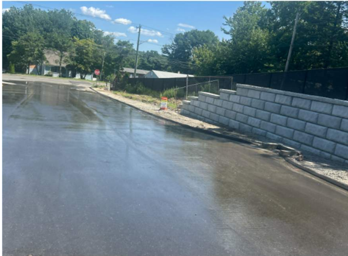
Retaining Wall at Calvin Murphy Drive – 7/24/26
