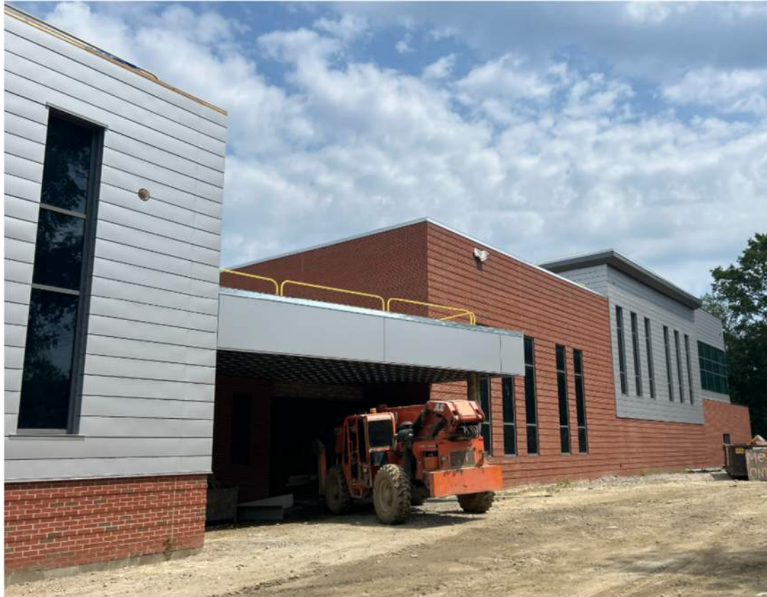
Building Envelope at Performing Arts Entrance – 7/27/26
