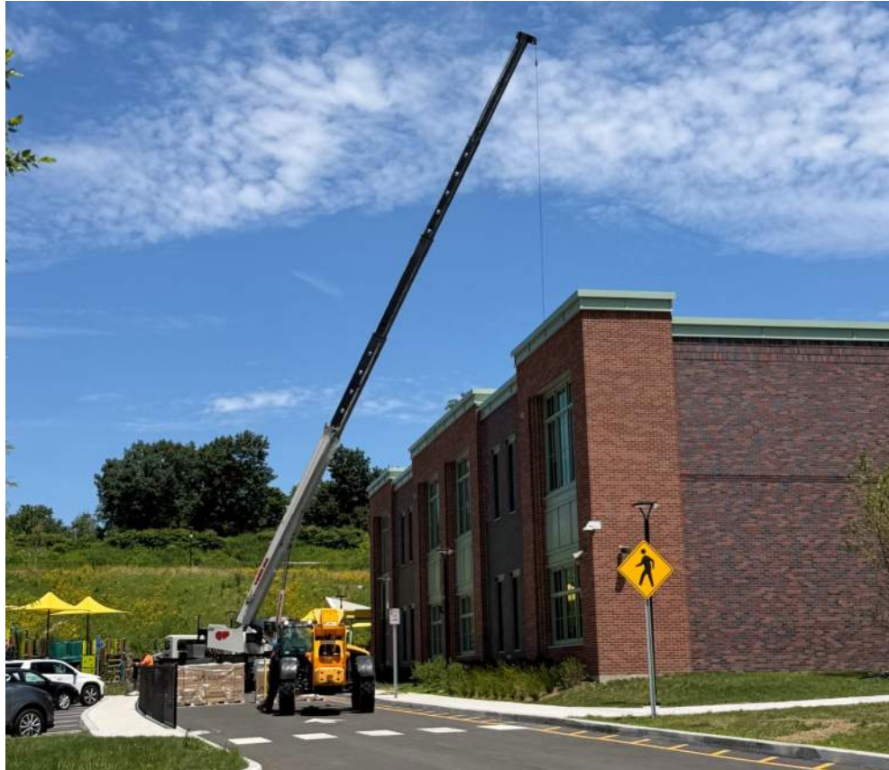
Crane Lifting Solar Equipment to Roof – 7/17/26
