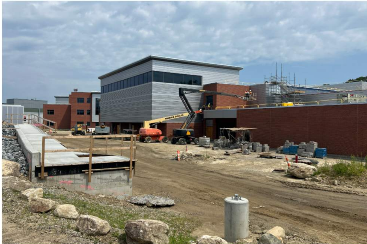
Building Envelope at P-TECH, Aux Gym, Pool – 7/27/26
