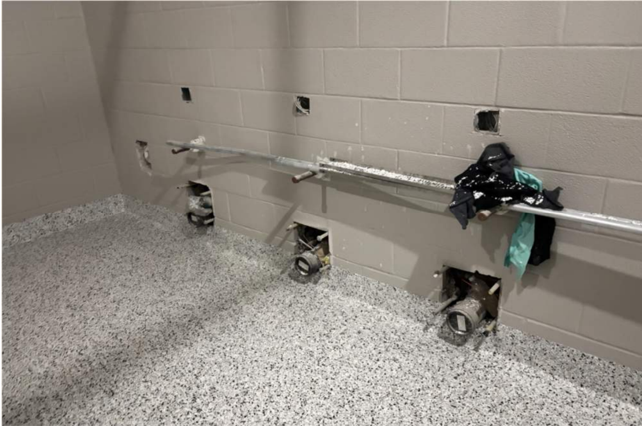
Bathroom Plumbing & Epoxy Flooring – 7/25/26
