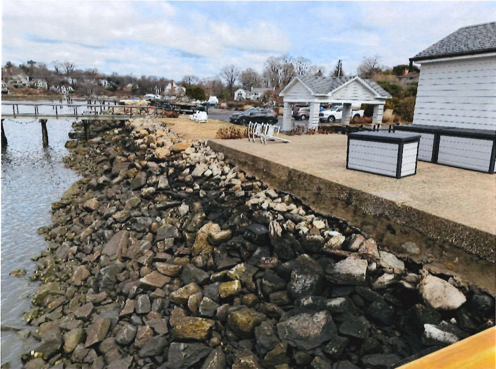
Seawall and Shed Concrete Pad Facing North. Photo Taken March 6, 2025
