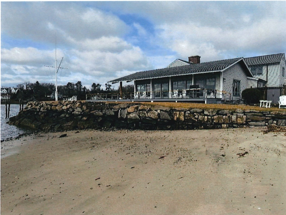
Seawall South of Clubhouse, Facing Northwest. Photo Taken March 6, 2025
