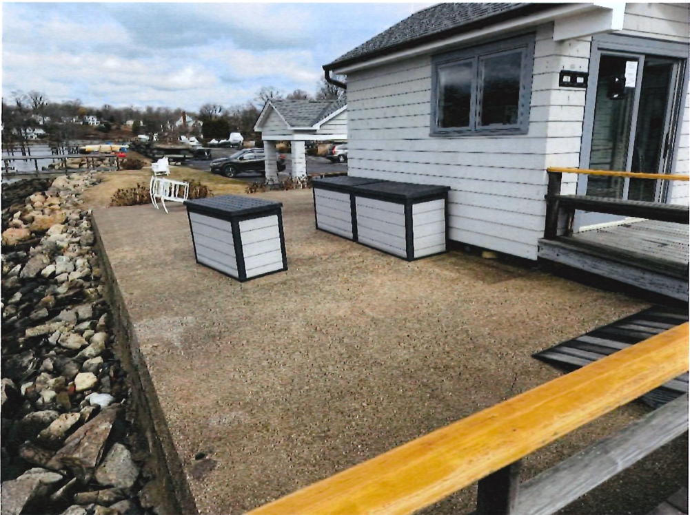
Concrete Shed Pad Facing North. Photo Taken March 6, 2025
