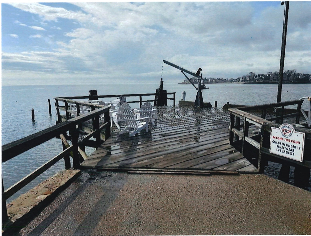
Southern Deck Facing Southwest. Photo Taken March 6, 2025
