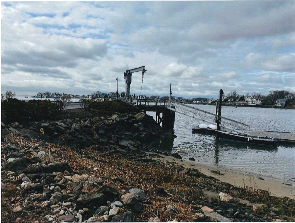
Seawall East of Crane, Facing Southwest. Photo Taken March 6, 2025
