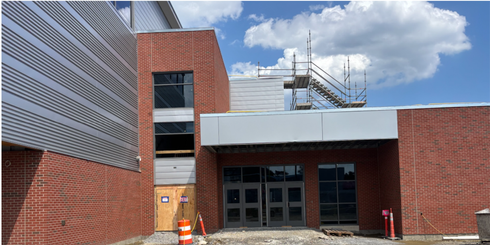
Building Envelope Pool Entrance – 8/24/26
