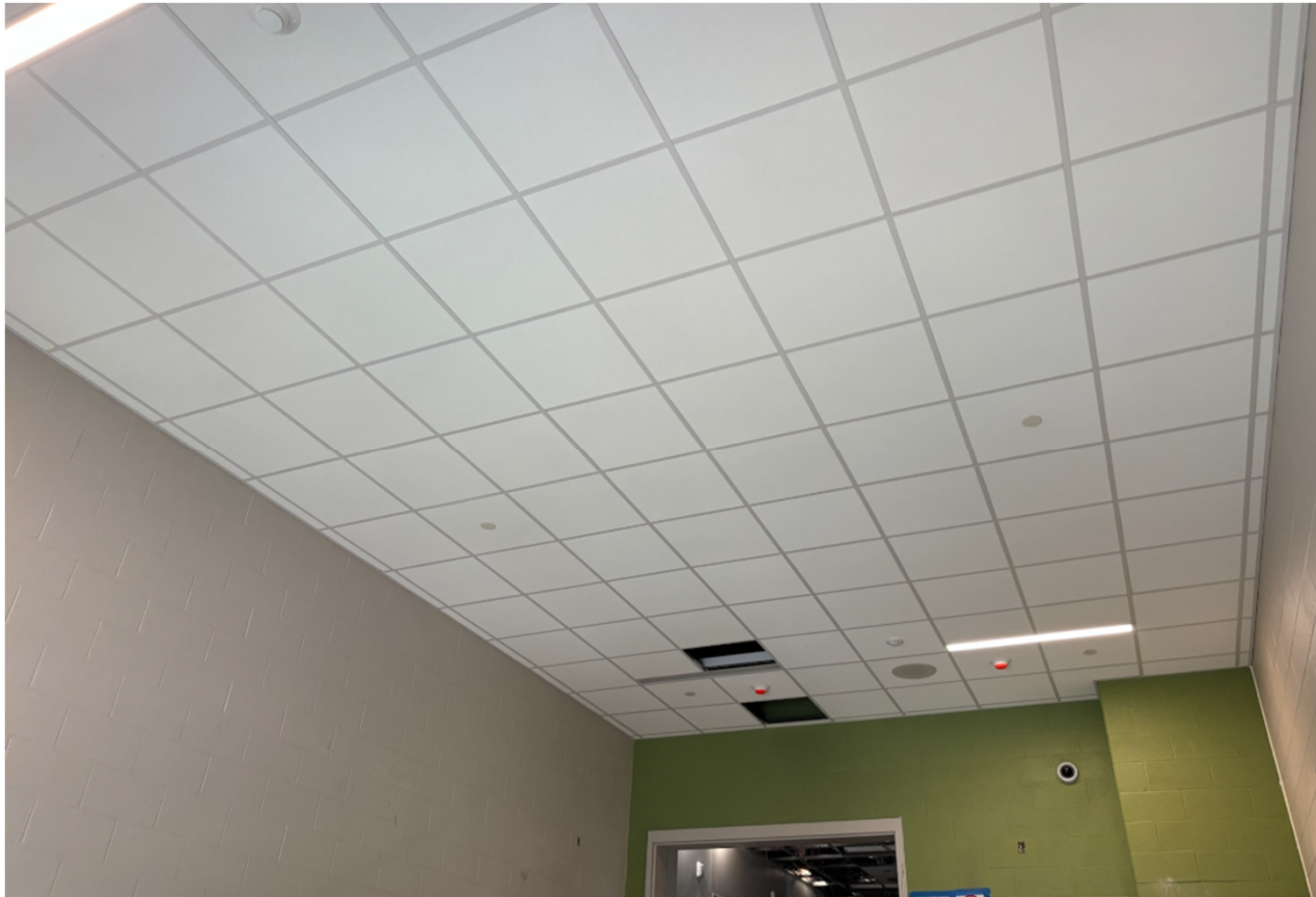
Exit Stair Finishes – 8/24/26
