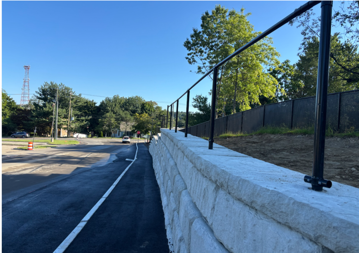
Retaining Wall with Fence & Sidewalk at Calvin Murphy Drive – 8/19/26
