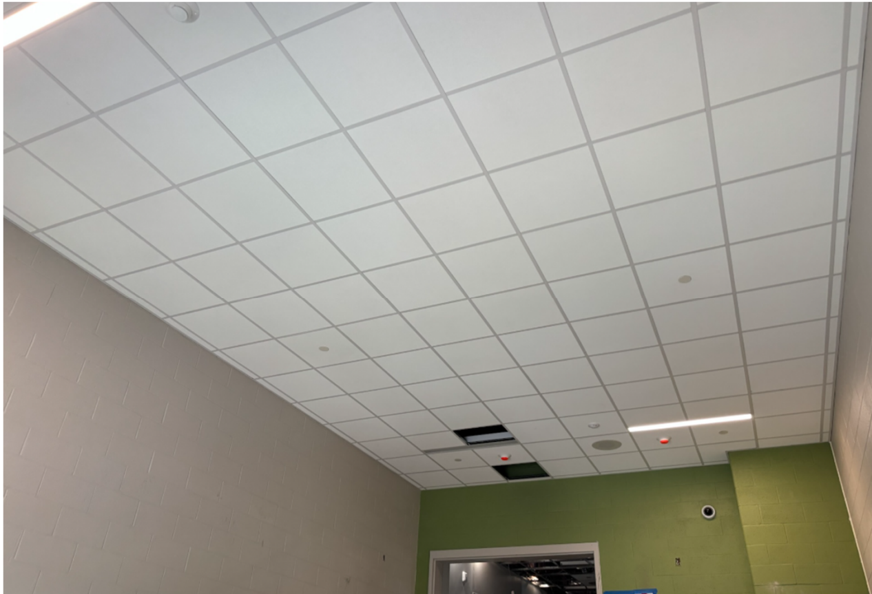
Exit Stair Finishes – 8/24/26
