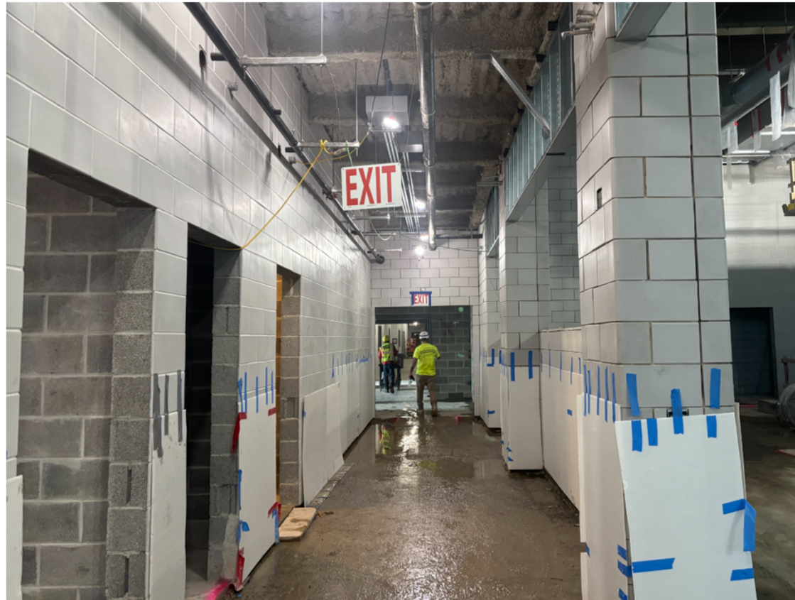
Pool Area Corridor – 8/24/26
