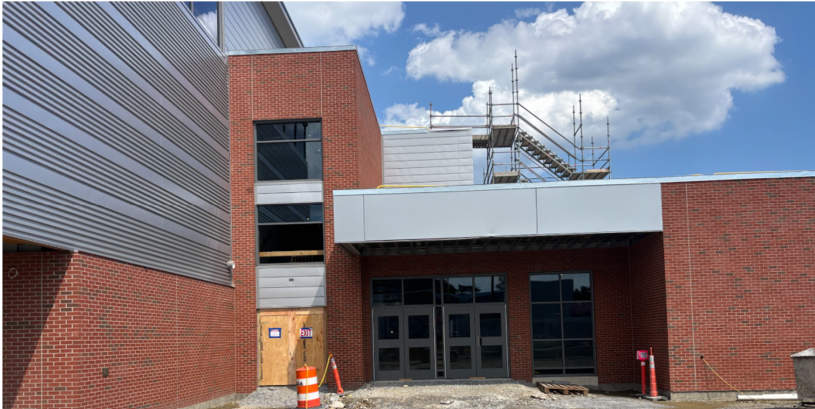
Building Envelope Pool Entrance – 8/24/26
