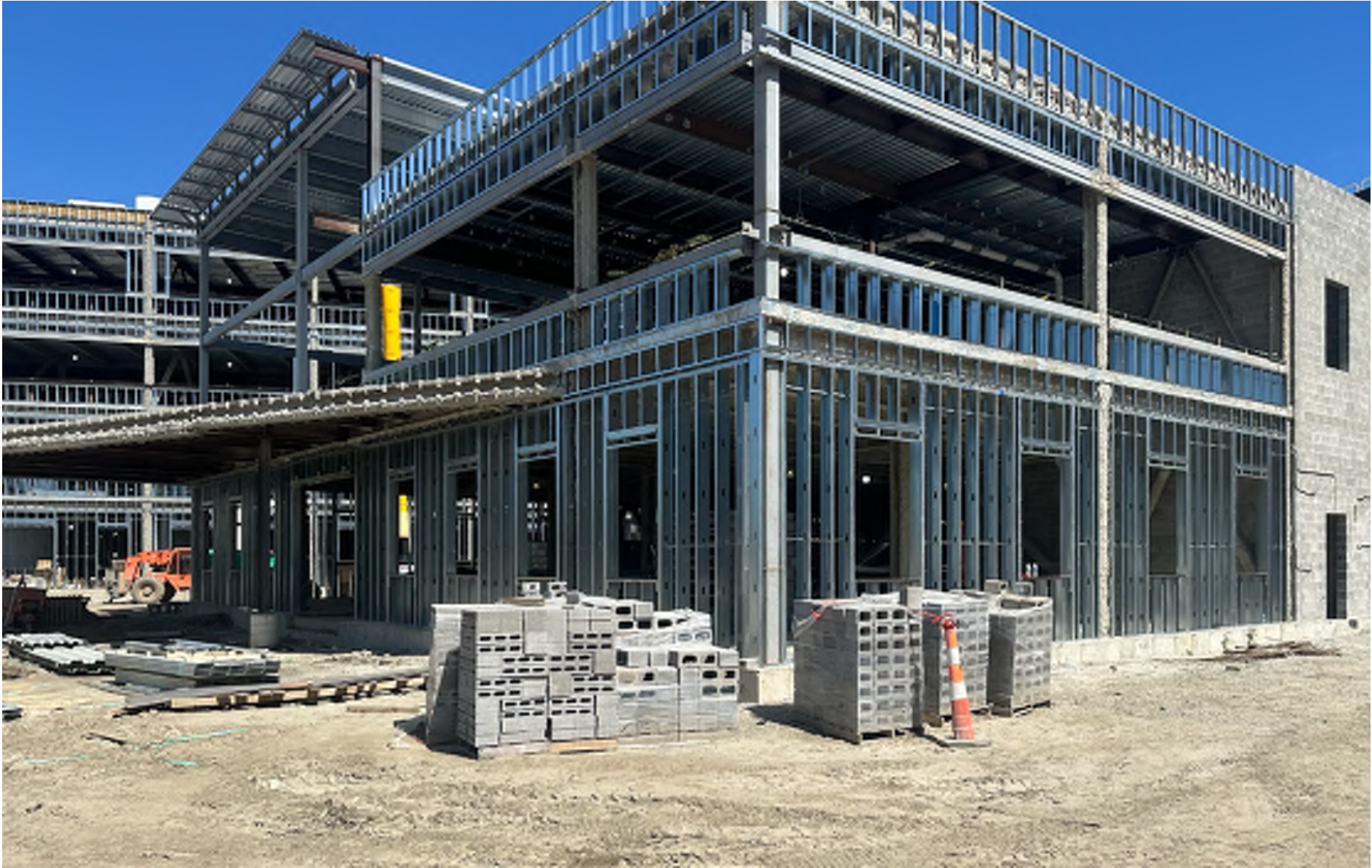
Exterior Metal Framing at Main Entrance 6/24/25
