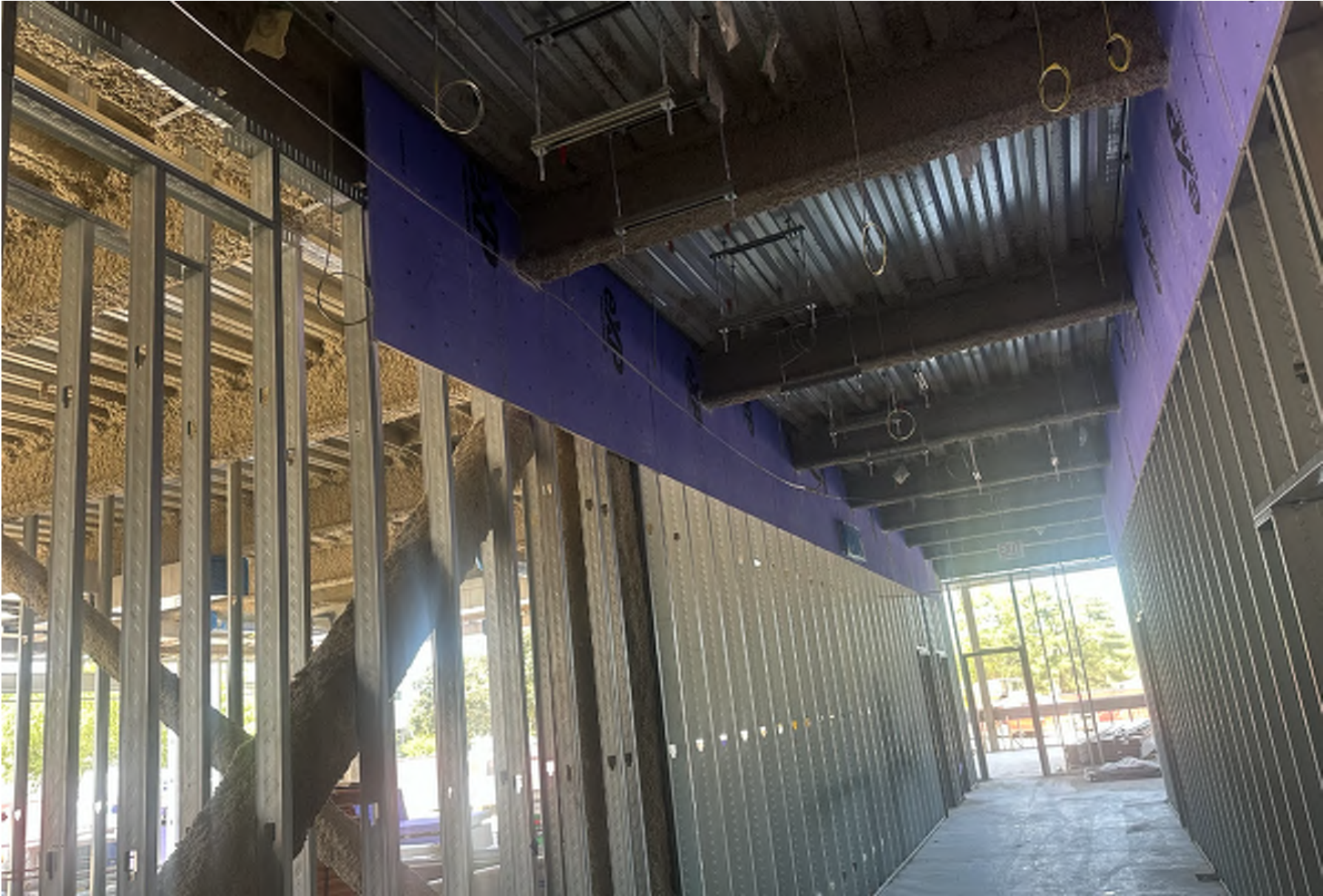
Interior Metal Framing, Top of Wall Sheetrock and MEP Rough-in 6/24/25
