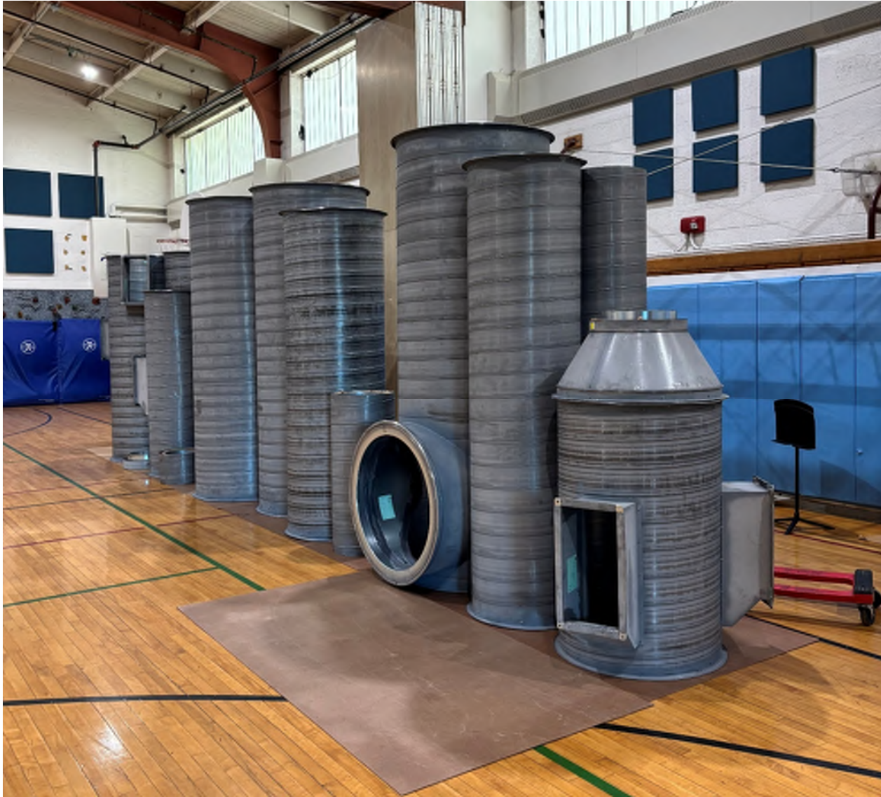
Brookside - New Spiral Ductwork for Gymnasium- 06/25/25
