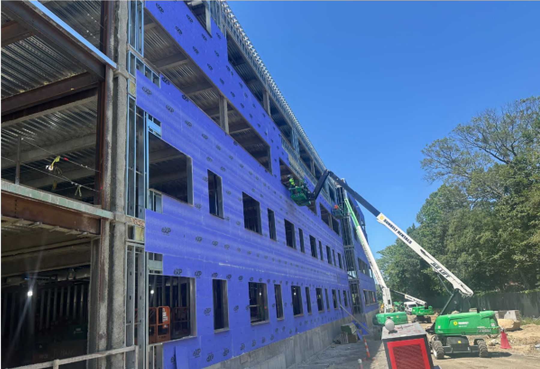
Exterior Sheathing at NHS 6/24/25
