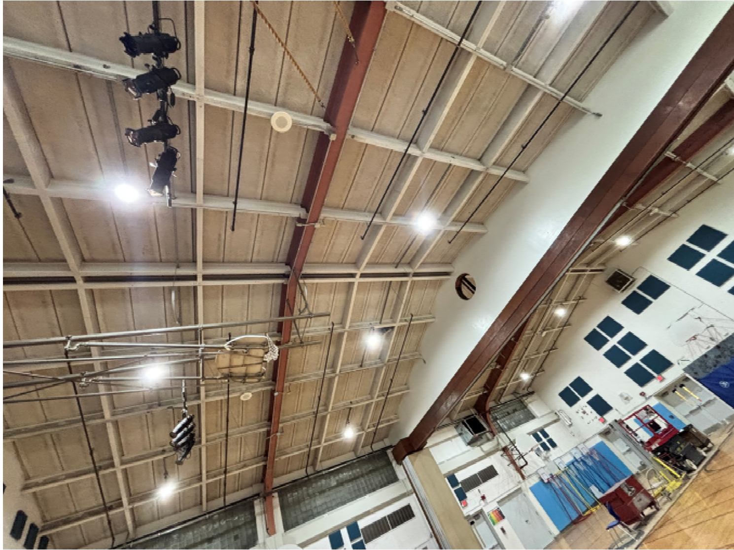
Brookside - Gym Ceiling with all existing ductwork removed – 06/25/25
