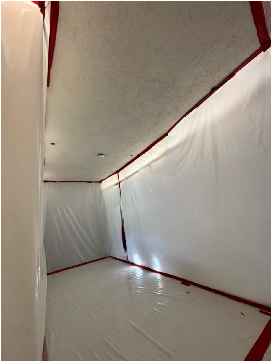
Rowayton – Containment in Classroom – 7/23/25
