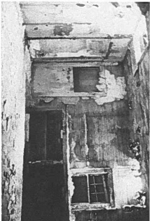
ABOVE: Gardener's Cottage prior to renovation
