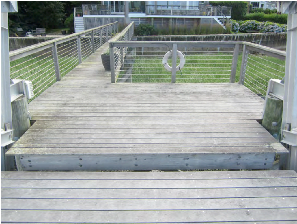
3. VIEW LOOKING LANDWARD FROM WATERWARD TERMINUS OF UNAUTHORIZED PLATFORM ATOP BOAT LIFT. NOTE UNAUTHORIZED EXTENSION OF PIERHEAD BETWEEN BOAT LIFT PILINGS.
