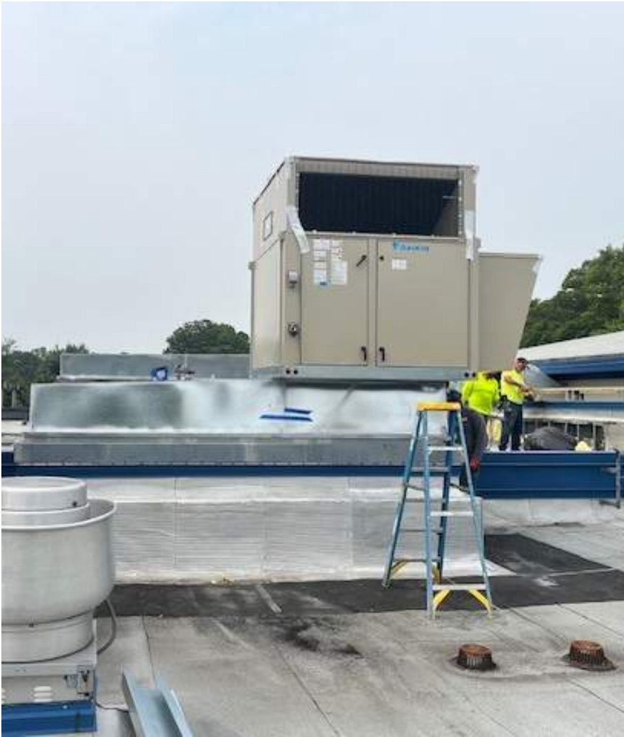
Brookside – RTU Installment – 08/05/25
