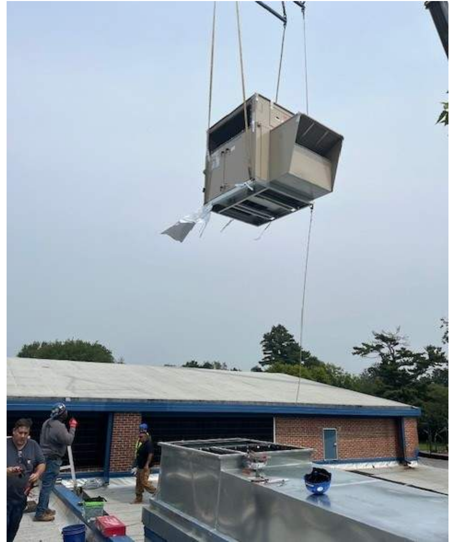
Brookside – RTU Installment – 08/05/25
