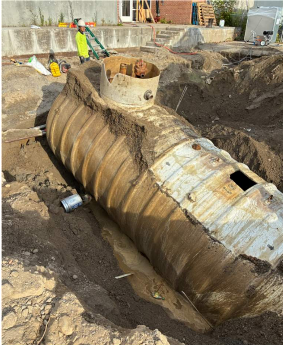
Brien McMahon High School – UST Removal – 8/16/25
