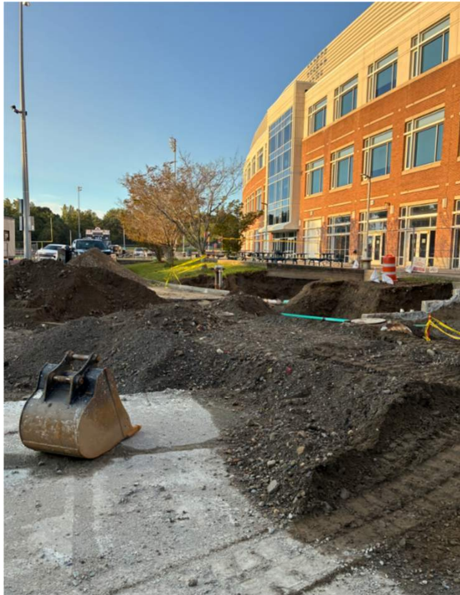
Brien McMahon High School – Chiller Pad and Underground Conduit Excavation – 9/9/25
