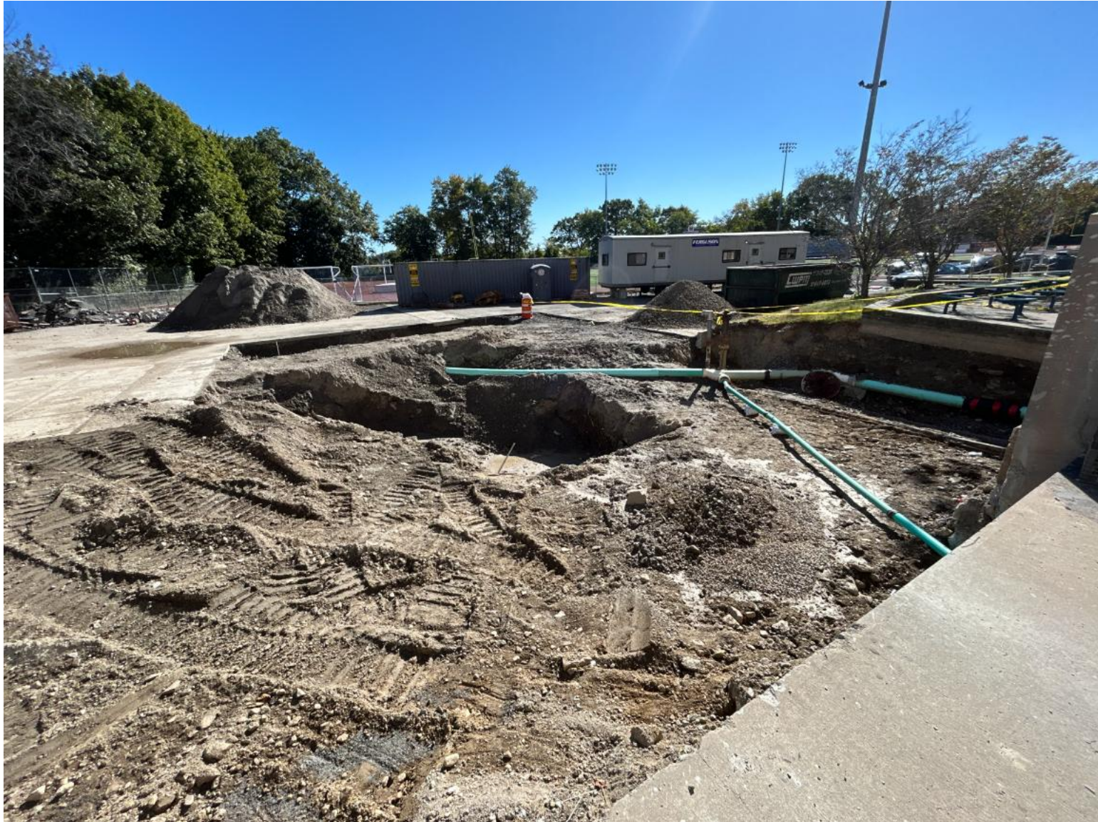
Brien McMahon High School – Drainage Lines – 10/9/25
