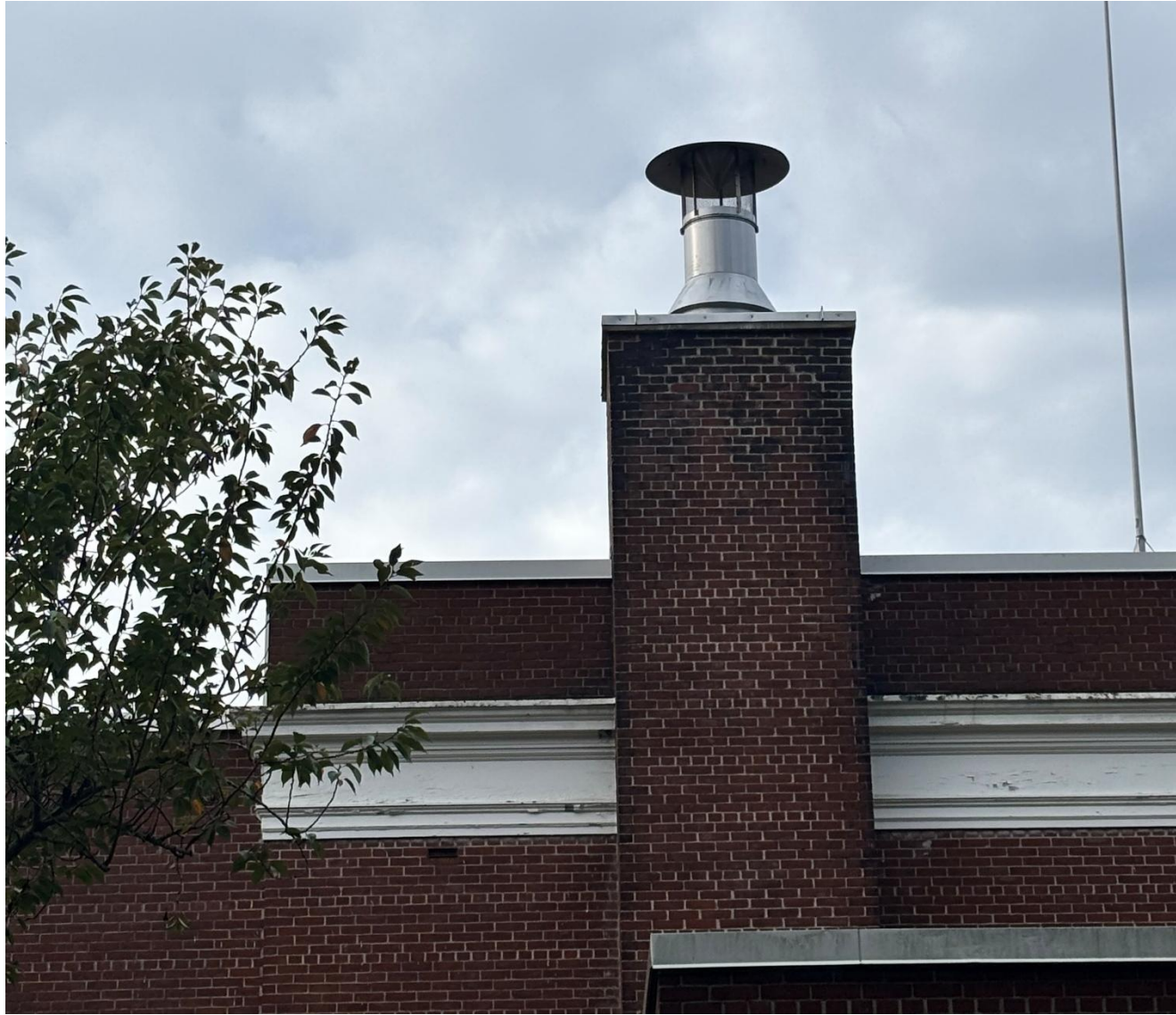
Rowayton – Repointed Chimney – 10/16/25
