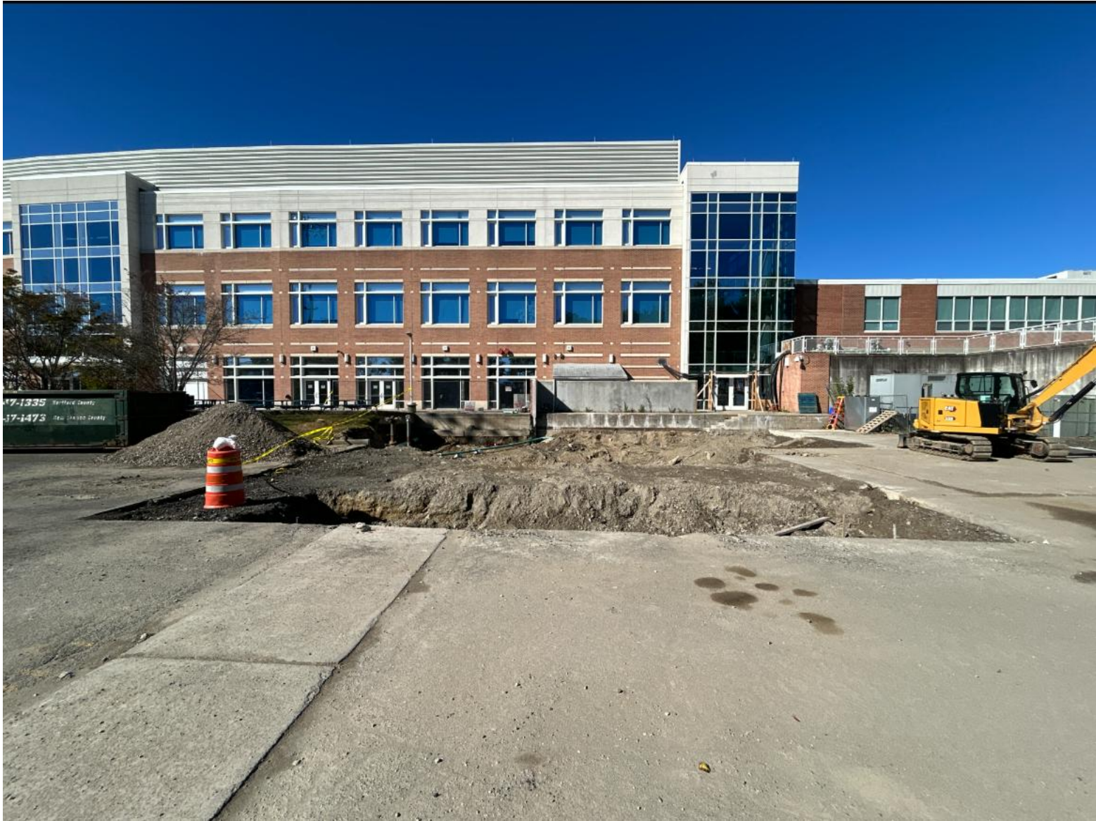
Brien McMahon High School – Loading Dock Area – 10/9/25
