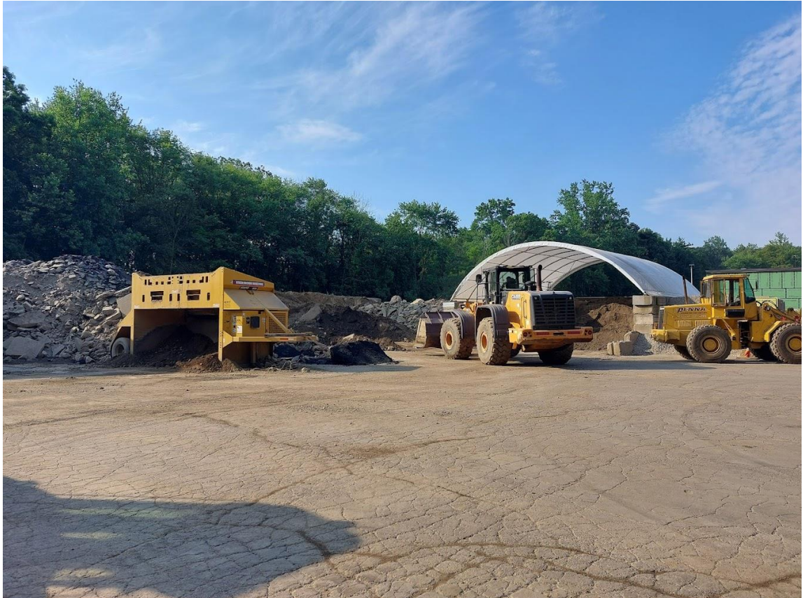
Photo: AJ Penna & Son Construction Yard with Sifter (left) and Loaders
