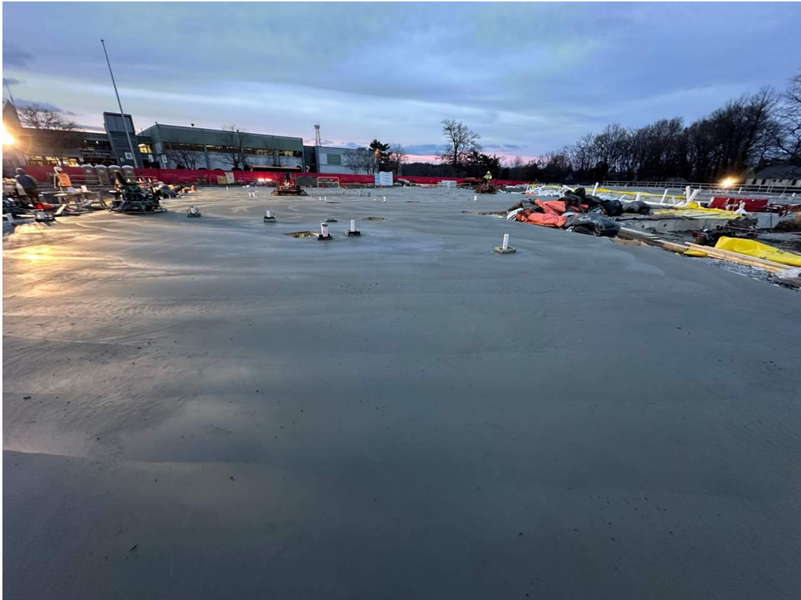
Concrete Slab on Grade 12/19/24
