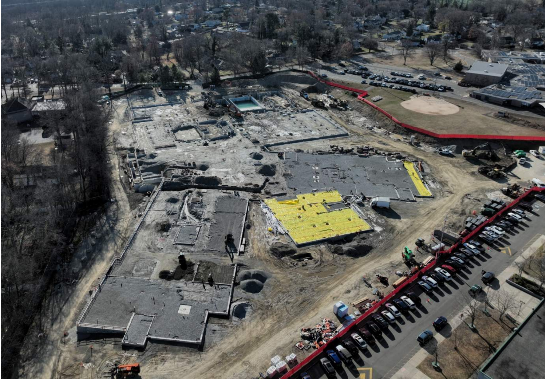
Drone Image – Foundations, Underslab Utilities, Pool Concrete 10/31/24
