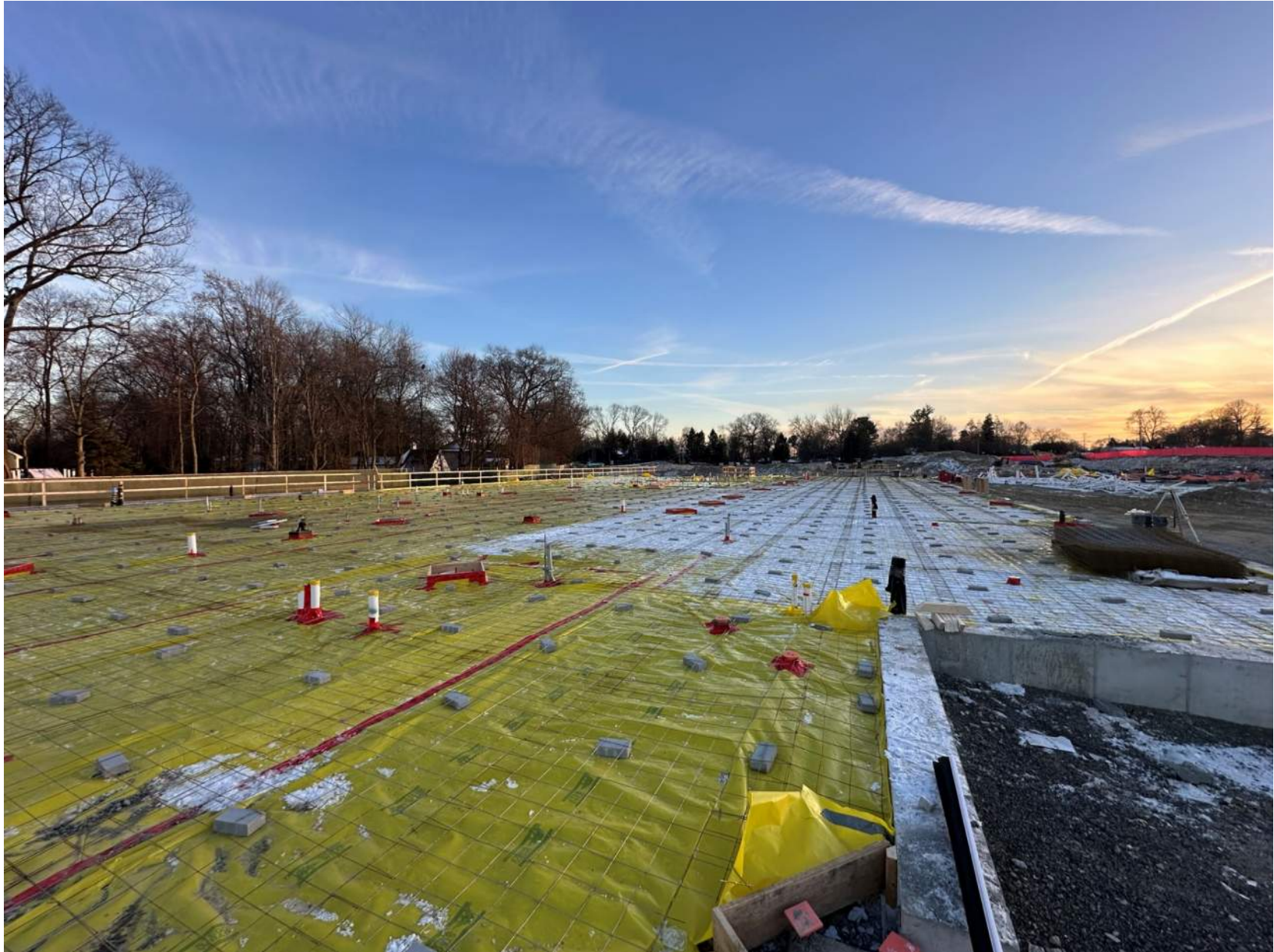
Slab on Grade Prep 12/23/24
