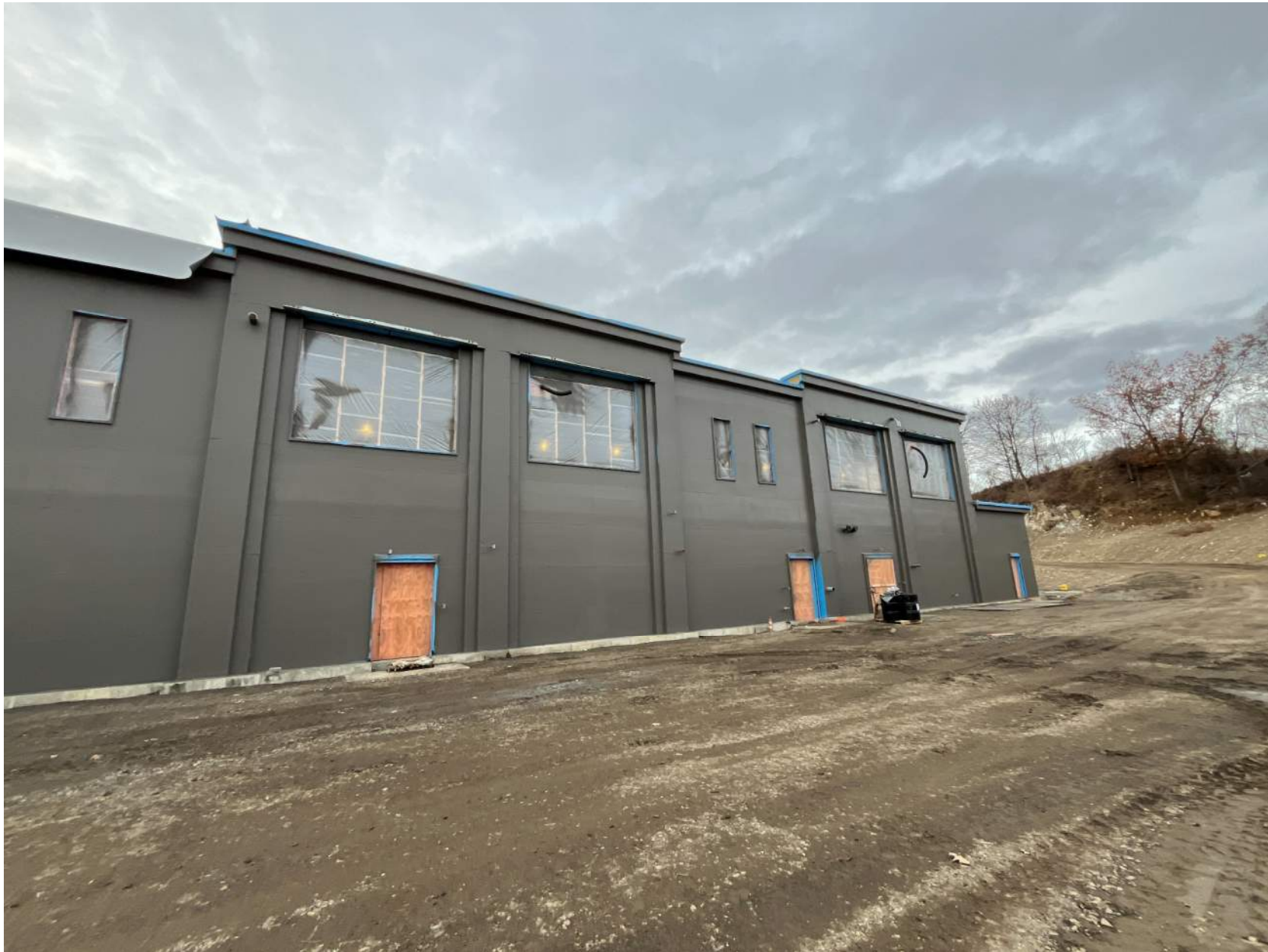
Building Envelope at Service Area 12/19/24
