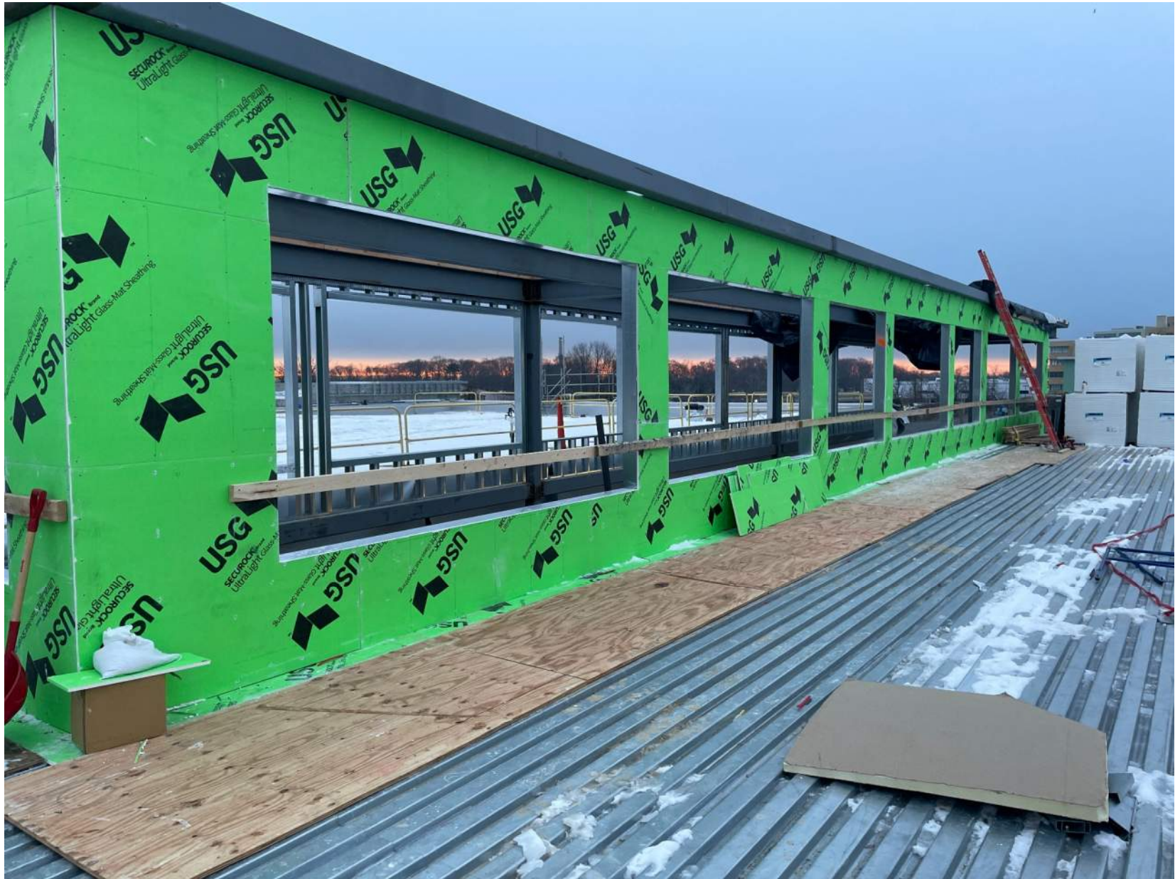
Building Envelope at Roof 12/24/24
