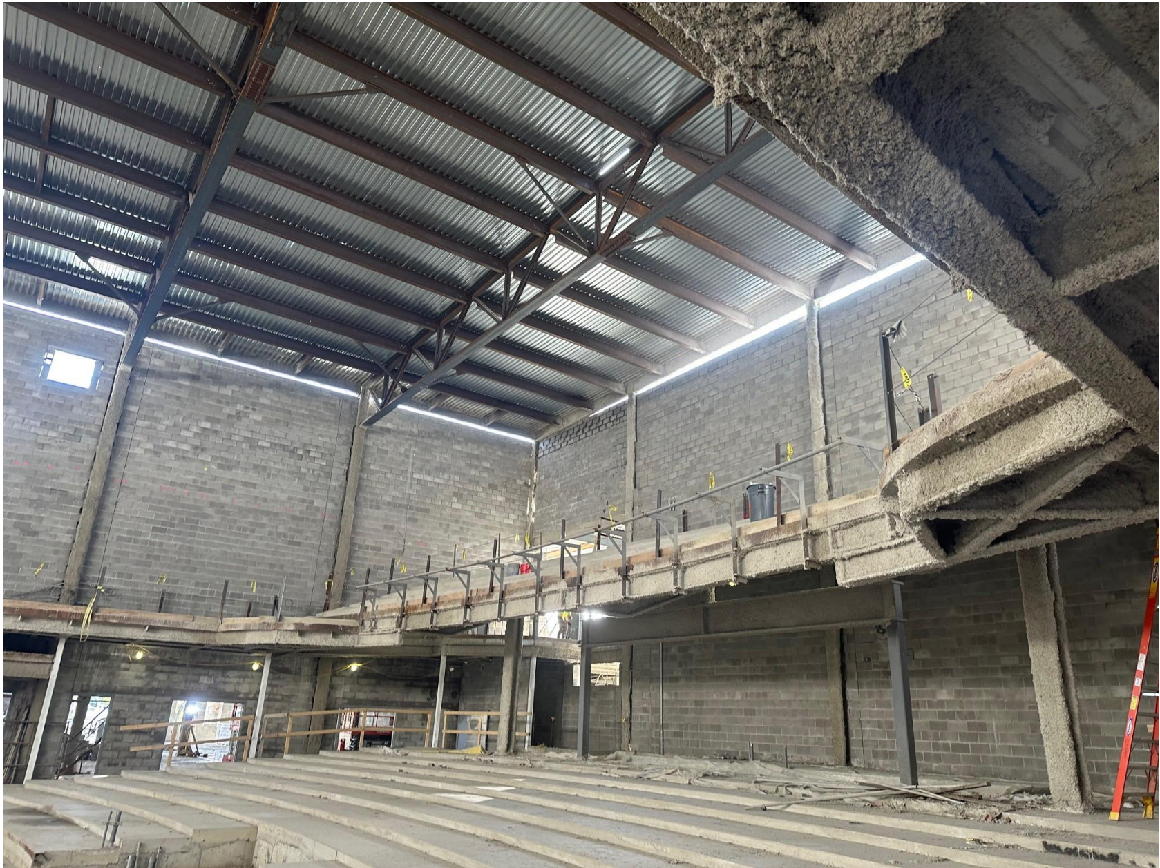
Building Structure Interior – Auditorium 11/17/25
