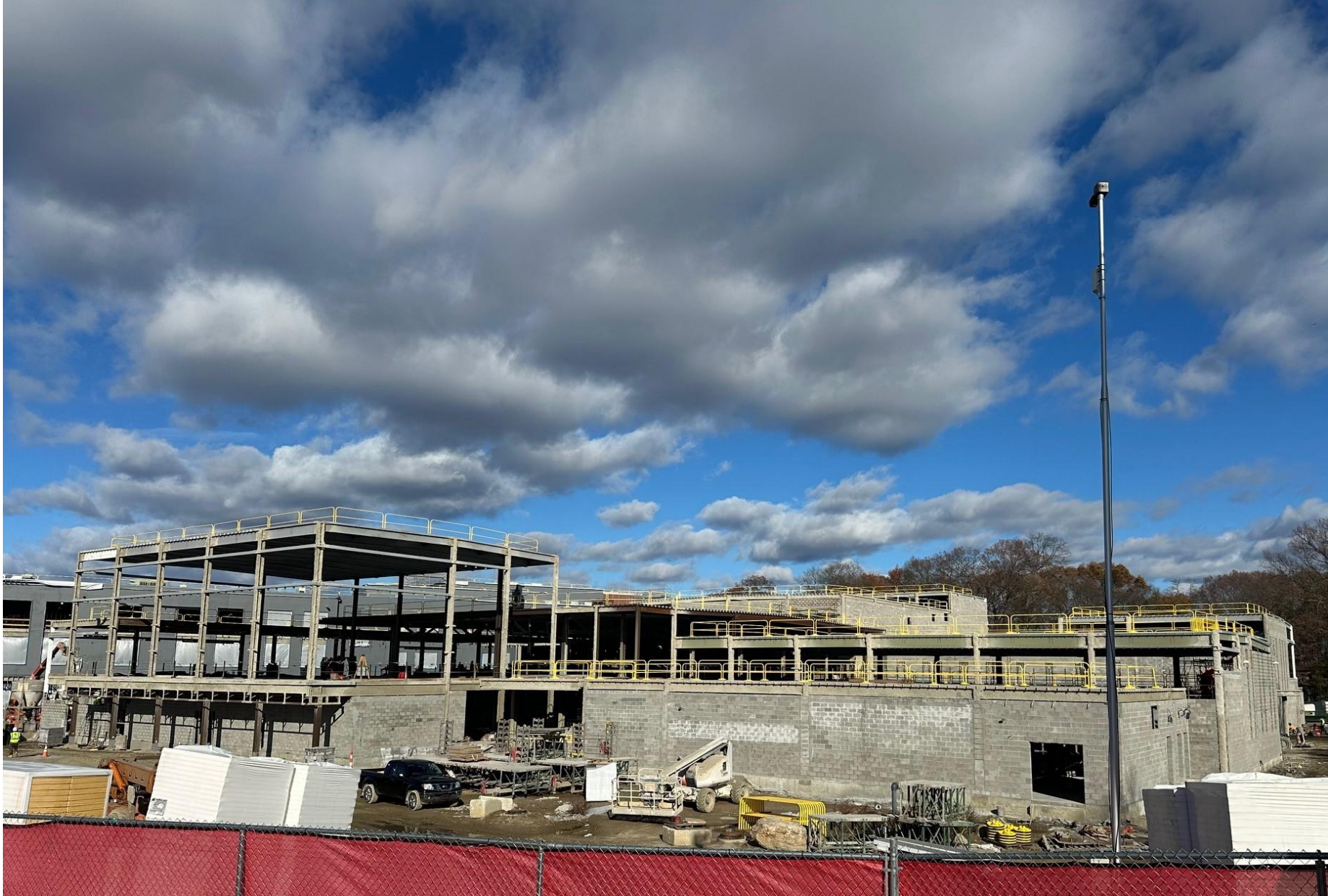
Building Structure – Auxiliary Gym & Pool Area 11/17/25
