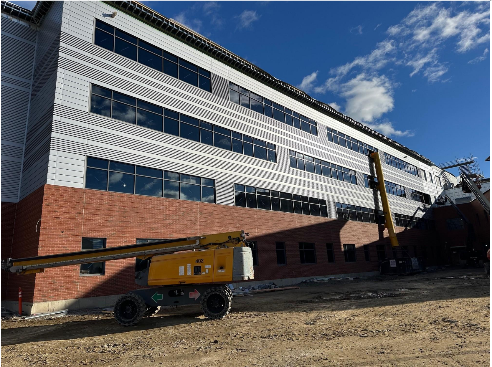
Building Envelope –NHS Wing 11/17/25
