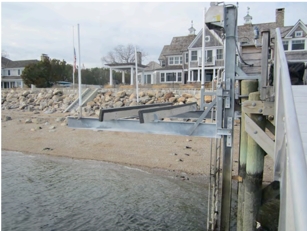
4. VIEW FROM ALUMINUM RAMP LOOKING NORTH TOWARDS BOAT LIFT. NOTE CLEARANCE FROM TOP OF BUNKS TO BOTTOM OF LIFTING ARMS.
