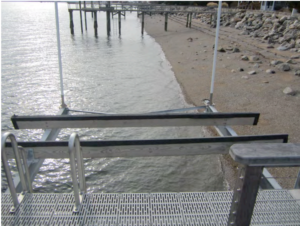
3. VIEW FROM PIER LOOKING TOWARDS BOAT LIFT. NOTE ACCESS PLATFORM WITH OPEN-GRID DECKING IN FOREGROUND.
