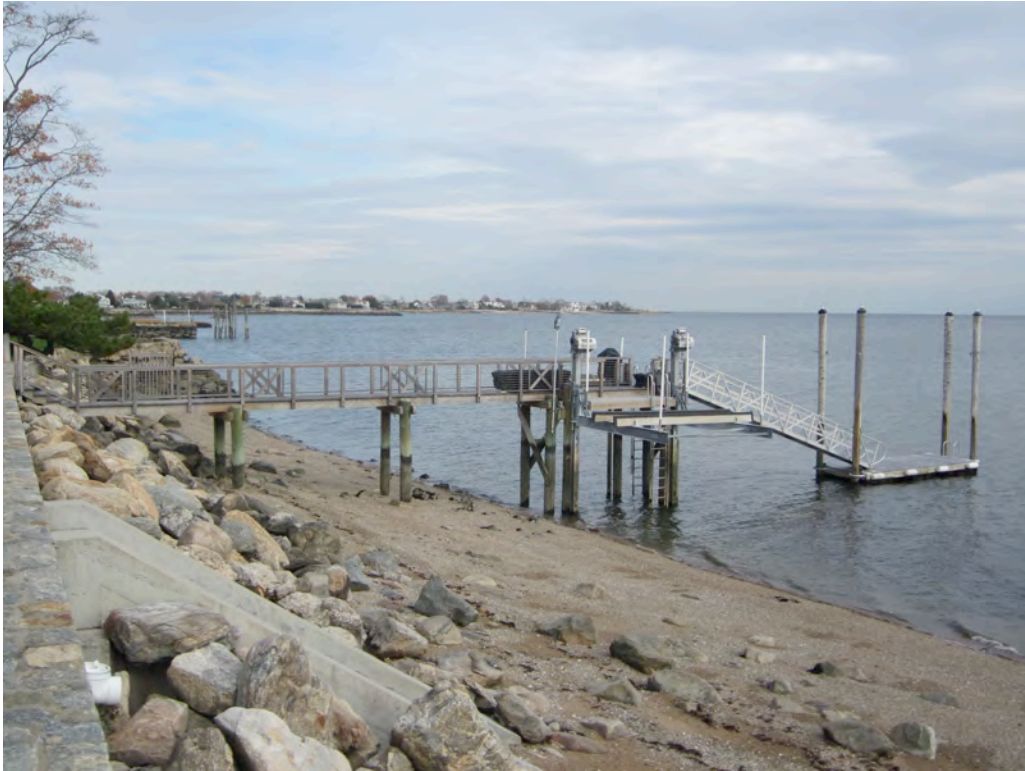
1. VIEW FROM WESTERN PROPERTY BOUNDARY LOOKING TOWARDS BOAT ELEVATOR TO BE REPLACED. NOTE EXISTING REVETMENT, PIER, RAMP, AND FLOATING DOCK.
