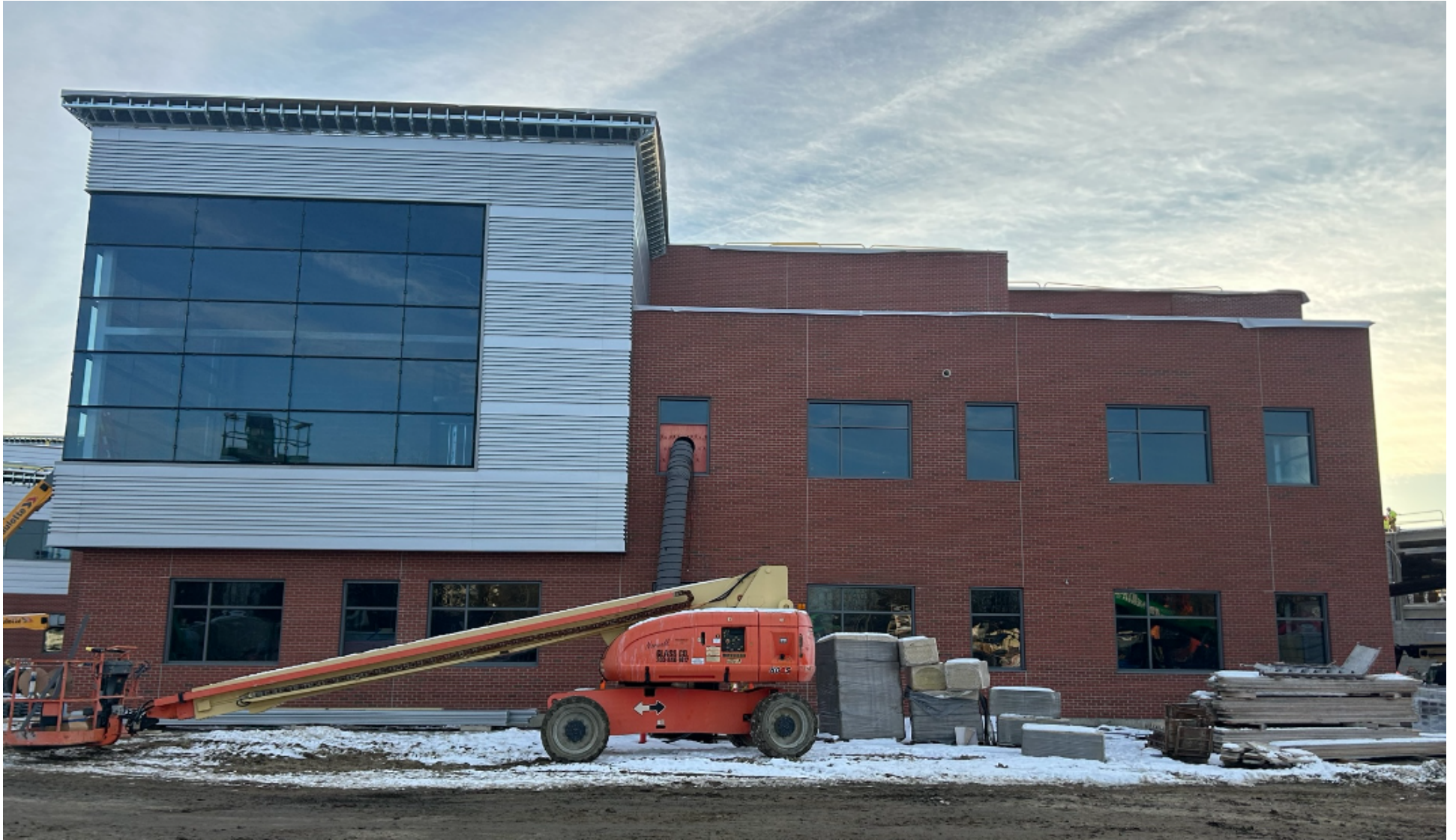
Building Envelope – P-TECH Wing with Project Room 1/27/26
