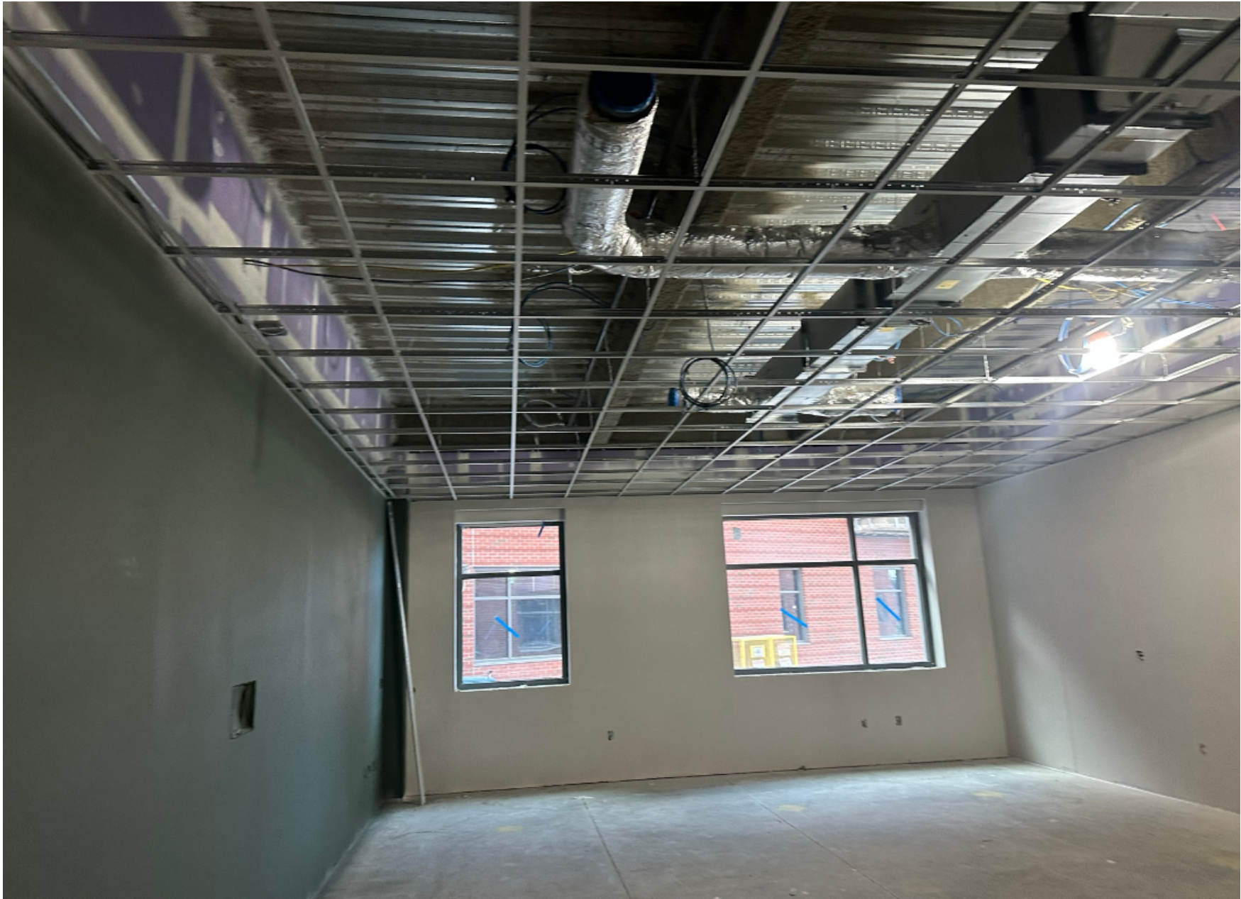
Classroom Finishes Progress 1/23/25
