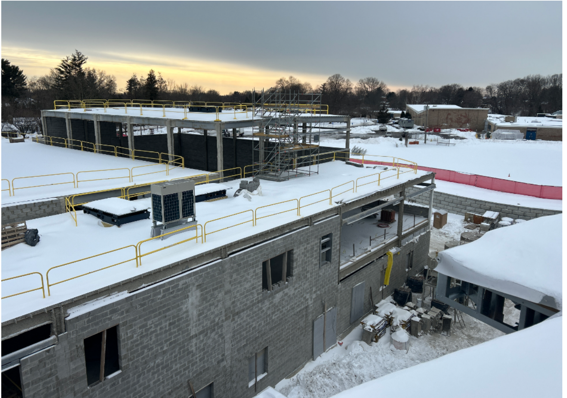
Building Envelope – Auxiliary Gym / Modular Retaining Wall 1/27/26
