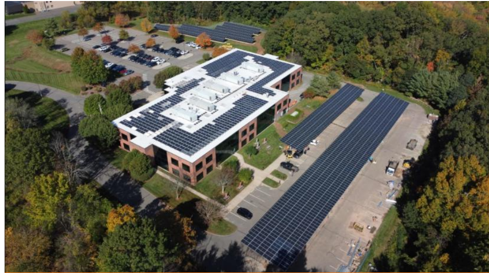
Lane Construction: 666 kW DC
