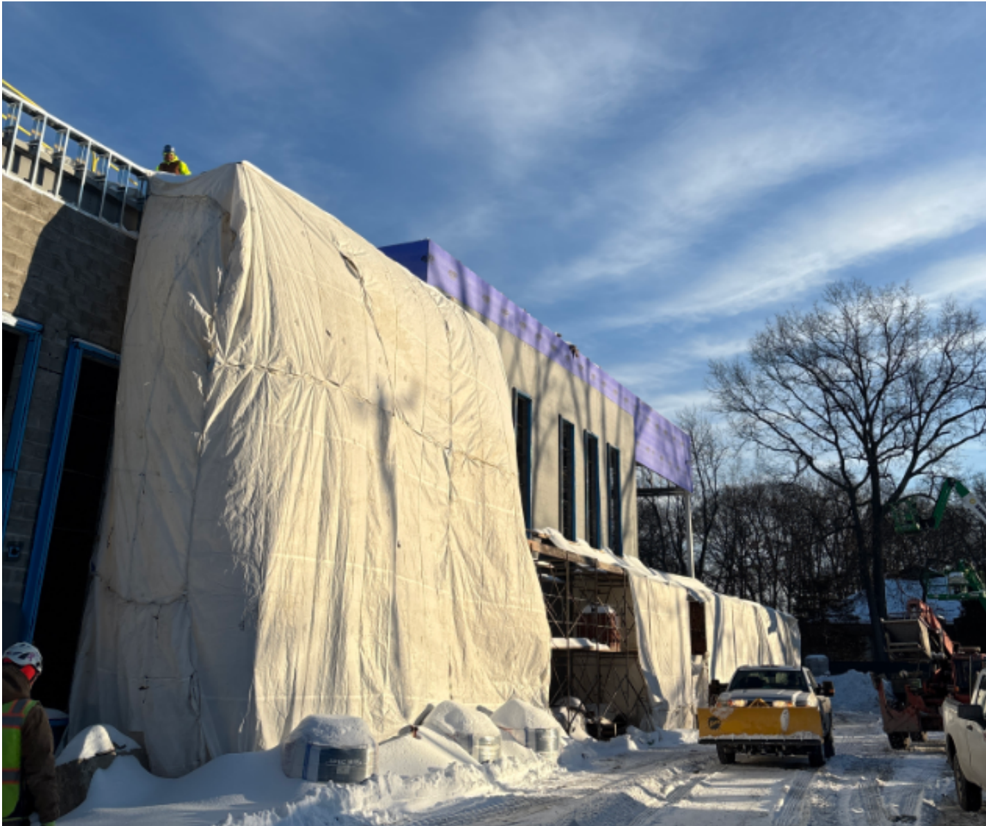
Building Envelope – Performing Arts (Band) Space 1/27/26
