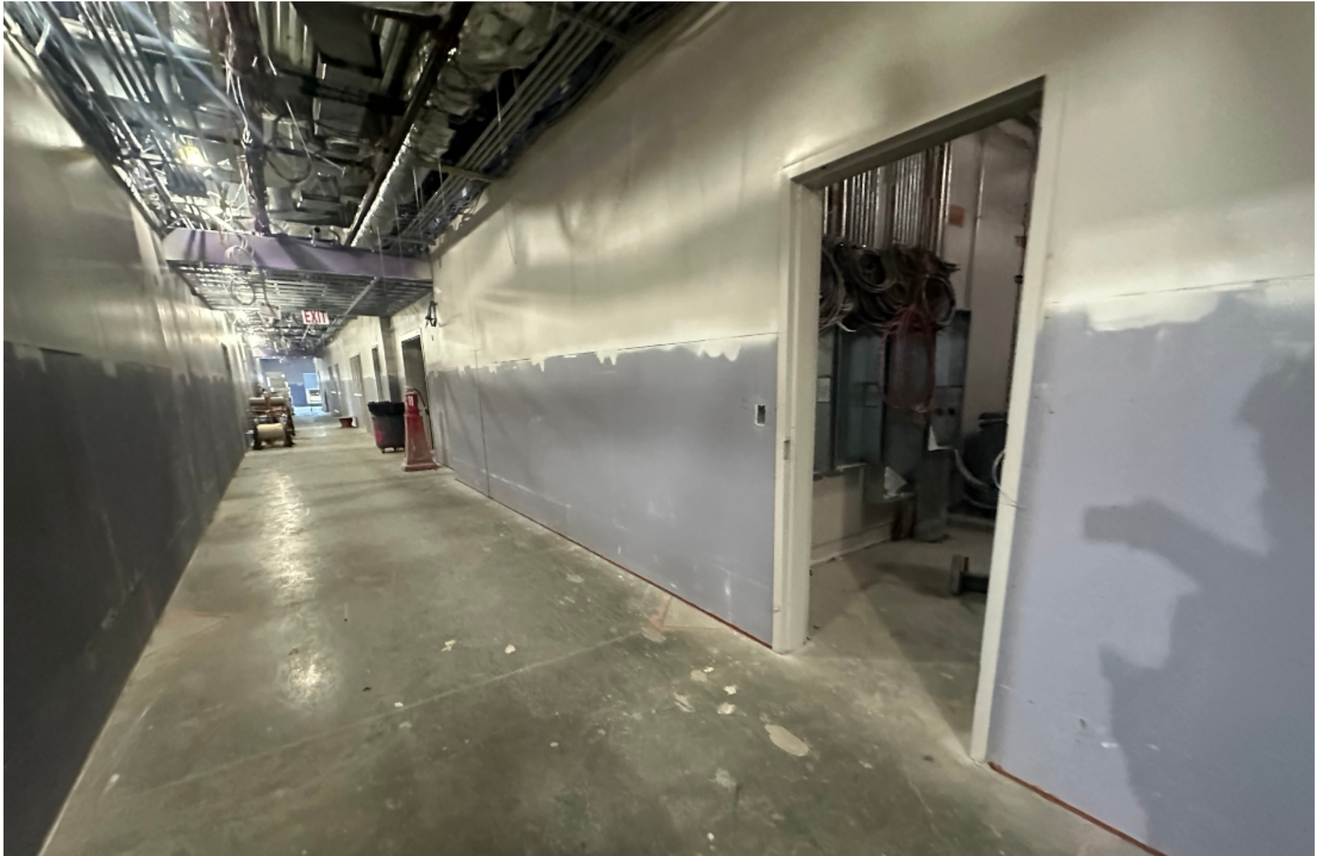
Corridor Finishes Progress 1/23/25
