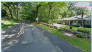
Grumman Avenue Sidewalk Extension
