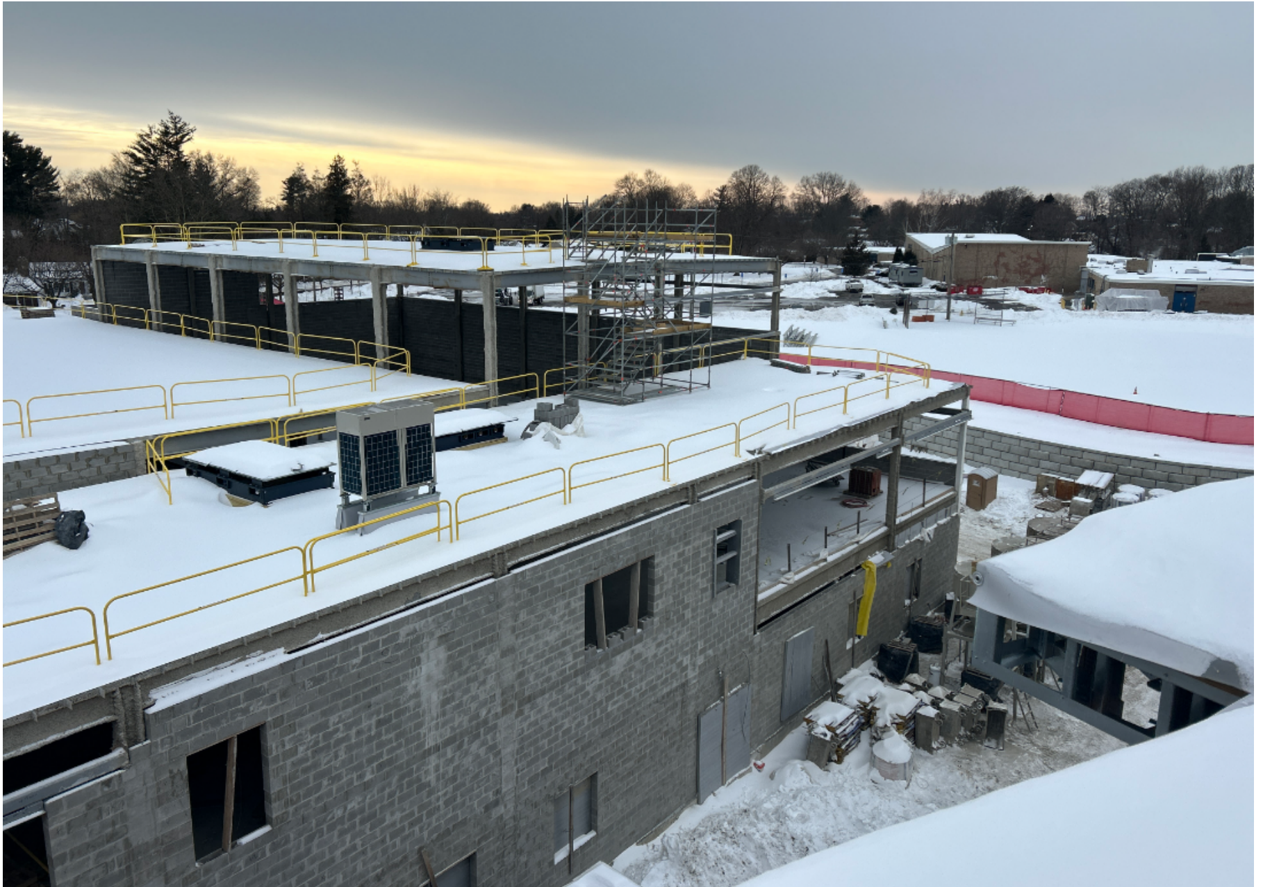
Building Envelope – Auxiliary Gym / Modular Retaining Wall 1/27/26
