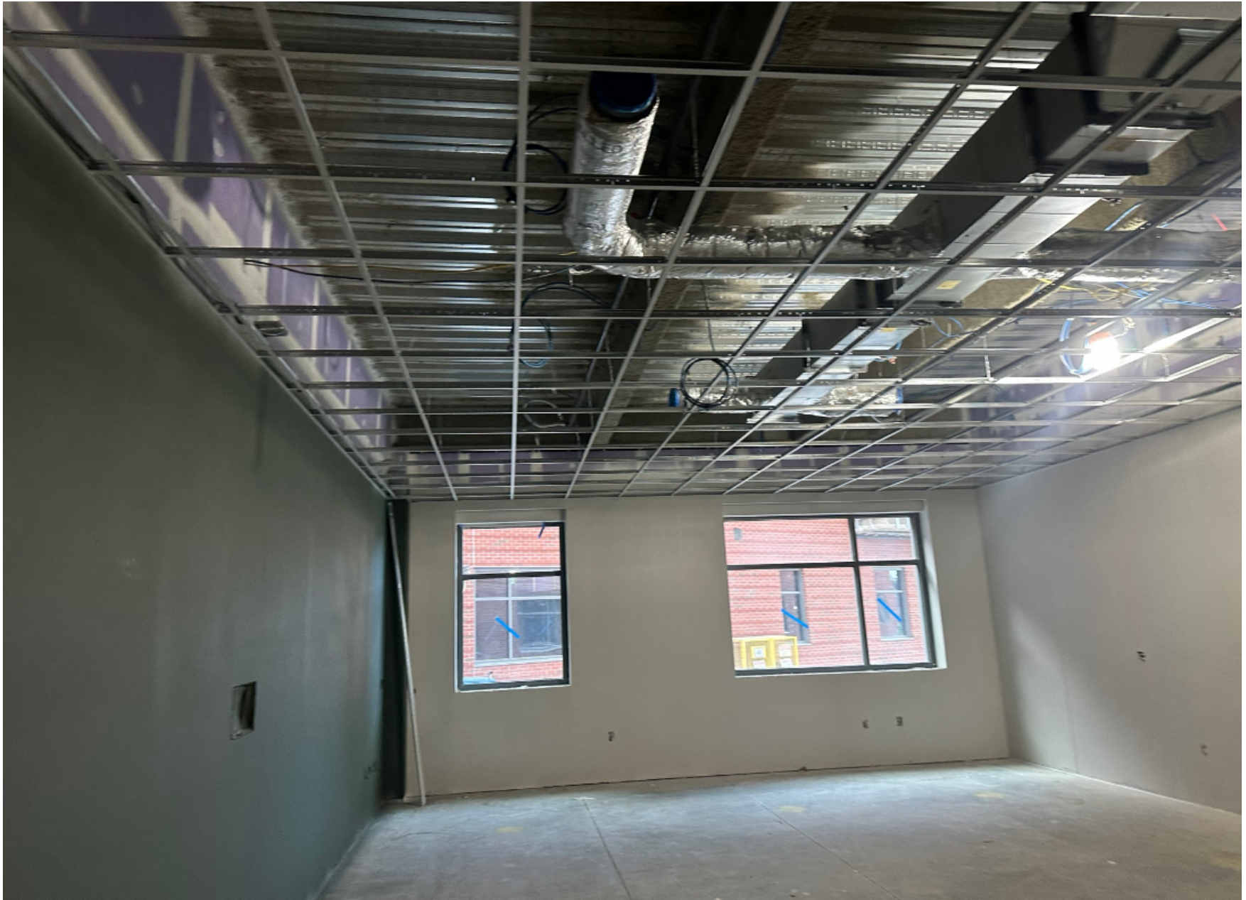
Classroom Finishes Progress 1/23/25
