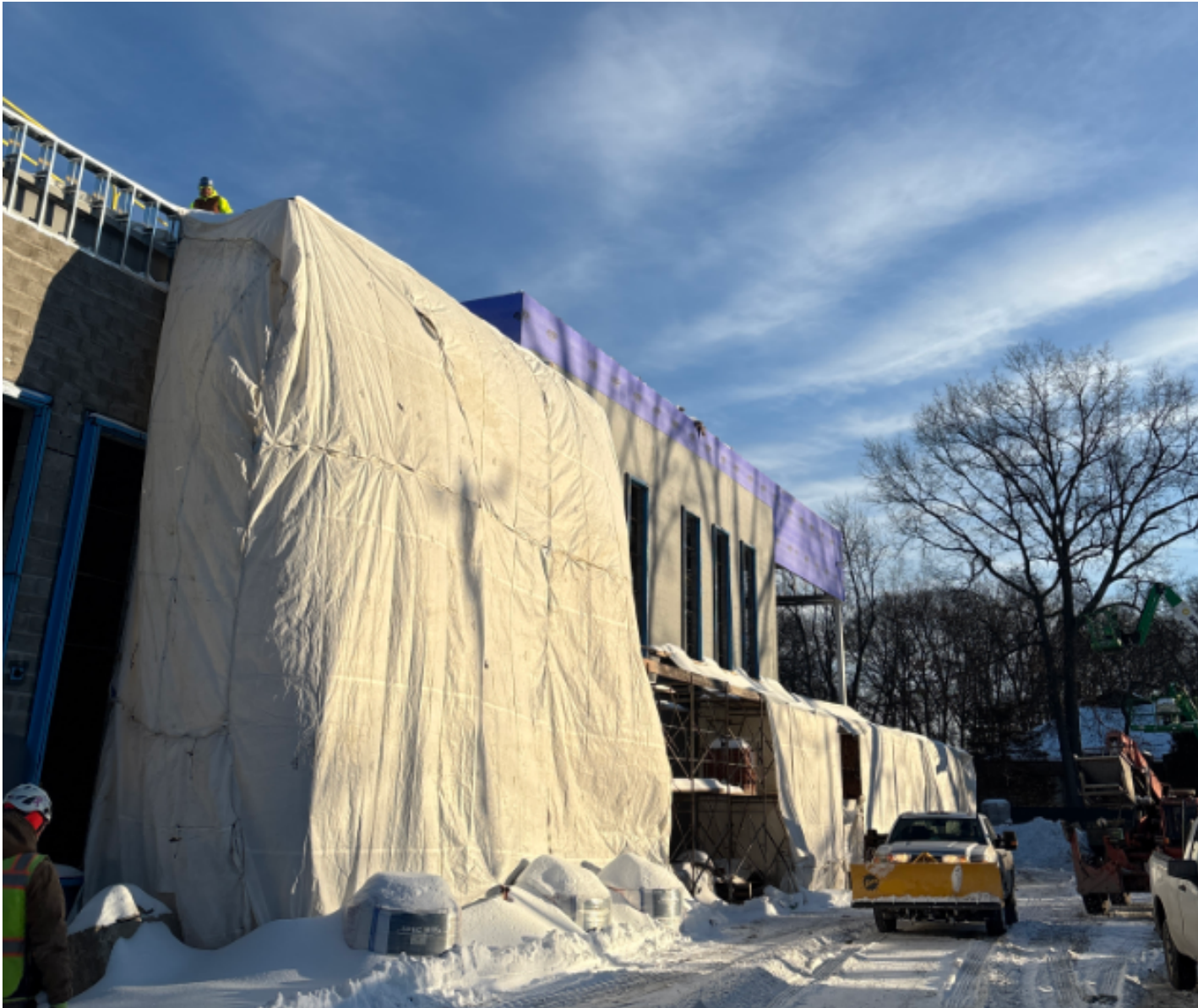
Building Envelope – Performing Arts (Band) Space 1/27/26
