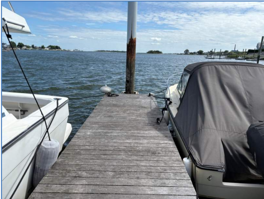
Figure 8 – Existing T-Head and Float Anchor Pile, View Facing South
