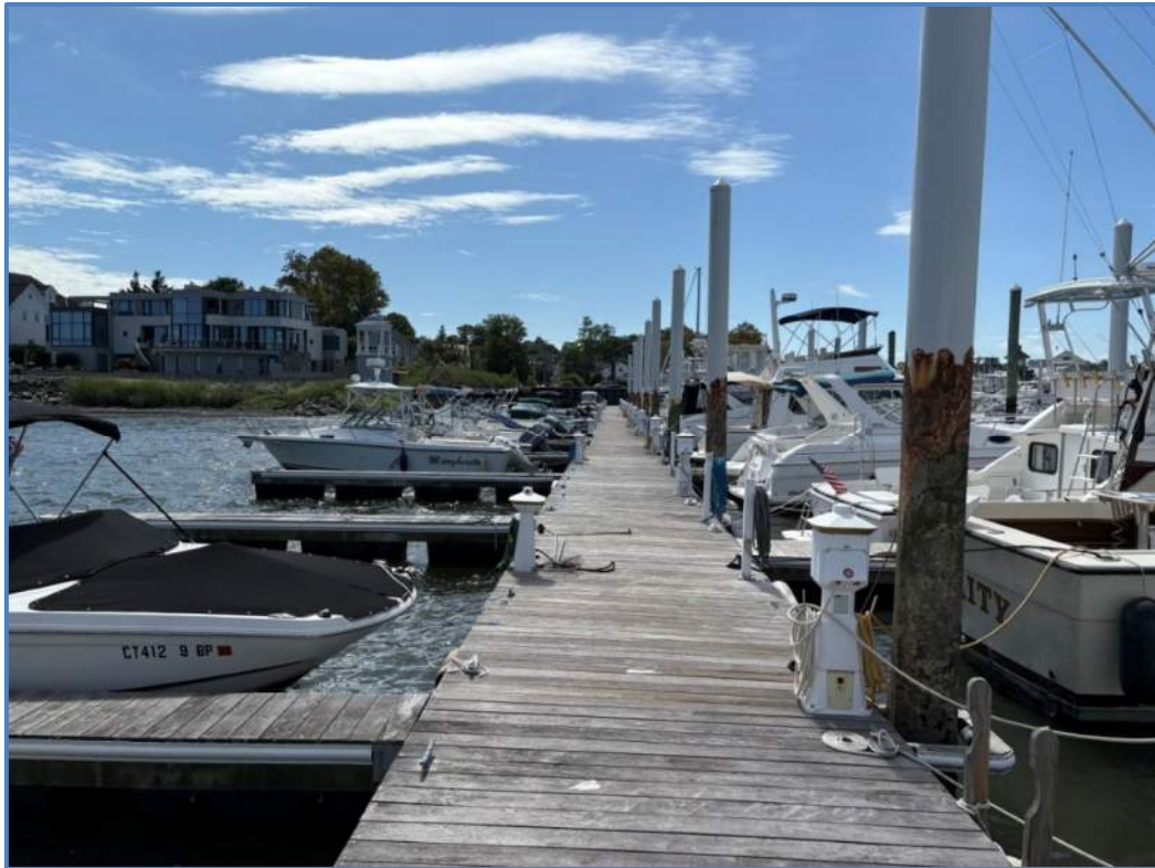
Figure 10 – South Dock Tree, View Facing West
