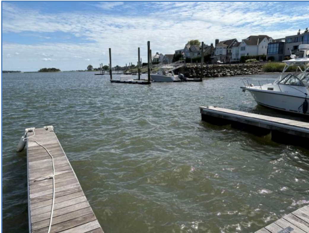
Figure 6 – Neighboring Property Dock, View Facing Southwest
