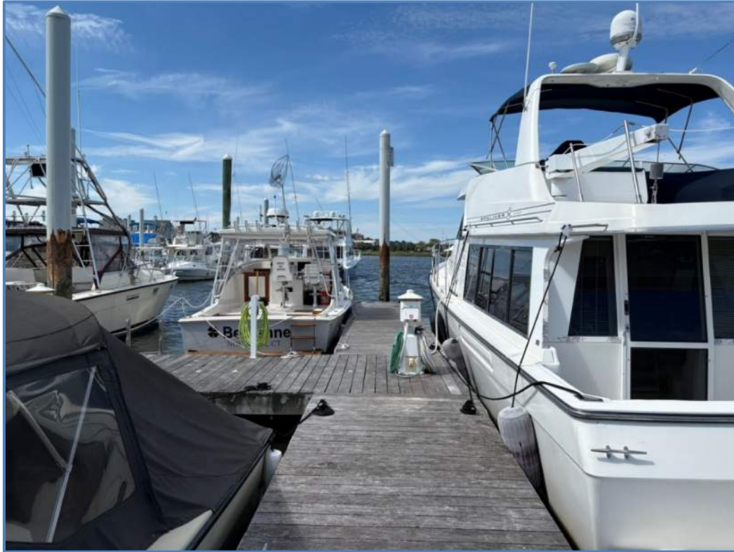
Figure 9 – Existing T-Head, View Facing North
