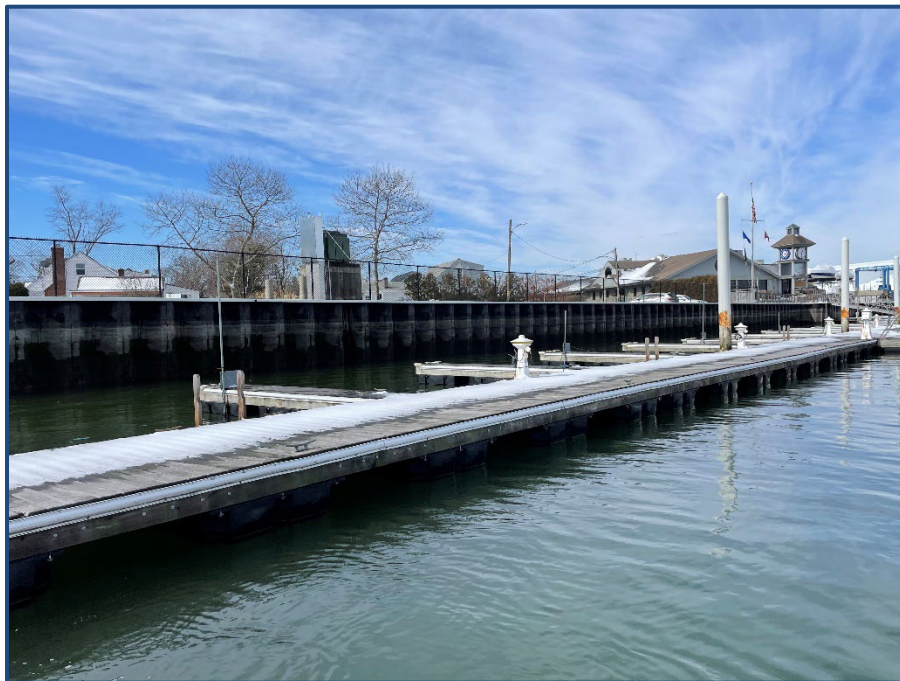
Figure 4: Photograph of bulkhead in dredge area
