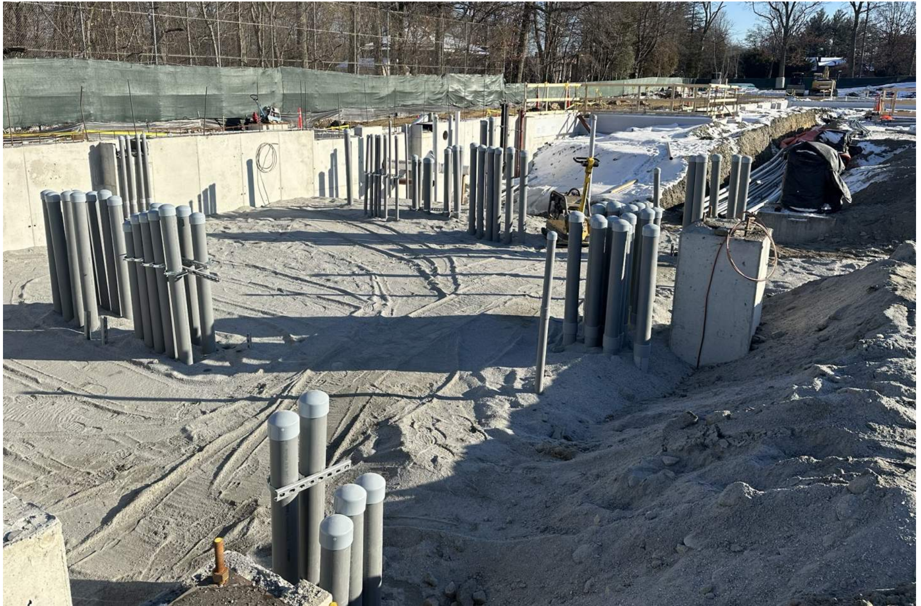
Underslab Utilities at Electrical & Emergency Electrical Room 1/24/25
