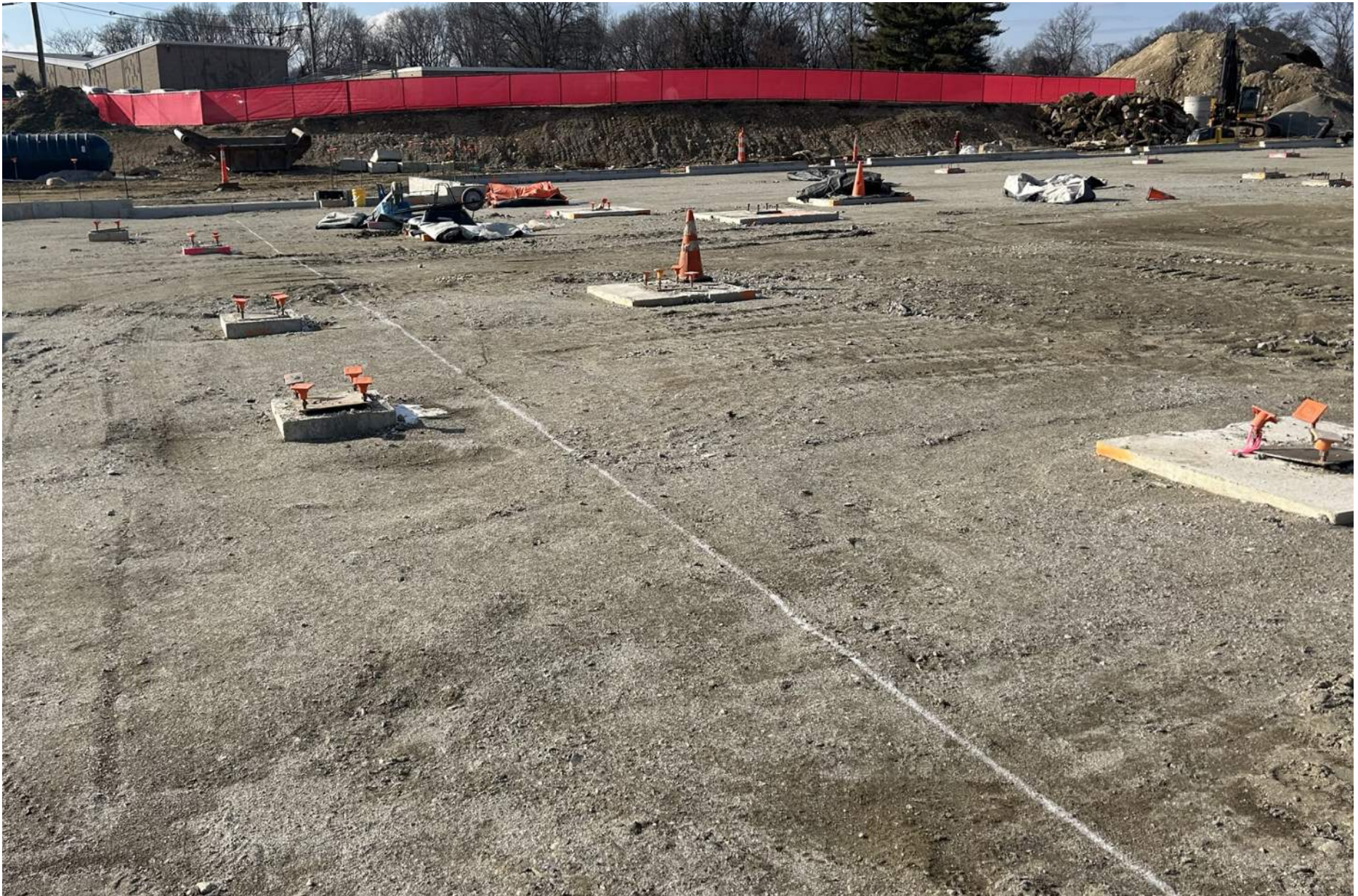
Slab on Grade Prep 12/23/24
