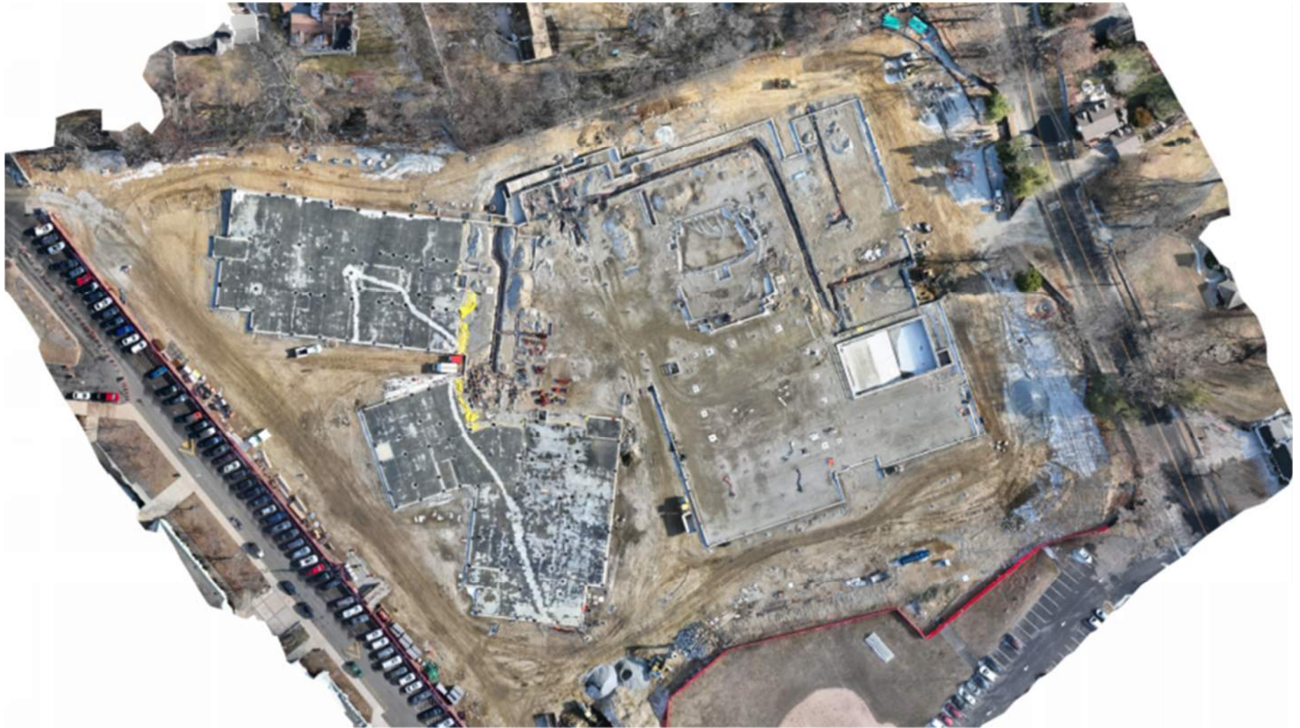
Drone Image – Foundations, Slab on Grade, Underslab Utilities, Pool Concrete 1/17/25
