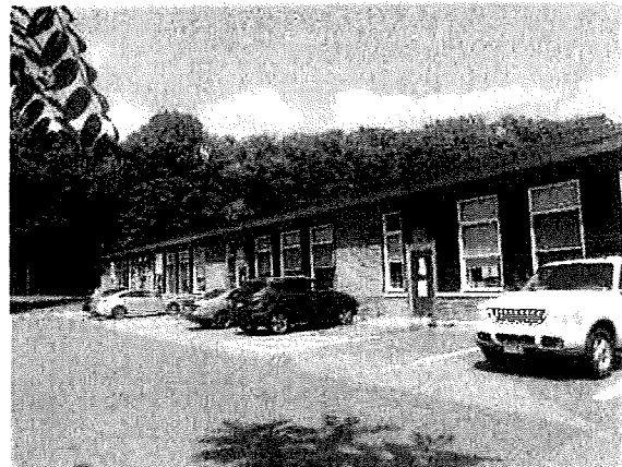
West facing view of existing classrooms
