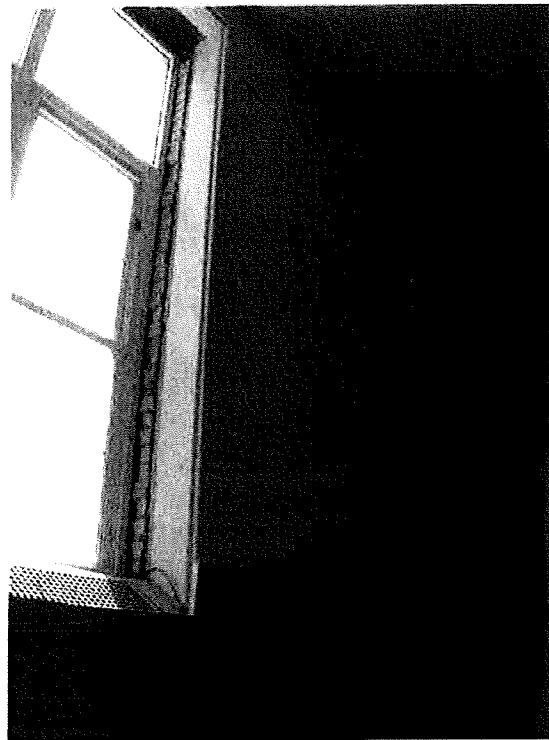
Existing Window Trim Detail
