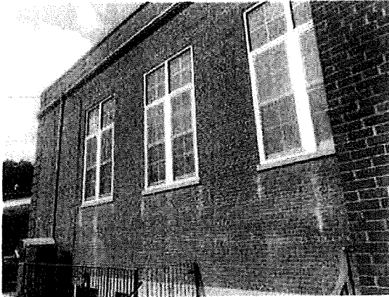
South facing view of existing Gymnasium
