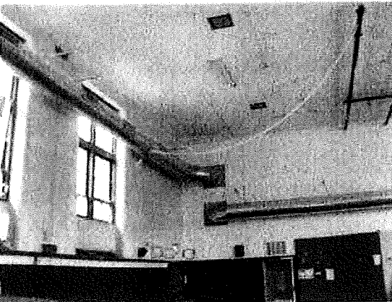
Existing Gymnasium Interior Ceiling View
