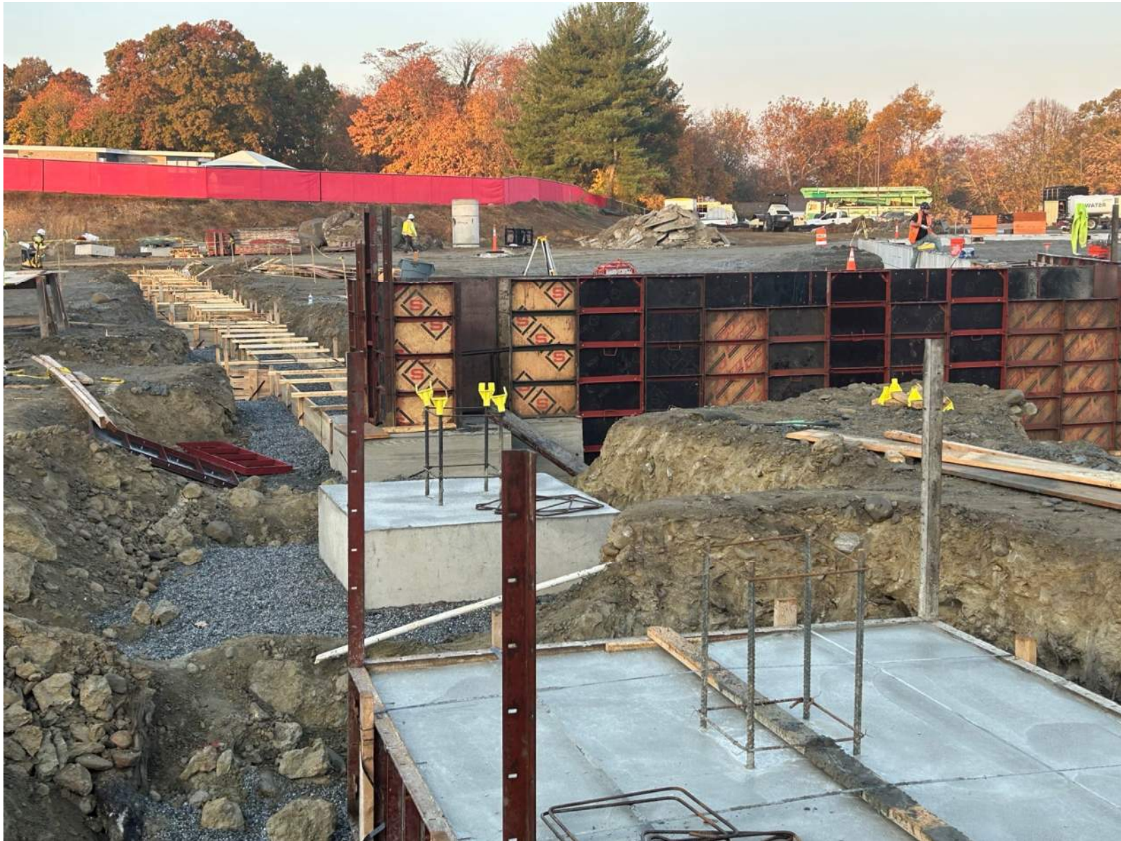
Interior Pier Footings, Exterior Footing Formwork, Exterior Foundation Wall Formwork 10/30/24
