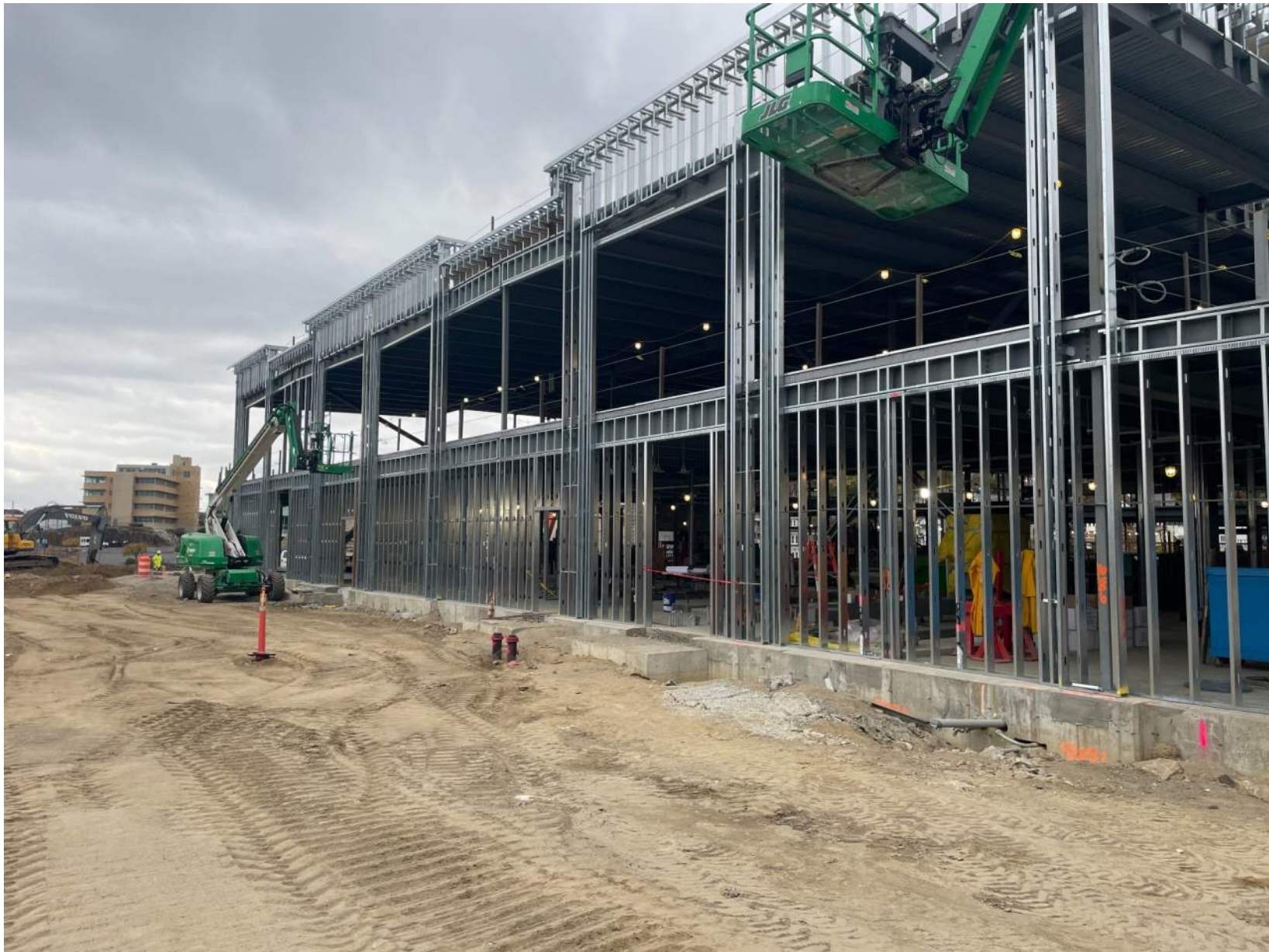
Exterior CFMF at Service Entrance 10/30/24
