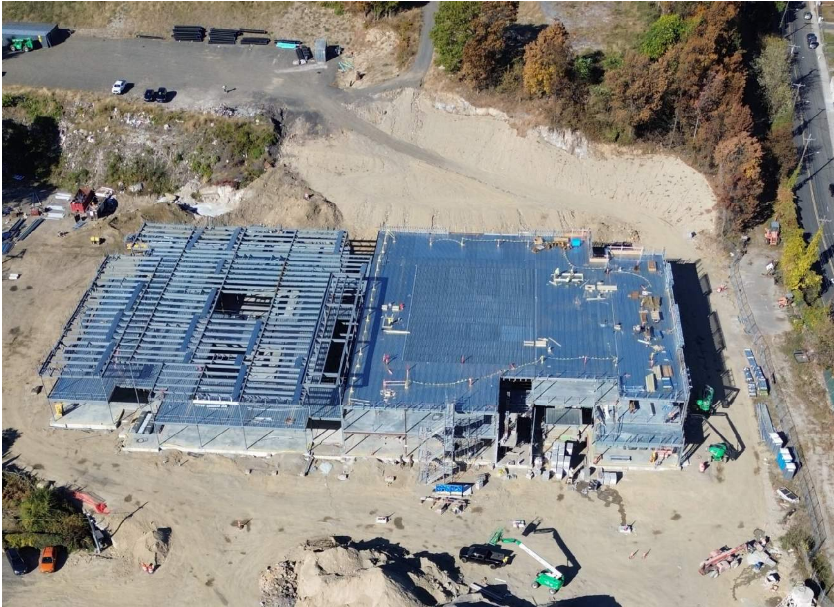
Drone Image – Steel & Metal Decking, Slab on Grade Concrete, 2 nd Floor Concrete 10/25/24
