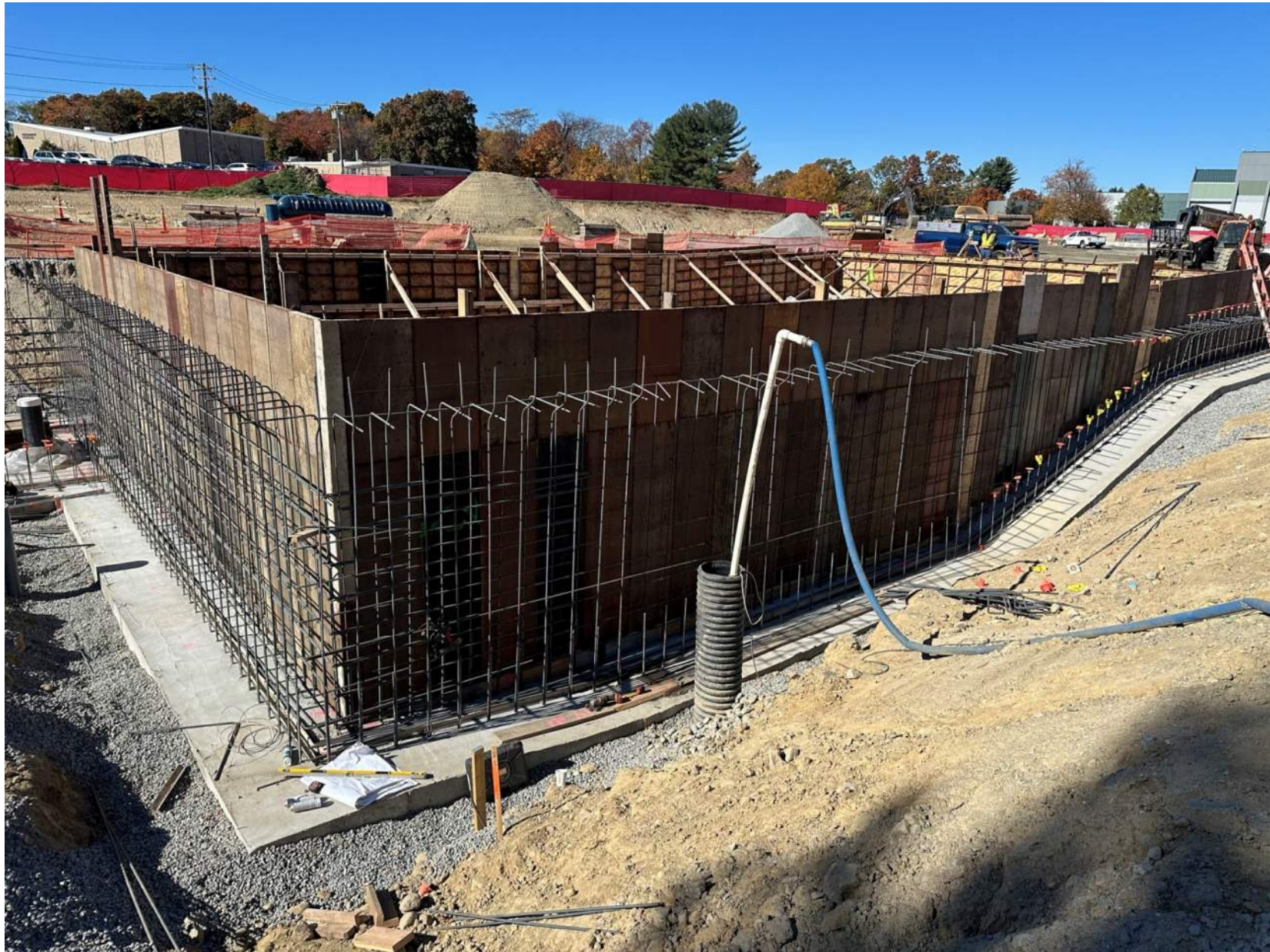
Pool Slab, Wall Reinforcement & Formwork 10/25/24
