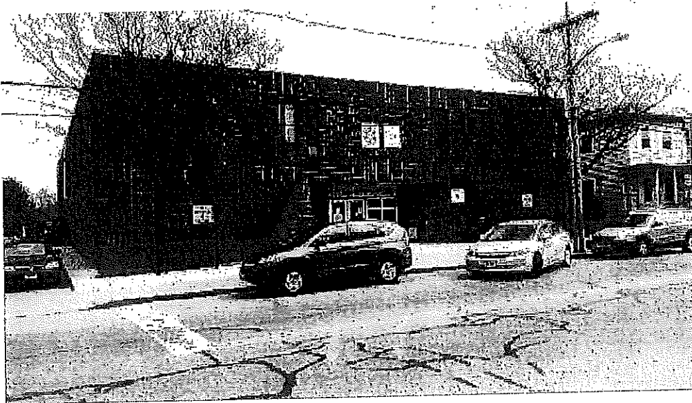
FRONT VIEW OF THE BUILDING
